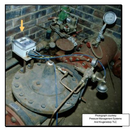
Figure 1.5: Typical installation of a time-modulated PRV controller
