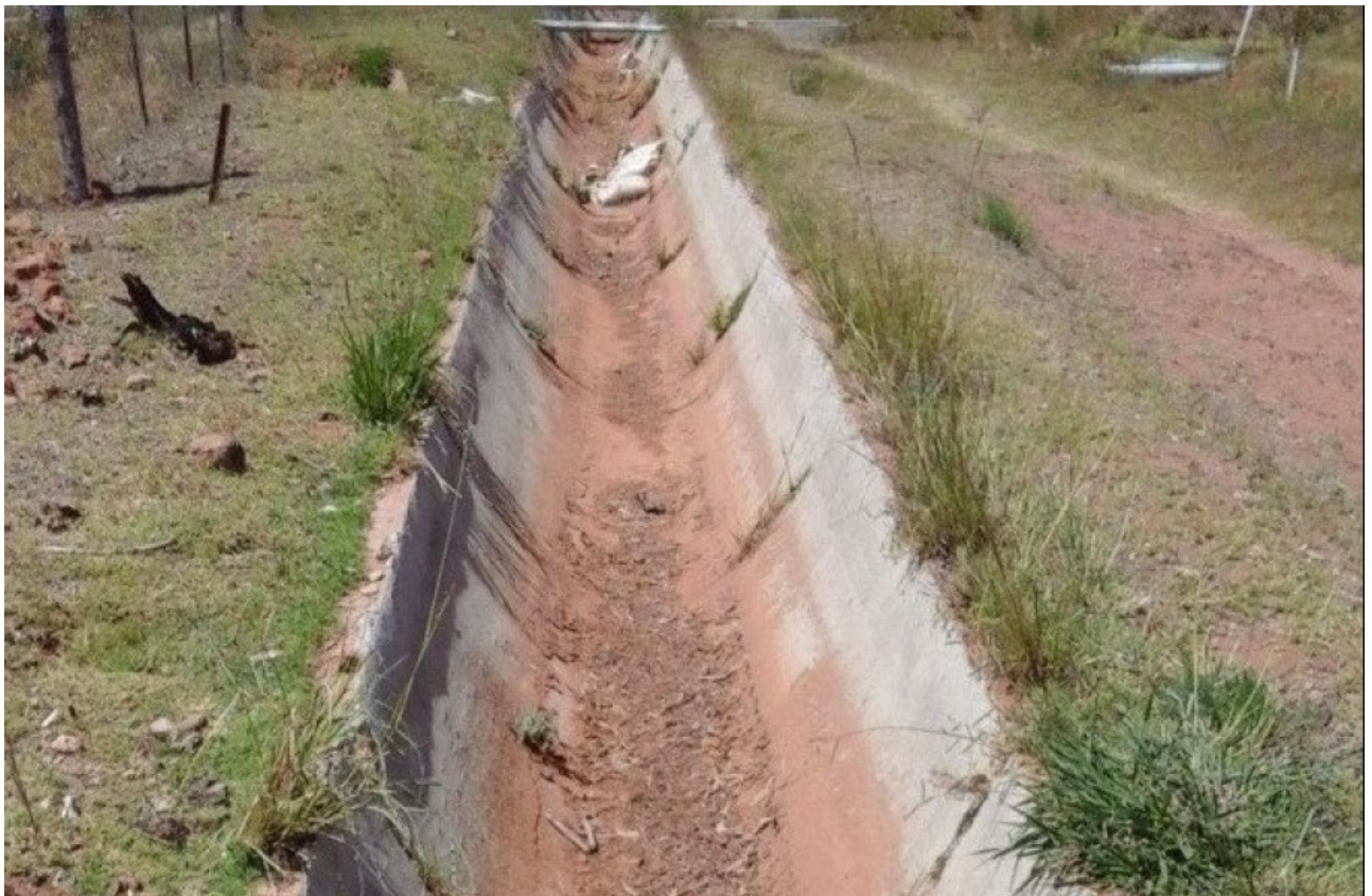
Figure 4.13: Empty canal in Ebenhaeser, West Coast
