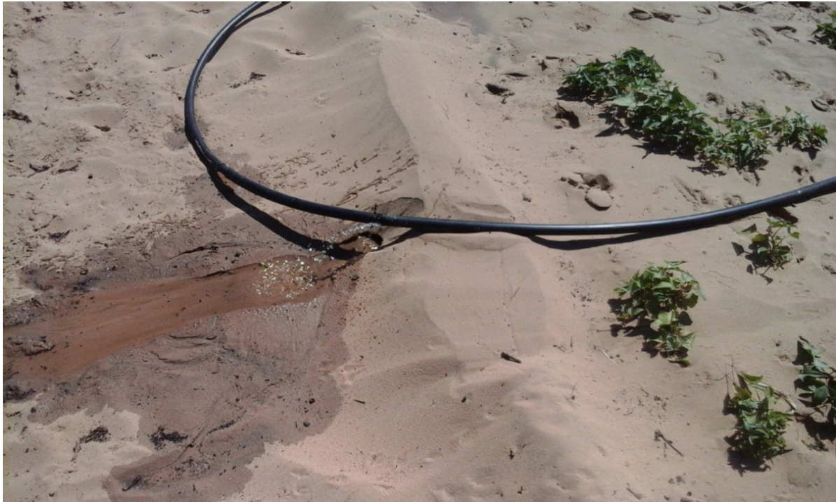
Figure 5.9: A broken pipe leaking while irrigating a vegetable garden in Lamberts Bay
