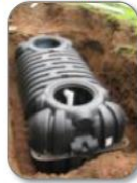
Flush: Septic tank
