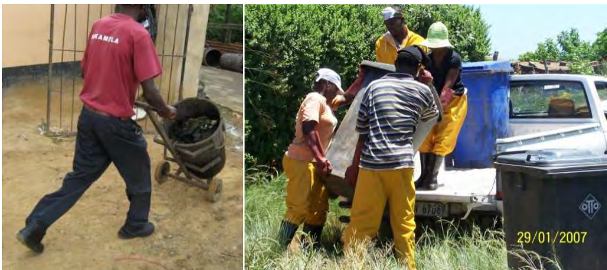
Figure 5.1 eThekweni pit emptiers cart sludge with a drumbarrow to the closest vehicle access point
