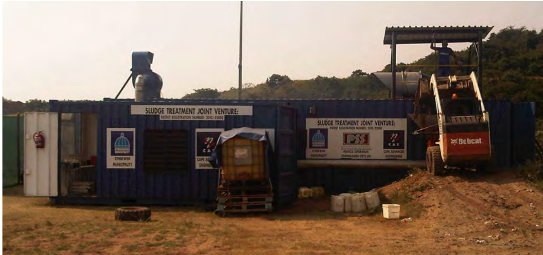
Figure 6.23 eThekweni sludge pelletising plant
