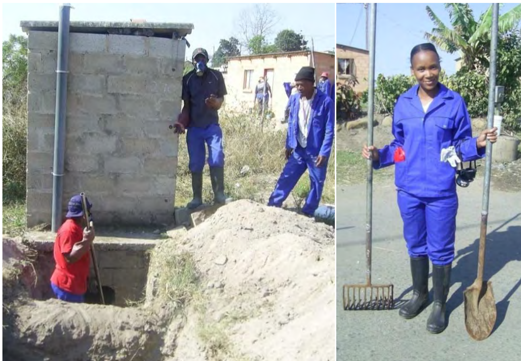
Figure 4.7 eThekweni pit emptiers at work
