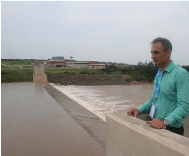
Umgeni Water planning services manager, Kevin Meier, watches millions of litres of water pouring over the R1.6 billion weir which form part of the Lower Thukela Bulk Water Supply Scheme near the mouth of the Thukela River. Water from this scheme is used to supply growing industrial and residential development in the Mandeni and KwaDukuza area, north of Durban.
