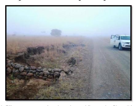
Figure 2-28: Efforts to stop erosion along the road (Located at Photo 7 in Figure 2-3).
