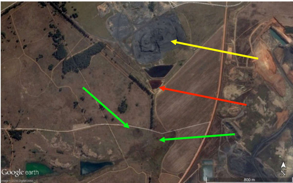
Figure 61 Coal stockpile (yellow arrow) with containment dam (red arrow) that leaks and leads to acid water seeps downslope (green arrows)
