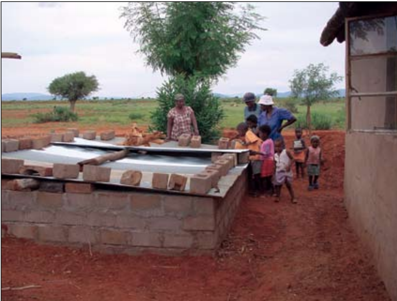
An example of a closed reservoir used to store rainwater for food growing purposes.
