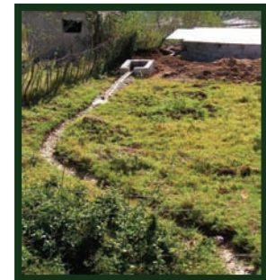
stormwater runoff to 30 000 litre underground collection tank
