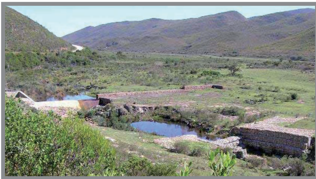
Figure 9: Structures B3 (left) and B1 (right) at Companjesdrift, May 2006. Note the leakage where the concrete abuts the stone gabion on B3. The overflow level on B1 was lowered after the collapse during the 2001 flood.
