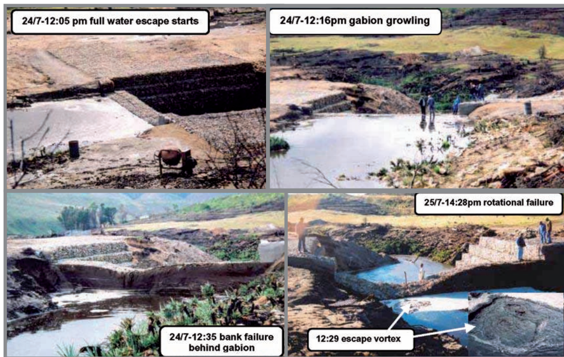
Figure 12: The collapse of an unfinished gabion structure B1. It rained on 22-25 July 2001 and at 11h00 on 24 July 2001. The pool behind the structure started filling up, by 12h00 water had reached the top of the gabion (top left). In the following 15 minutes water seeped under the gabion instead of overtopping the structure (top right) as can be seen by the surface disturbance. By 13h26 the people standing on top of the structure felt movement and heard groaning and soon afterwards the bank behind the gabion failed (bottom left). Overnight subsidence and rotational failure followed (bottom right). When the gabion was repaired, the height of the overflow was lowered by 2 m. After that the structure remained stable until 2006.
