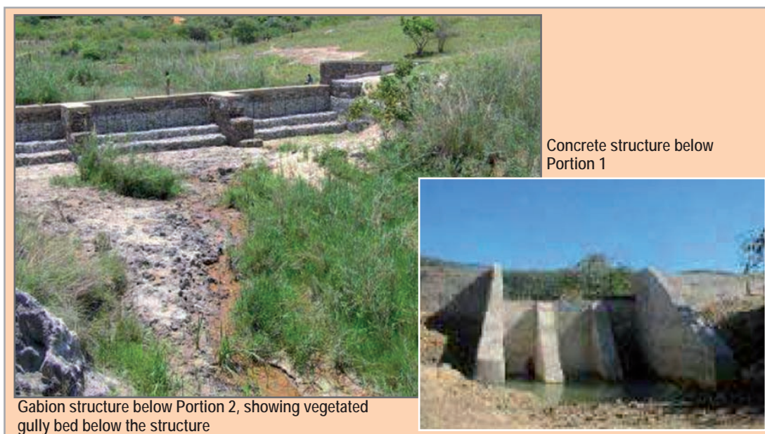
Figure 7: The two principal rehabilitation structures in the Manalana wetland
