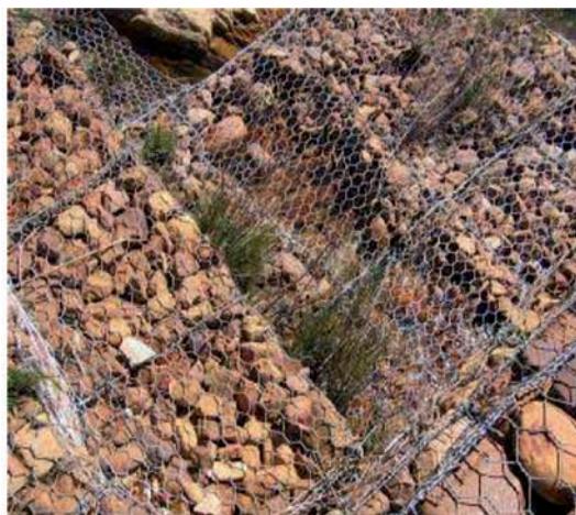
Figure 13: A view of gabion baskets with clasts missing at the Dwarsrivier structure (A1)
