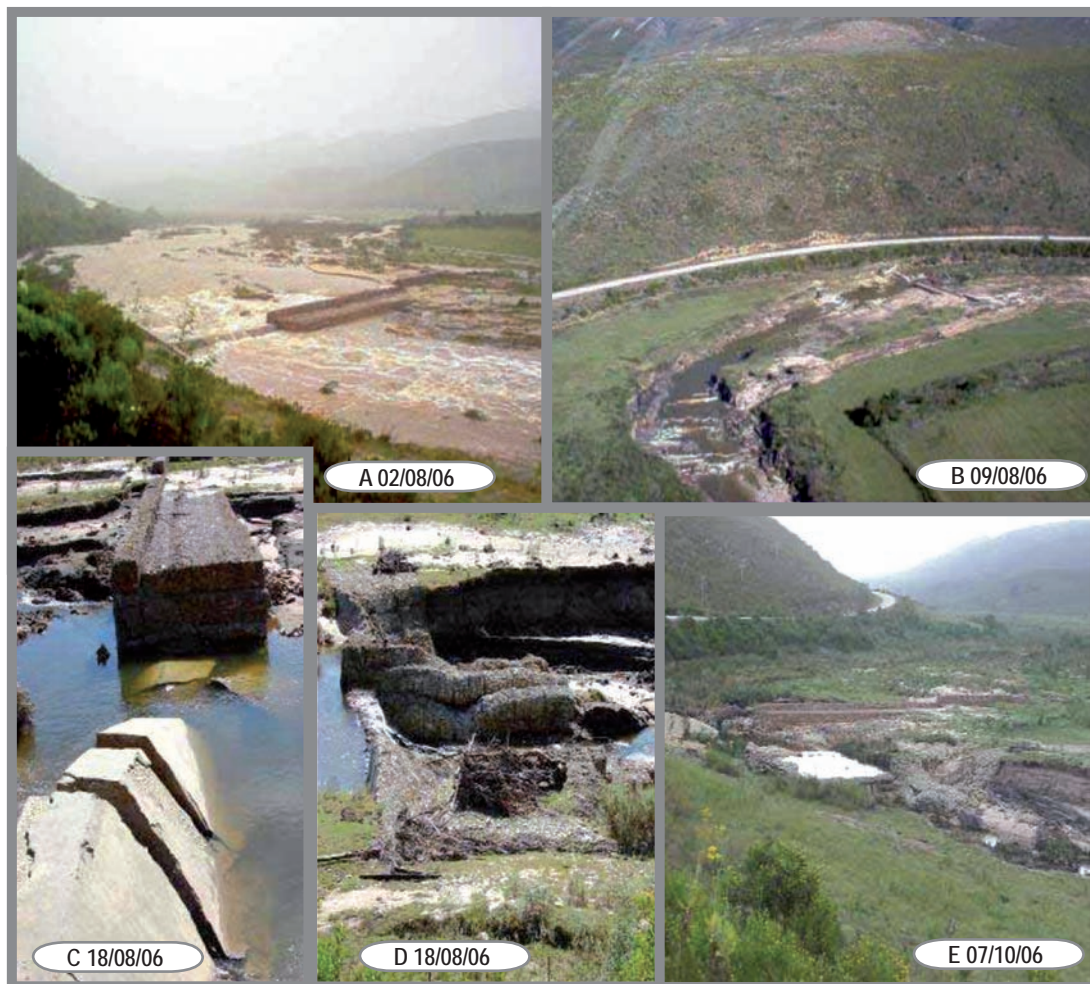
Figure 15: Sequence of events at the weirs B1 and B3 at Companjesdrift on the Kromme River, August 2006.
