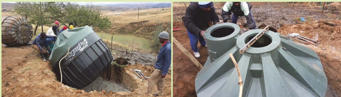
Plate 4-32: The new tank is carefully lowered into the hole (left), a spirit level is used to ensure that the tank is level on installation
