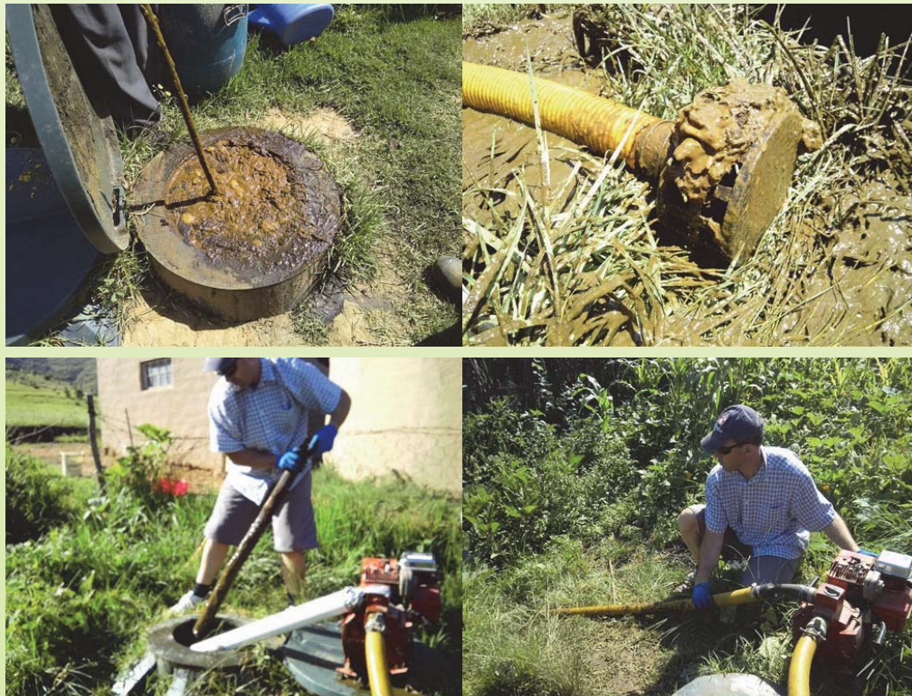
Plate 4-23: Clockwise from top left: blocked inlet chamber at capacity, slurry-pump filter blocked by solid matter, mixing the digester with a stick and slurry pump, emptying the digester
