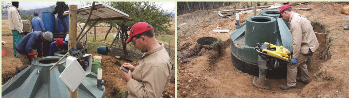
Plate 4-34: A remote monitoring station (see Case study 4.12) is installed at this site (left), the surrounding ground is lightly compacted as the tank is filled with water
