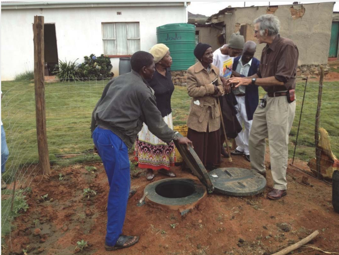
Plate 4-17: David Alcock fluently explaining the process of anaerobic digestion at a WRC K5/1955 pilot household in KZN
