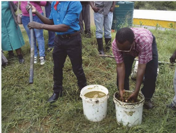
Plate 4-15: The manure-water mixture is mixed by hand or using an implement (left), and then poured into the digester once thoroughly mixed (right)
