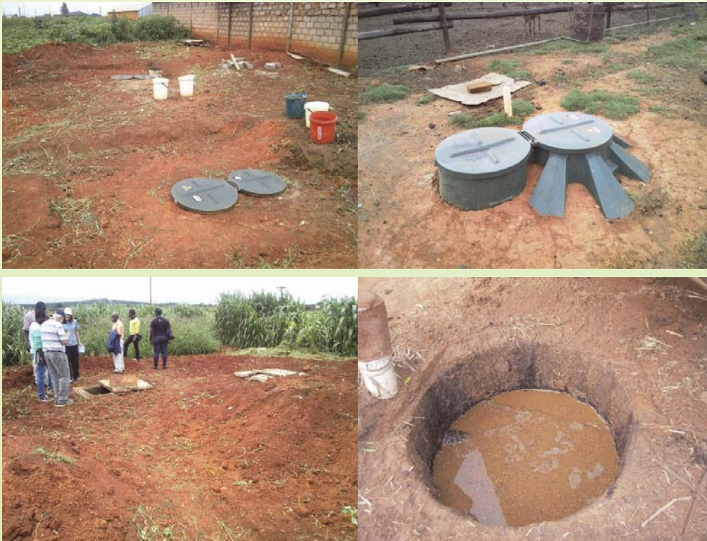
Plate 4-29: Clockwise from top left: A digester installed below ground level and prone to flooding; a digester installed slightly out of ground to avoid flooding; a flooded slurry collection tank; two slurry collection pits that will likely be flooded
