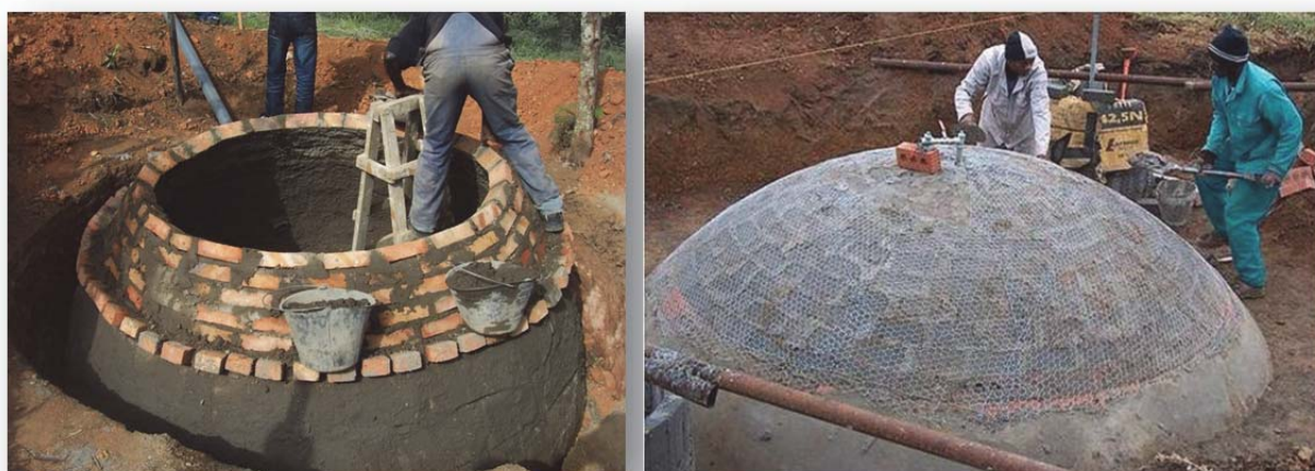
Plate 4-3: A fixed dome digester during construction and near completion (source: Tangka 2010; Lebofa 2006)
