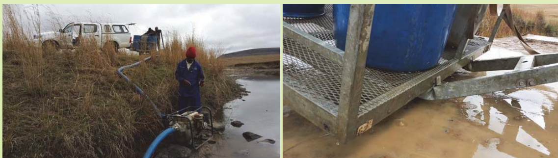
Plate 4-35: Collecting water from a river some distance away from the installation site (left), after a number of trips, the trailer broke under the load of water transportation along bad roads (right)
