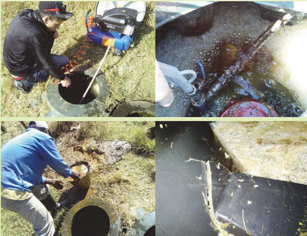
Plate 4-28: Tank pressurised to identify fault areas (top), cracks revealed after digestate was removed to drop water/digestate level (bottom).
