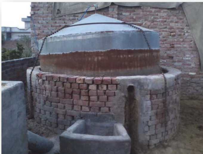
Plate 4-4: Examples of floating dome digesters (source: Biogas Technology 2011; Technology Times 2011)
