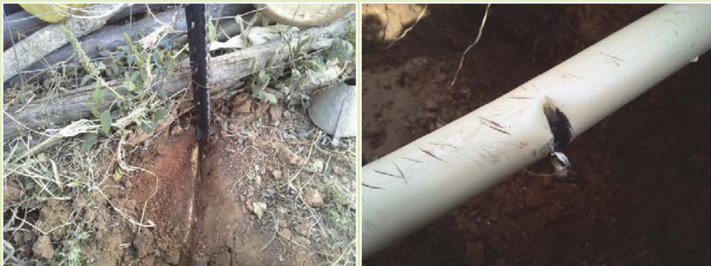
Plate 4-27: Fence post hammered into the ground (left), gas line cut caused by fence post (right)
