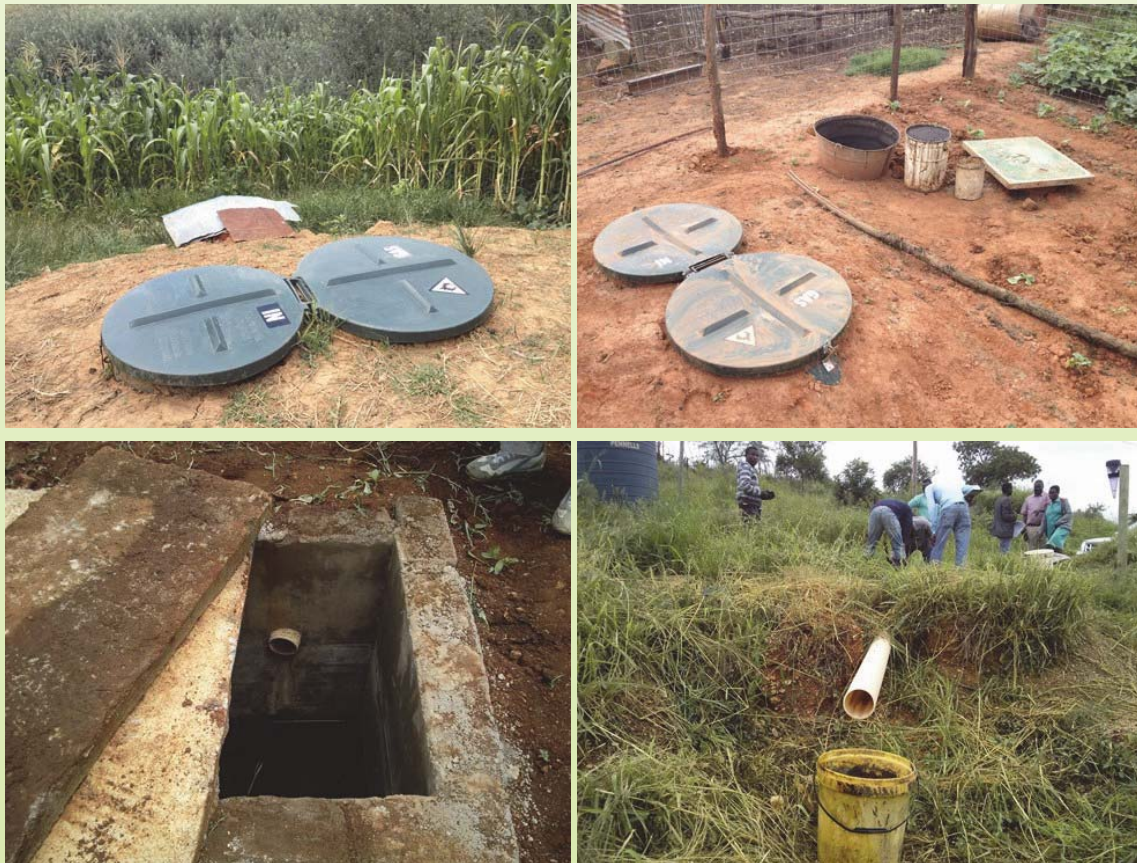
Plate 4-22: Clockwise from top left: digester installed on slope, digester installed at location with no slope, large slurry collection pit, slurry outlet installed on a slope below the digester
