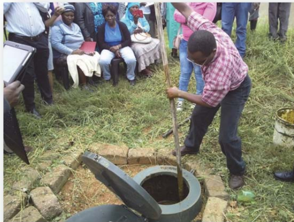
Plate 4-16: The inlet can be mixed with a stick, after feeding or on alternating days
