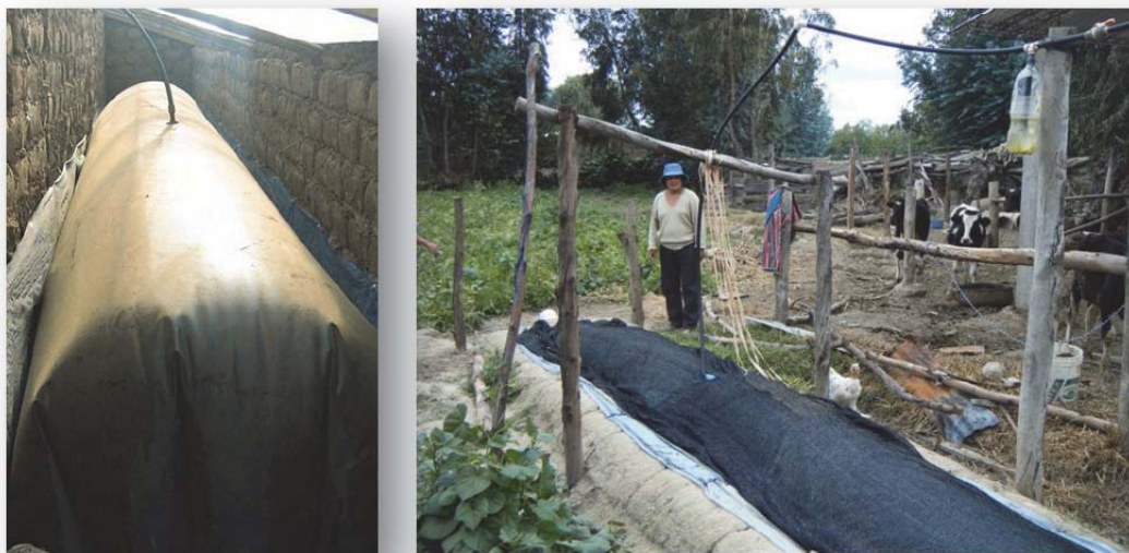
Plate 4-2: Various tube digester installations – style and size can vary greatly (source: Energypedia 2010; Weatherford, 2010)
