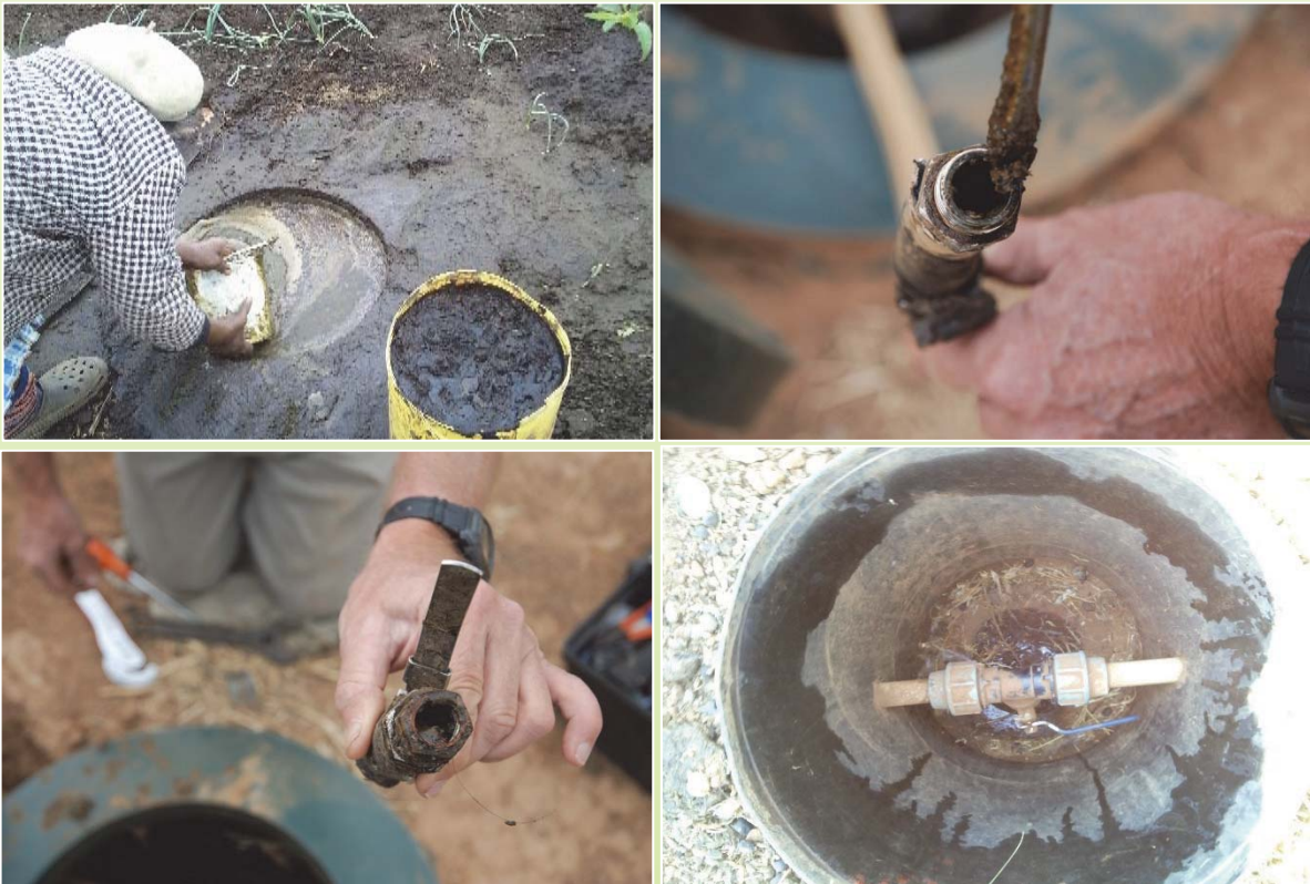
Plate 4-21: Clockwise from top left: overflowing slurry pit, blocked gas line, blocked gas valve, moisture trap
