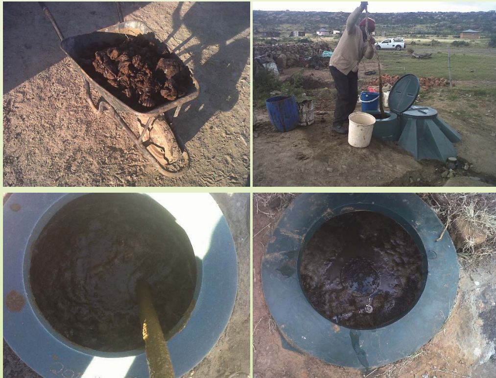
Plate 4-26: Clockwise from top left: (a) Cattle dung serves as the primary feedstock, (b) Additional mixing of feedstock within the biodigester, (c) Consistency of the feedstock is very thick and additional water is added and (d) evidence of overloading the digester as material accumulates above gas inspection hatch.
