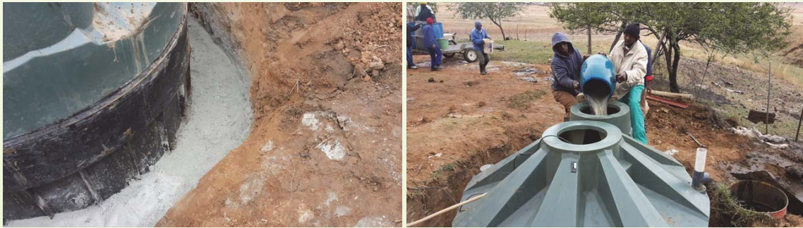
Plate 4-33: The soil around the tank is mixed with cement for stabilisation, this can be done to varying degrees as required per site (left), the tank must be filled with water as sand is compacted around the tank – this is necessary to avoid the tank collapsing inward from external pressure (right)
