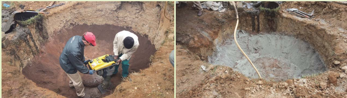
Plate 4-31: The hole is prepared with a sand base and using an automated or manual stamper (left), cement and sand is used in various ratios to stabilise the soil as required (right)
