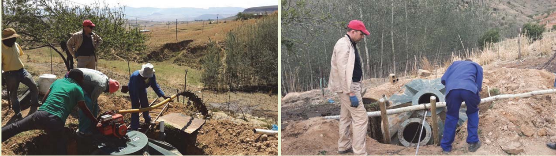
Plate 4-30: The old tank must first be emptied (left), poles are used to help slide the tank out as it is pulled with a chain
