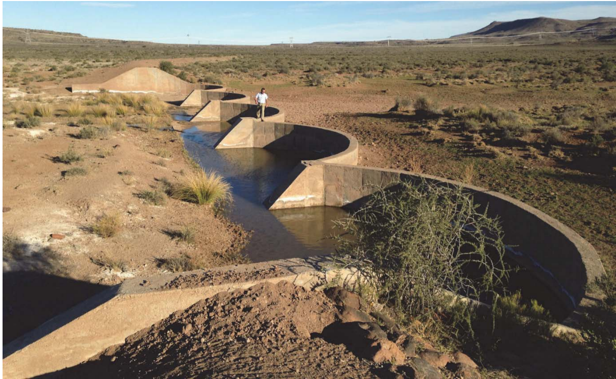
Figure 5.33: Incision control weir near 3 Sisters, Karoo
