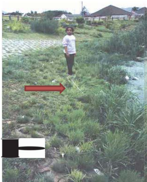
Figure 10.17: Vegetation established in planter blocks set into canal wall – left hand photo in 2002, one year after construction, and right hand photo 14 years after construction, showing dense kikuyu grass over planted areas (arrowed)
