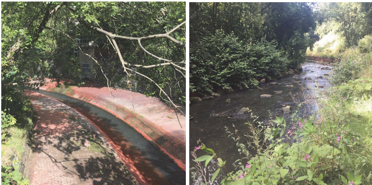
Figure 10.15: Un-rehabilitated, canalised section of the river Medlock (Manchester, United Kingdom) (left hand photo) and upstream, post rehabilitation channel (right hand photo), showing removal of concrete channel base, addition of rocks to improve instream habitat diversity and establishment of marginal vegetation. Canal side walls largely retained because of concerns around possible contaminants in fill on either side of the channel. Note how the same discharge is conveyed in each of the two channels, illustrating the role of canals in speeding up rate of flow
