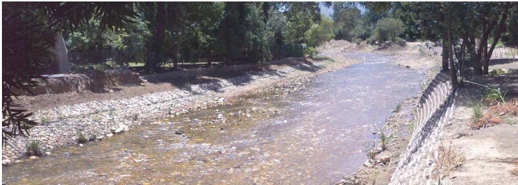
Figure 4.62: A river channel with gabion mattresses on the one bank and Loffelstein blocks on the other. The river is on a bend and more aggressive flow was expected along the outer bend, hence the use of concrete blocks.
