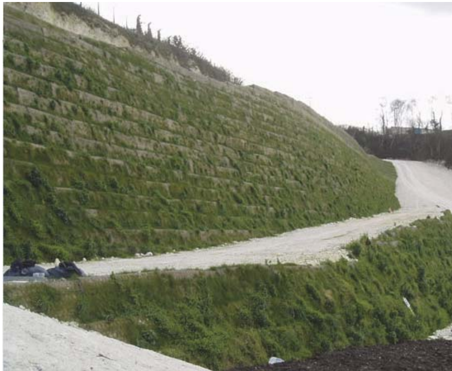
Figure 4.43: A "Green Terramesh" retaining wall
