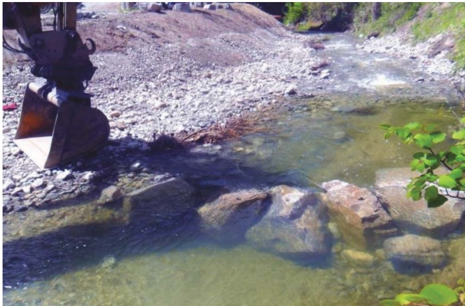
Figure 4.16: Construction of micro-groyne (photo C Sindelar, Austria)
