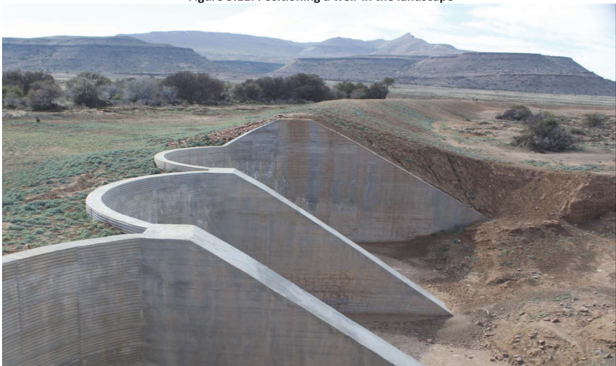
Figure 5.12: Typical river incision arrest structure in the Karoo with long earth banks to collect water that would otherwise have bypassed the structure in other gulleys
