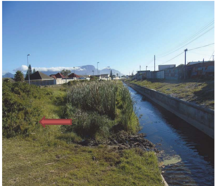
Figure 10.17: Vegetation established in planter blocks set into canal wall – left hand photo in 2002, one year after construction, and right hand photo 14 years after construction, showing dense kikuyu grass over planted areas (arrowed)
