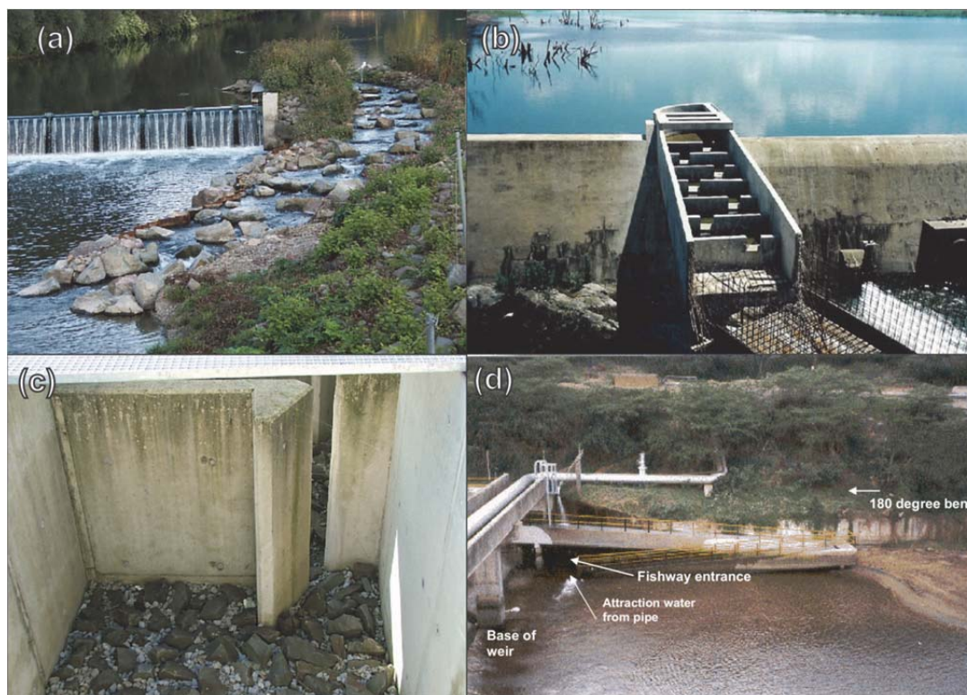
Figure 11.2: (a) A natural bypass channel on the Lenne River in France; (b) Pool and Weir fishway (notched) on the Lebombo gauging weir, Komati River; (c) a Vertical Slot fishway in Germany and (d) the Nhlabane fishway on the Nhlabane estuary showing the attraction water (from Bok et al. 2007).
