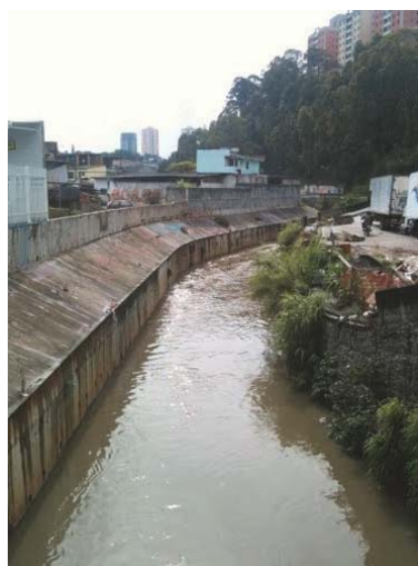
Figure 5.26: Steel reinforced concrete lined canal
