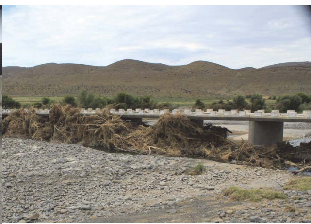
Figure 3.2 Debris dam against bridge piers (woody vegetation flotsam blocking bridge) (photo: H. King)
