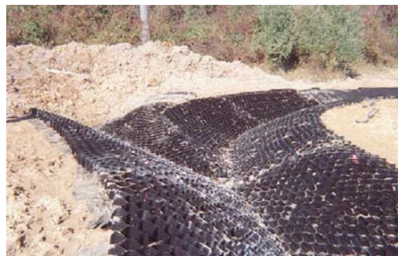
Figure 4.25: Geo-cell prior to soil fill used to reinforce channel. This can be a good solution if the cells are filled with cementitious material and the flow velocities are not too high. It is however more appropriate for addressing surface drainage than river stabilisation.
