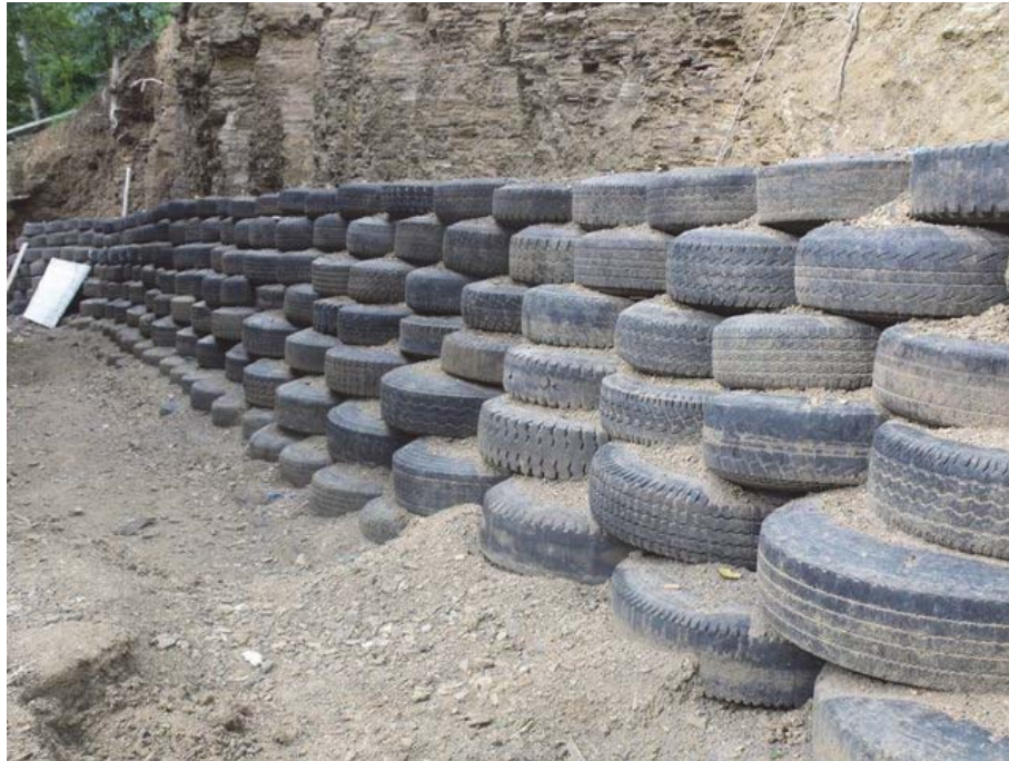
Figure 4.51: Retaining wall made with used tires
