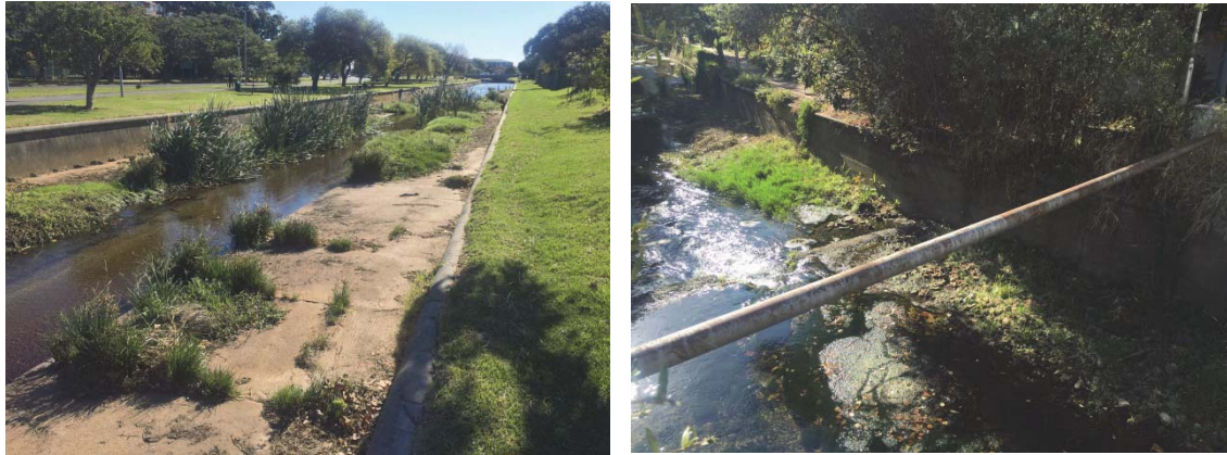
Figure 10.8: Natural establishment of vegetation on sediment in lined canals
