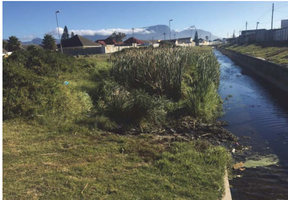
Figure 10.3: Removal of canal wall along a length of 60 m and creation of a small area of planted but still hard stabilised riverine habitat, 7 m (maximum) width
