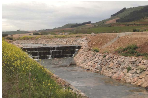
Figure 4.36: Many river channels in Spain are protected with a large stone facing which is very similar to rip-rap in principle
