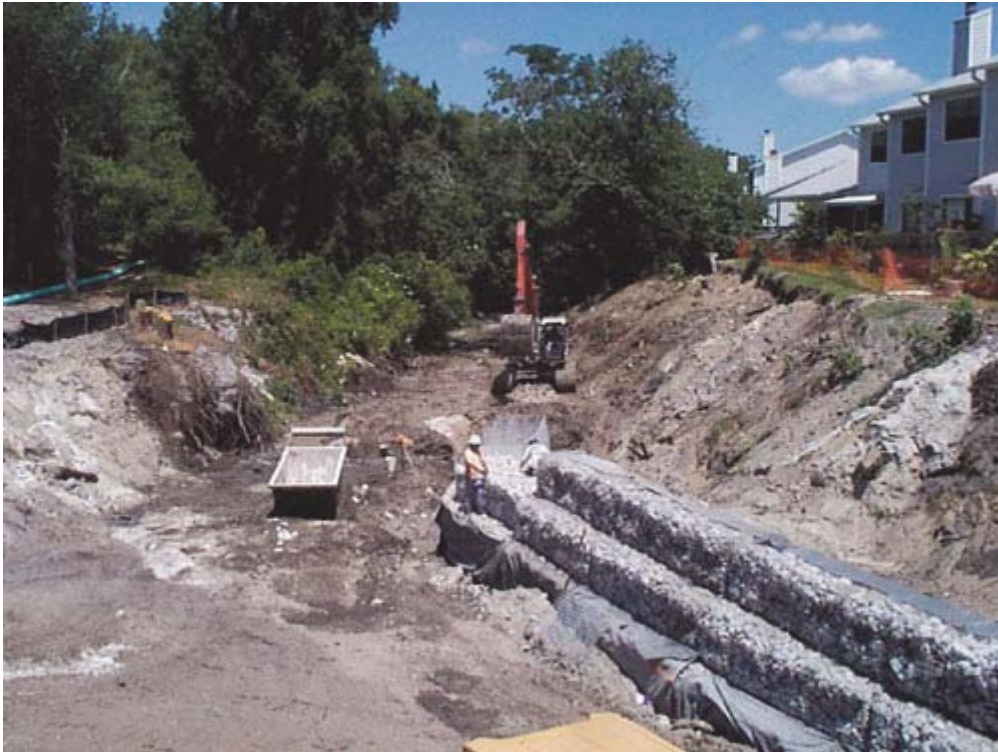
Figure 4.37: A retaining wall being constructed as a river training wall
