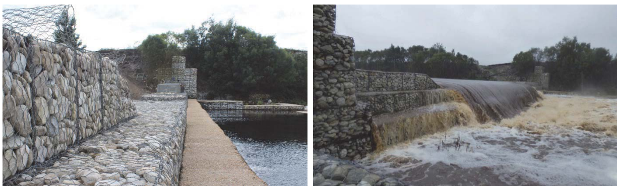
Figure 5.34: A weir on the Duiwenhoks River during construction (left) and during 1:5 year flood right. Although it is only a small flood, the energy of the water is high because it is falling more than 2 metres – imagine what a 1:50 year flood would look like. For this reason consider that it is a simple matter to detail a structure on a plan, but to ensure that a structure is designed to be stable under severe conditions can be very challenging and should only be undertaken by persons with appropriate qualification and experience.
