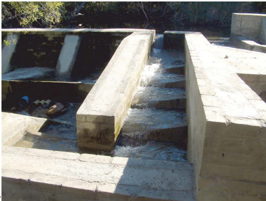
Figure 5.21: Fish ladder constructed with masonry and concrete (Piketberg). In order to discharge at the point where the weir’s water falls back into the stream, this fish ladder turns back on itself.
