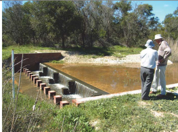
Water extraction weir discharging low flow into irrigation canal (masonry)
