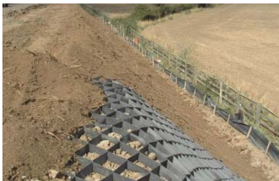
Figure 4.24: Geo-cell used to stabilise slope This can be very effective for slope stabilization, but not in the presence of fast flowing water.
