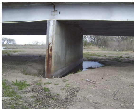
Figure 3.1 Local scour around bridge pier (source: internet)
