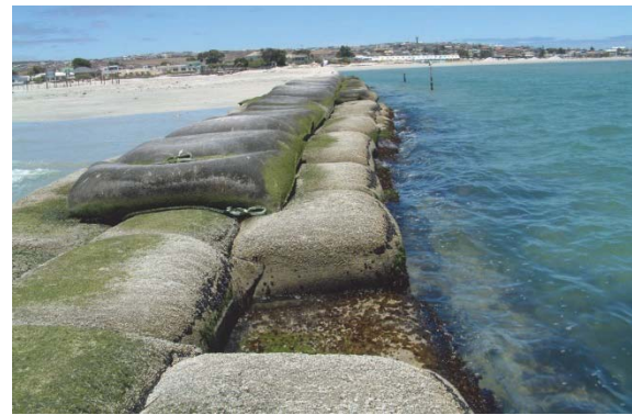
Figure 4.23: Large sand filled geobags used to construct groynes in the sea at Langebaan
