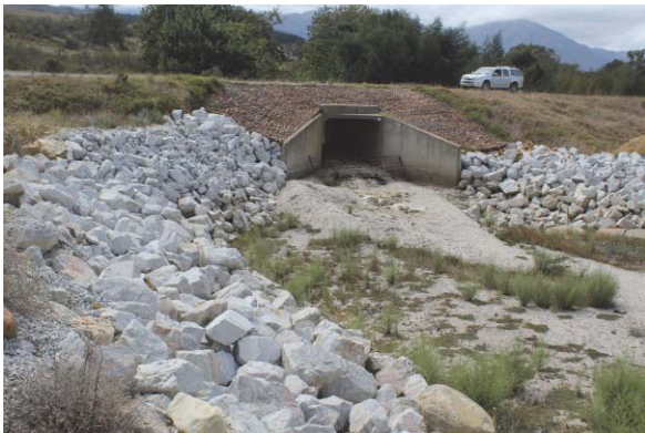
Figure 4.35: Rip-rap protecting river banks from scour at culvert outlet (Genadendal)
