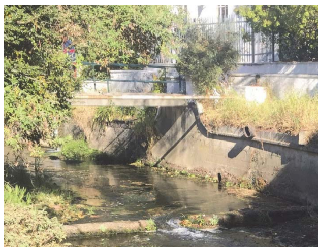
Figure 10.9: Low weirs increase habitat diversity, limit pedestrian use of canals and have been designed to have a negligible effect on flood levels
