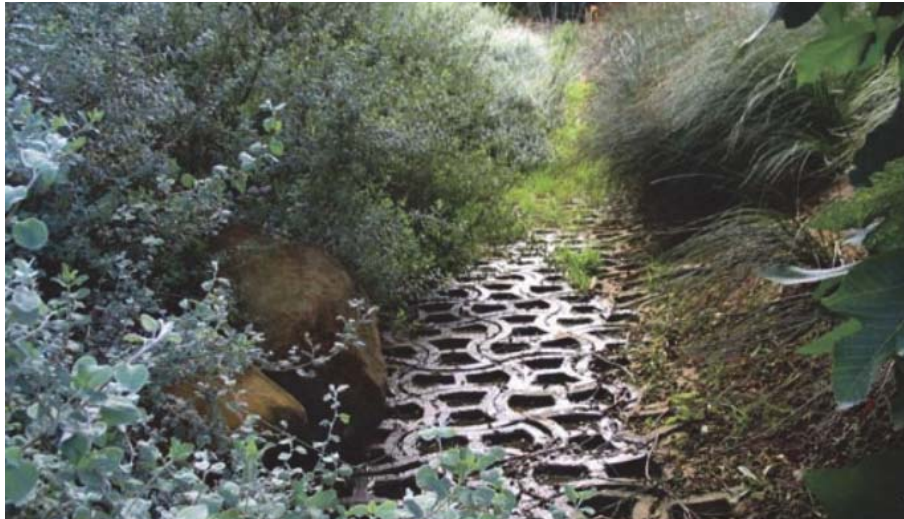
Figure 4.60: Channel with concrete block base to prevent erosion but still to allow growth of plants
