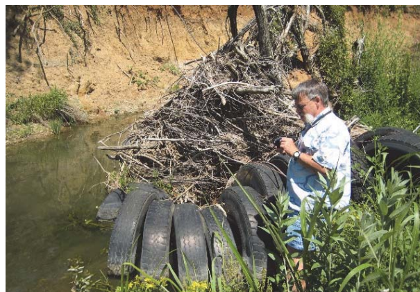
Figure 4.53: The remains of a typical failed tyre structure
