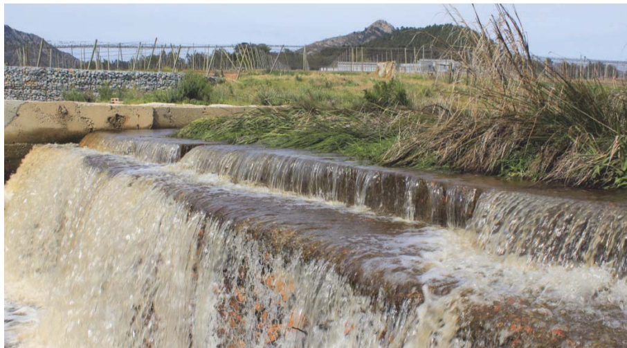
Figure 5.16: Typical vegetation growth upstream of a spillway reducing its discharge capacity (this must be taken into account in the design phase)
