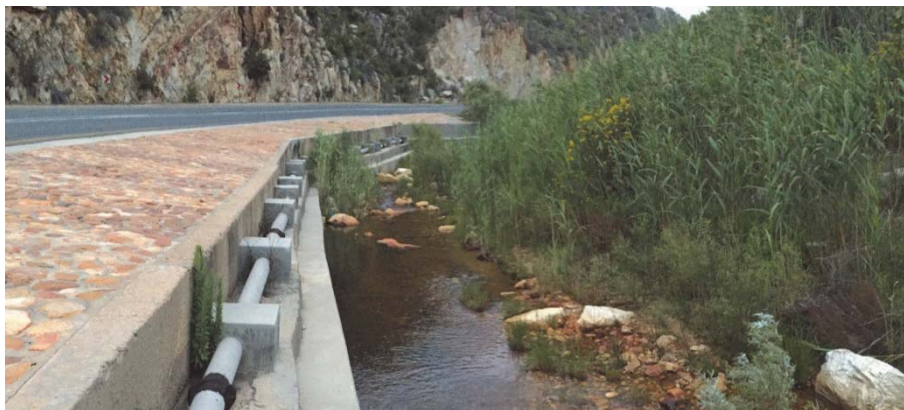
Figure 4.50: Reinforced earth retaining wall protecting a road from river
