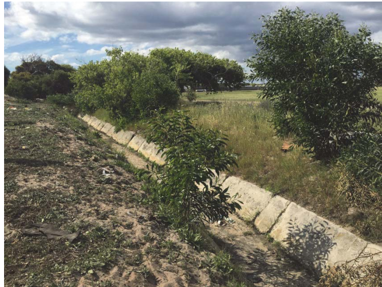
Figure 10.16: Small canals such as this seasonally dry system lend themselves to removal of canal walls and (ideally) base, shaping of the banks and planting with indigenous vegetation.
