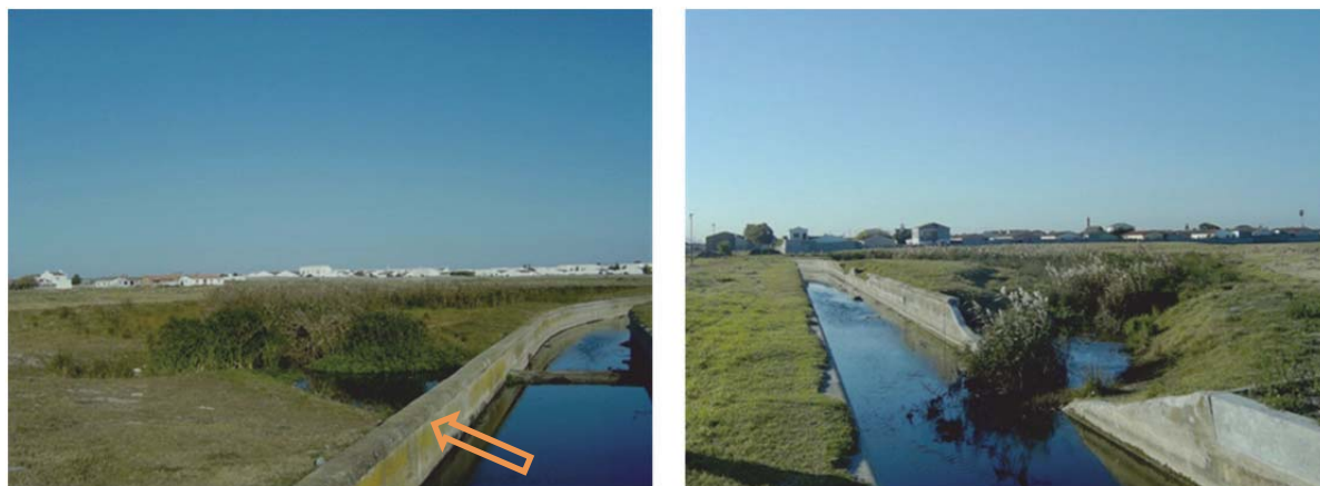
Figure 10.14: Low flow outlet (arrowed) from Langvlei Cana, Retreat, Cape Town (left) and downstream inlet from low flow channel (right), showing creation of broad reedbed wetland and low flow channel outside of the lined canal. See Volume 3: Case Study 16
