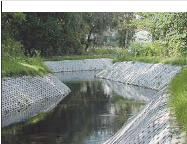
Figure 4.29: Channel protected with flexible block armoring
