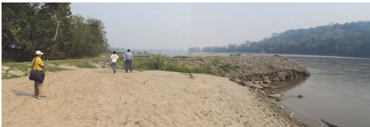
Figure 4.5: Erosion control groyne on bank of Upper Amazon at Campanilla, Peru. The river is too wide for the structure to influence the opposite bank
