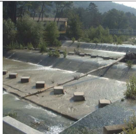
Stepped bed erosion control weir (gabion and concrete) – Italy
