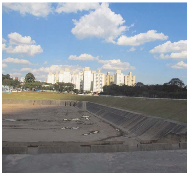
Figure 4.58: 8 m deep storm water detention pond Sao Paulo
