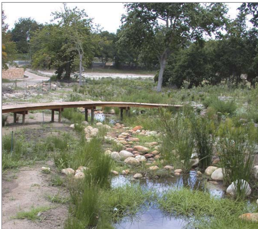
Figure 10.7: Planting of recently reshaped and widened stream in Cape Town residential estate. Initial condition was narrow (<1 m wide) trench through alien vegetation
