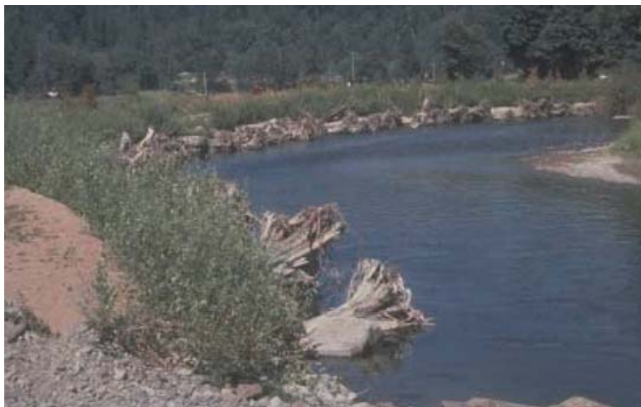
Figure 4.40: Tree stump erosion protection (Alberta Fish Habitat Manual)
