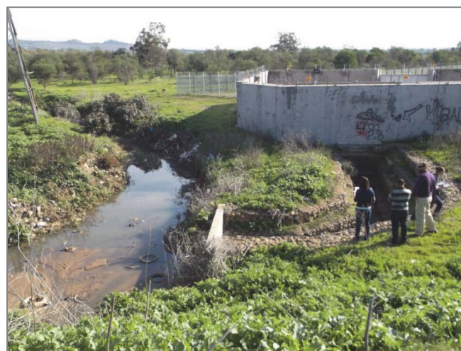
Figure 8.2: Low flow diversion to the sewer from a tributary of the Berg River at Mbekweni mixed informal / formal settlement near Wellington in the Western Cape.
