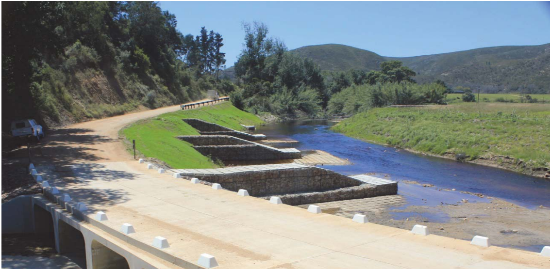
Figure 4.6: A typical river where rehabilitation work on one bank can influence the stability of the opposite bank
