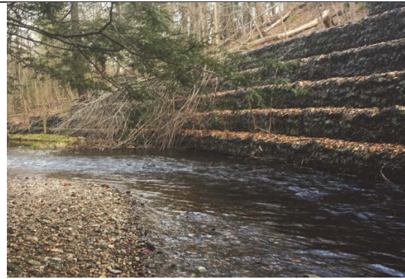
Figure 4.46: Gabion retaining wall ( https://theriverfinn.files.wordpress.com/2014/04/20140428_170047_1.jpg )
