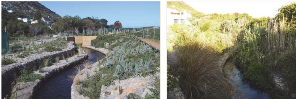
Figure 10.11: Creation of planting areas behind gabions on the Silvermine River, Cape Town. LHS: 2002, immediately after planting; RHS: 2009, showing plant establishment. Planted areas comprised bidim® lined, soil filled spaces behind the lower gabion, allowing plant roots access to water
