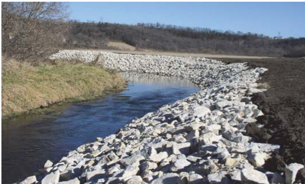
Figure 4.33: Riprap erosion protection on a river bank
