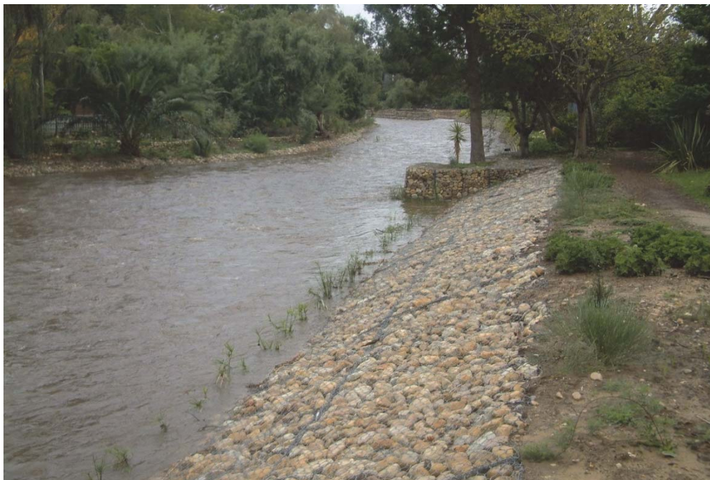
Figure 4.28: Gabion mattress protection stabilizing a river bend (Lourens River)
