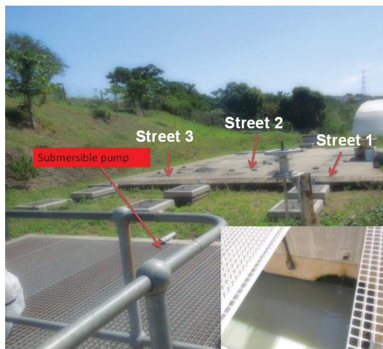
Figure 3.4 Layout of the anaerobic baffled reactor at Newlands-Mashu
