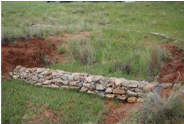
Figure 4.11: Use of stone lines and stone packs to control gully erosion
