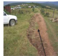
hard surface / roadway
