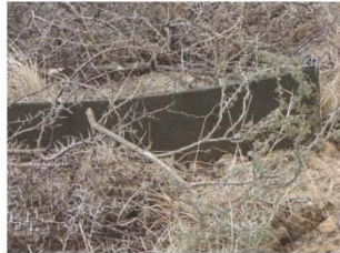
Brush pack and silt fences in a reshaped donga
