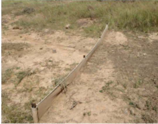
(a) SILT FENCES Silt fences constructed from hessian can be placed across shallow drainage lines to trap sediment. Vetiver can be planted along the line of the silt fence to continue its trapping function after the fence has decayed. Silt fences made of hessian are vulnerable to fire.
