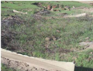
Brush pack and silt fence stabilise a shallow donga
