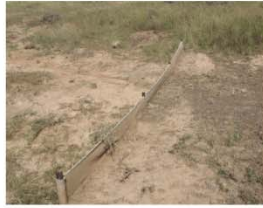
A silt fence traps soil and helps plants grow
