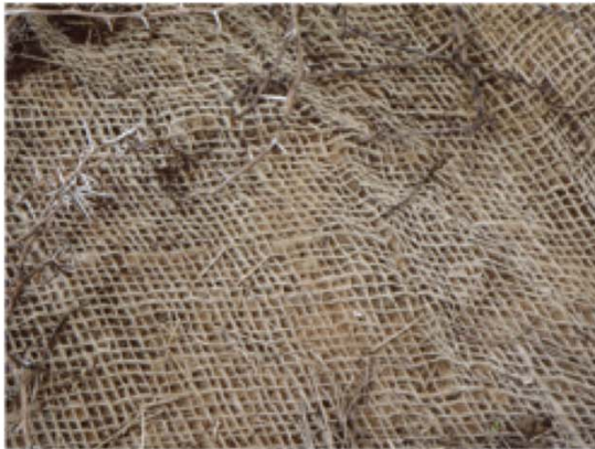
(c) NETTING Netting on a gully floor
