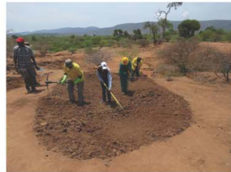
Re-sloping a small donga. The side walls and head cut are dug away to give gentler slopes. The widened donga is protected with a blanket and silt fence.
