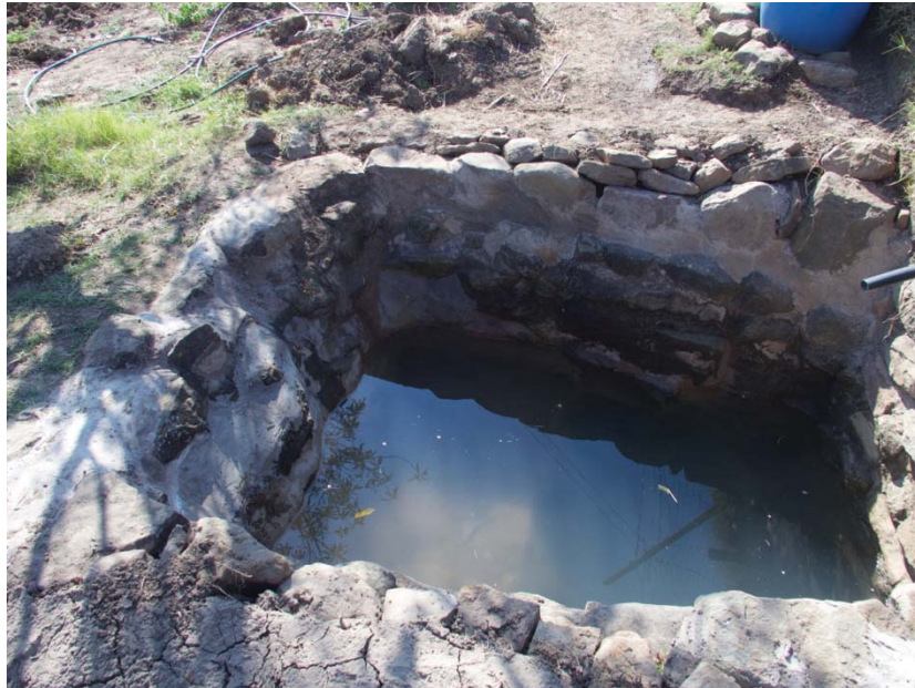
Figure 5.14: A small water storage dam constructed in a garden in Sinxaku for watering vegetables
