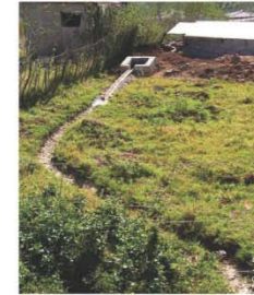
Figure 1 Diversion furrow leading to a catchpit
