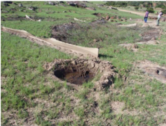
(c) Micro-pond, brush packing and silt fencing used in combination to reduce surface runoff and stabilise a shallow gully.
