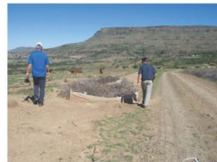
Brush pack and silt fences alongside a road
