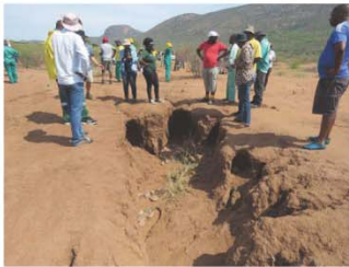
Re-sloping a small donga. The side walls and head cut are dug away to give gentler slopes. The widened donga is protected with a blanket and silt fence.
