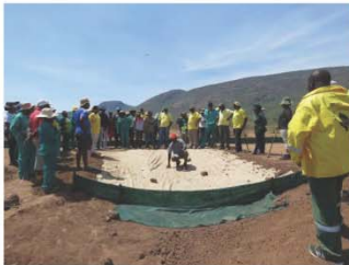
Re-sloping a small donga. The side walls and head cut are dug away to give gentler slopes. The widened donga is protected with a blanket and silt fence.
