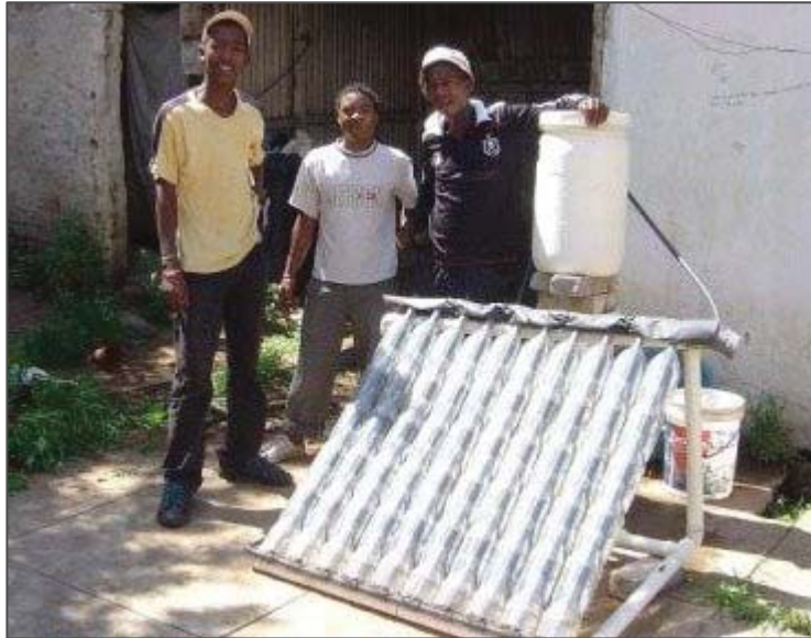
Figure 3.9: A 'home made' coke bottle low pressure solar water heater (source: Tony Lopes, lowtech 25 )
