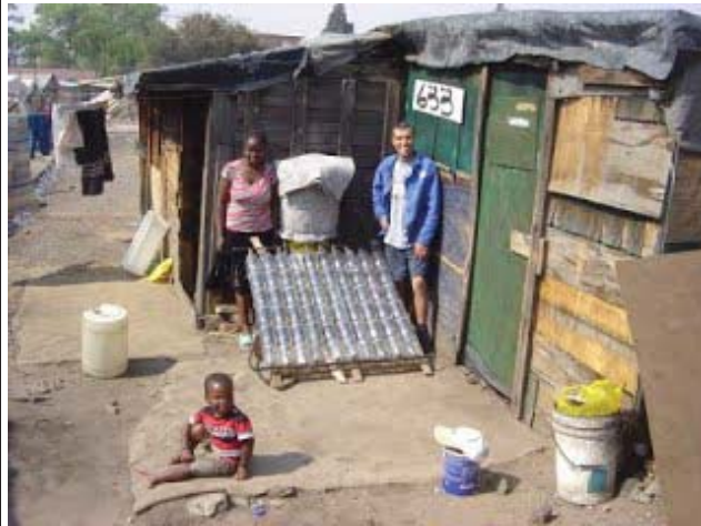
Nomusa at 633 Denver squatter camp with her 10 column array geyser and 60 litre container. Her paraffin bill has halved.
