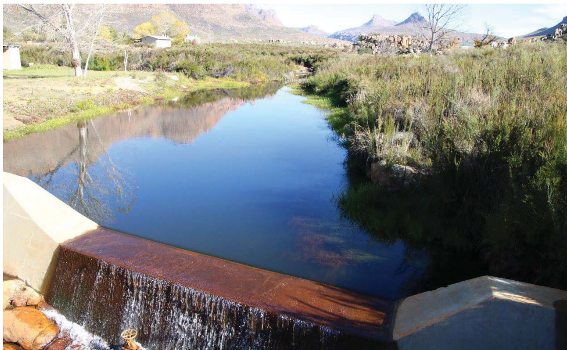
Barrier weir on the Krom River constructed by the Cederberg Tourist Park within the Resort area in support of the proposed fish conservation project (Photo Sean Marr).
