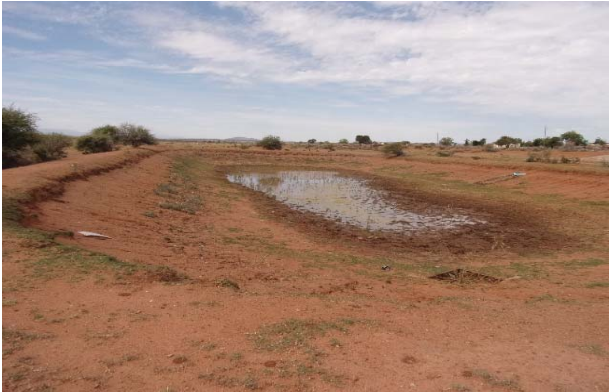
Figure 23: Showing the position of the balancing dam which is now non-functional
