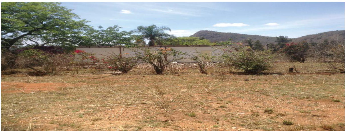
Figure 14: Vandalised coffee pack house
