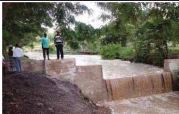
Figure C.4.2-2: Sand dam. (Source: Africa Harvest)
