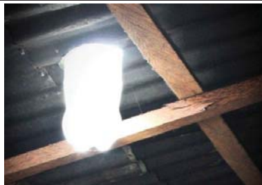
Figure E.6.1-7: Solar bottle bulb (clean plastic bottle, water and bleach)
