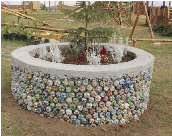
Figure E.6.2-2: Ecobrick tree basket
