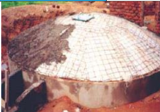
Figure C.2.2-7: Covering the roof of the tank with mortar
