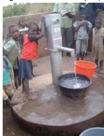
Figure E.3.2-3: Borehole pump. (Source: Joissam Ghana Ltd. 2015)
