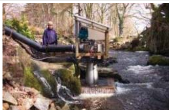
Figure E.5.7-2: Cross-flow turbine b
