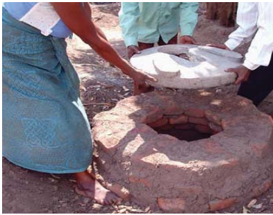
Figure E.4.2-8: Installing small slab on ring beam for Arborloo (Photo: Peter Morgan)
