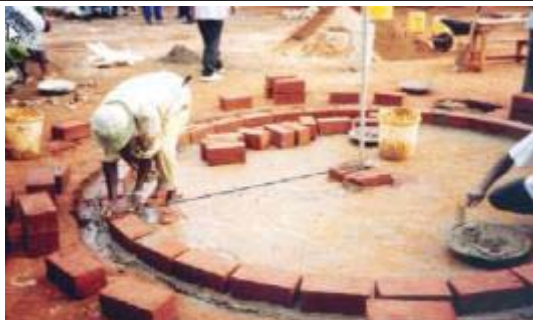
Figure C.2.1-4: Foundation of tank
