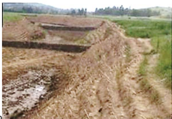
Figure A.4.6-2: Severe gully erosion before (top) and after reshaping (bottom) including check dams across the gully to manage runoff. Gully banks are stepped for revegetation. (Source: Researchgate)
