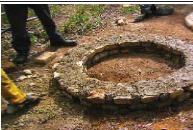
Figure E.4.2-5: Ring beam (circular brick collar)
