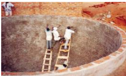
Figure C.2.2-5: Plastering the inside of the tank
