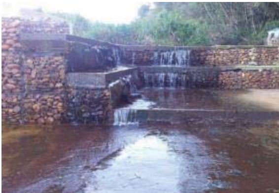
Figure A.5.4-3: Example of gabion structure used to guide watercourse (Source: F. Nagdi).
