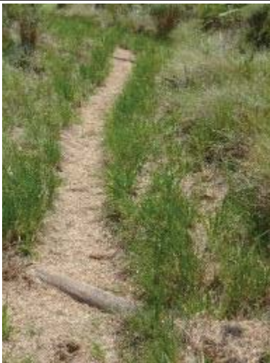
Figure A.2.4-4: Small wooden poles to direct runoff off the path, and path covered with cut grass when muddy to prevent erosion.
