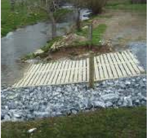
Figure A.5.2-5: Cattle crossing should have a hard surface to enter and exit the water, to prevent mud and siltation of the watercourse, prevent bank erosion, and make it easier for the cattle to enter and exit.
