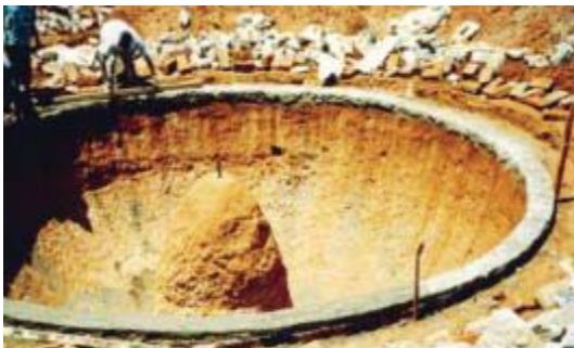
Figure C.2.2-3: Ring beam around the top of the tank
