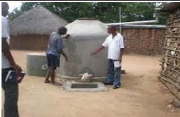
Figure C.2.1-2: Rooftop rainwater harvesting tank
