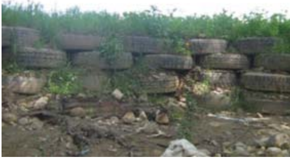
Figure A.5.4-1: Stacked tyres providing bank protection (Source: S. Braid).
