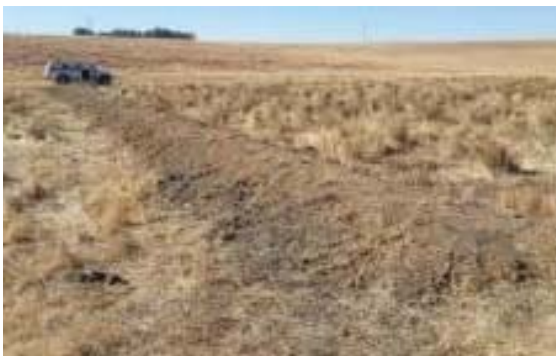
Figure A.5.3-2: Unlined earth berm (F. Nagdi)
