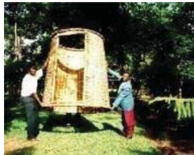
Figure E.4.2-12: Portable superstructure of an Arborloo
