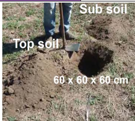
Figure E.3.1-8: A ready planting pit
