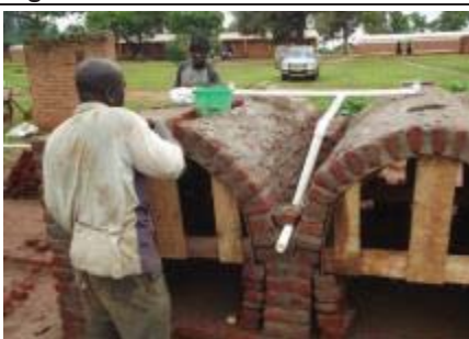
Figure E.4.1-5: Constructing a composting toilet
