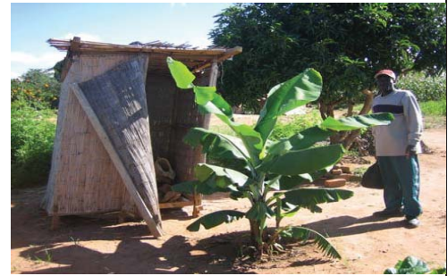
Figure E.4.2-10: Completed Arborloo
