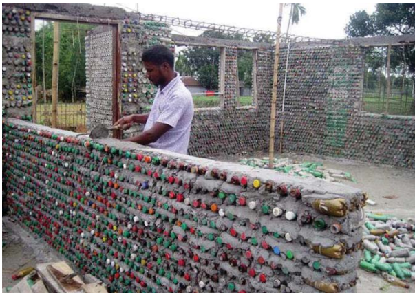
Figure E.6.2-3: Laying Ecobricks as walls of a house.
