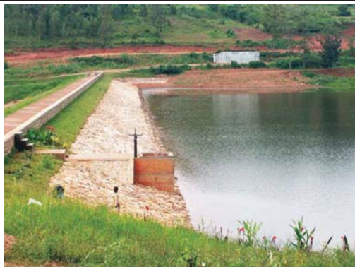
Figure C.4.3-3: Slopes of an earthfill dam
