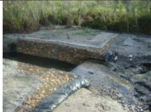
Figure A.5.4-2: Example of gabion structure used to guide watercourse (Source: F. Nagdi).
