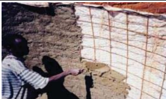
Figure C.2.1-6: Plastering of mortar
