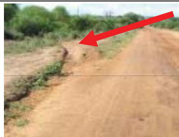
Figure C.2.3-4: Rainwater to be diverted into ditches through diversion
