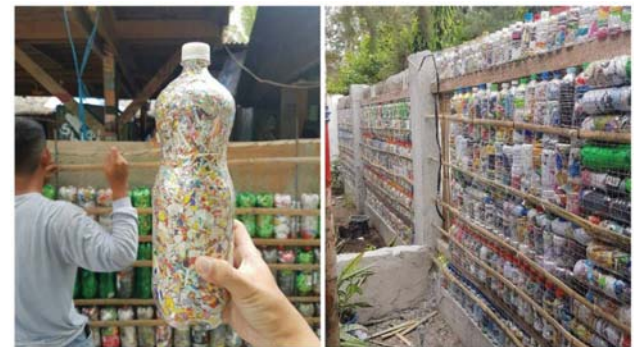
Figure E.6.2-6: Ecobrick Fences and walls
