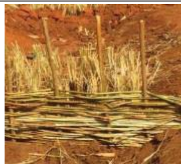
Figure A.4.4-5: A vegetation barrier, with woven material, and a strip of vetiver grass upstream. (Source: S. Braid)
