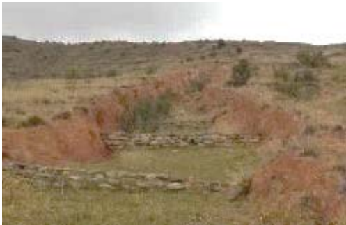
Figure A.4.3-4: Stone check dams in Tukela catchment. (Source: S. Braid).
