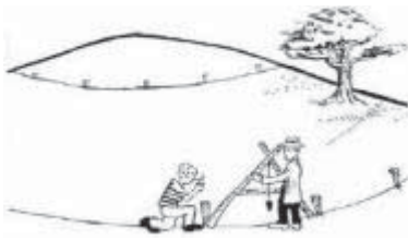
Figure C.3.1-1: Stone bunds – Mark out contour lines
