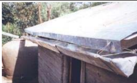
Figure C.2.1-9: Splash guard gutter filling tank
