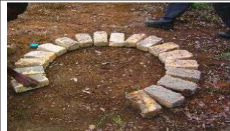
Figure E.4.2-4: Ring beam (circular brick collar)
