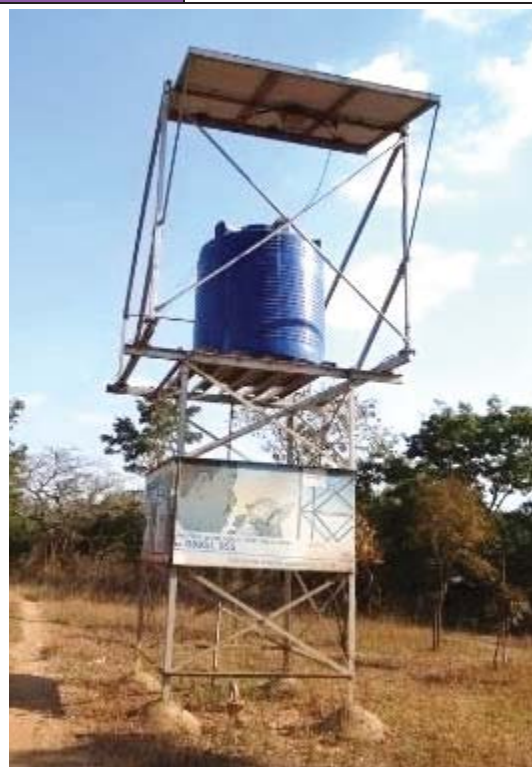
Figure E.5.5-2: Solar borehole pump. (Photo: S. Braid)
