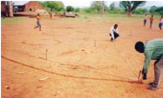
Figure C.2.2-1: Measuring the tank and marking with wooden pegs.
