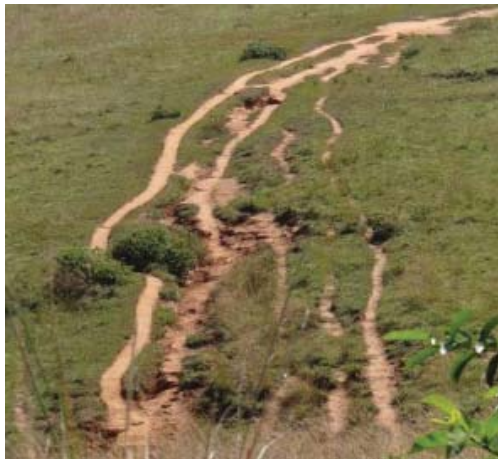
Figure A.4.1-2: Unmanaged erosion, e.g. along footpaths and livestock tracks can rapidly progress into gully erosion (S. Braid).
