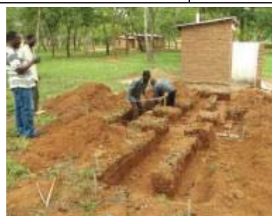
Figure E.4.1-6: Constructing a composting toilet
