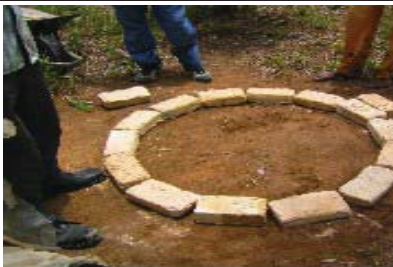
Figure E.4.2-2: The mould for a circular slab
