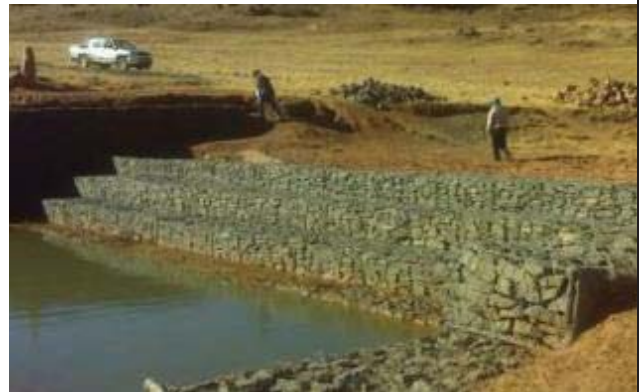
Figure A.5.4-4: Example of gabion structure used to guide watercourse (Source: F. Nagdi).
