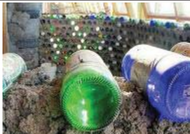
Figure E.6.1-6: Glass bottle wall
