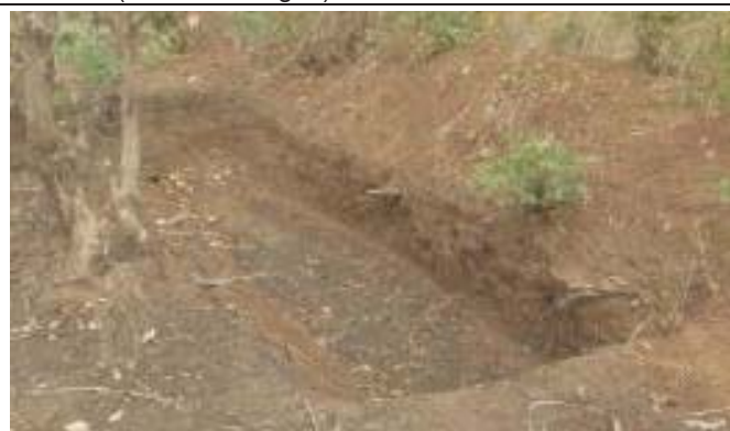
Figure C.3.4-2: Completed infiltration trench.
