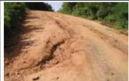
Figure C.2.3-5: Erosion on the road if no water harvesting mechanism
