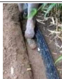
Figure D.5.4-4: Plastic barrier being installed in trench b .
