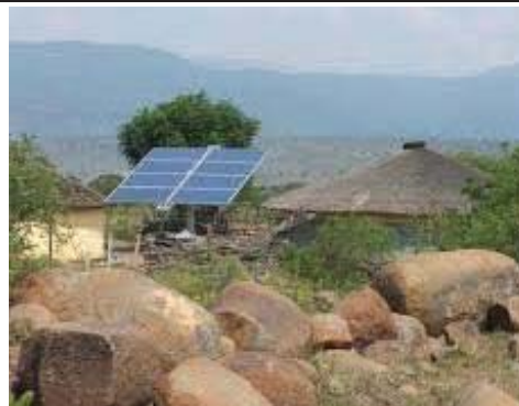
Figure E.5.4-2: Solar panels
