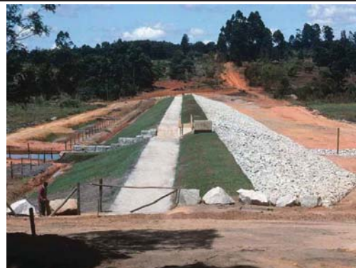
Figure C.4.3-4: Construction of a farm dam
