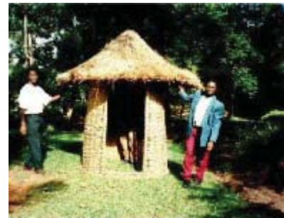
Figure E.4.2-13: Portable superstructure of an Arborloo
