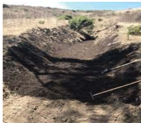
Figure A.4.6-4: Manual reshaping o gully bed and banks to a gentler slop.
