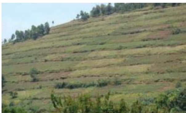
Figure 4-13: Example of aligned contour bunds across adjacent plots = good practice
