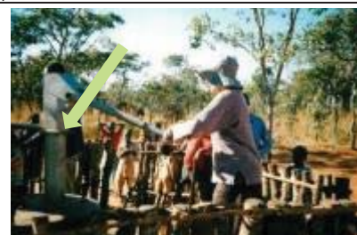
Figure E.3.2-7: Flange Bolts and Nuts – Check that these nuts are tight. (Source: Joissam Ghana Ltd. 2015)
