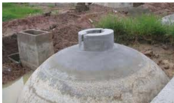
Figure E.5.8-4: Biogas digester c
