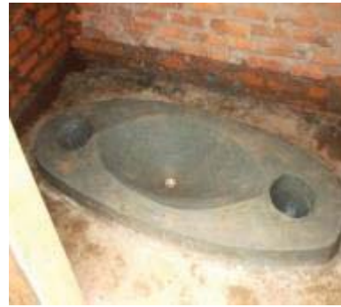
Figure E.4.1-10: Inside a composting toilet. (Photos: T. Mahoney)
