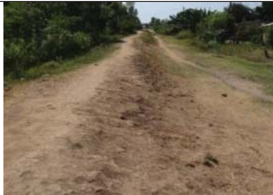
Figure A.5.3-3: Berm – well vegetated on left poor condition on the right, e.g. cattle walking over it breaking it up (S. Braid).
