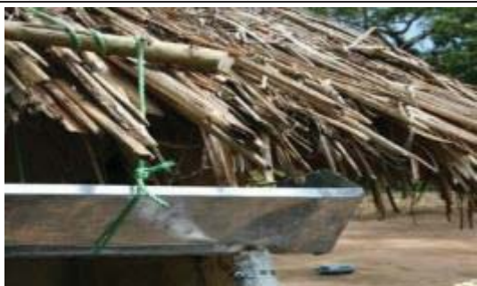
Figure C.2.1-8: Steel gutter fitted to roof
