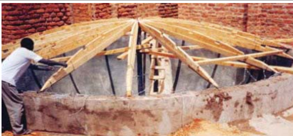
Figure C.2.2-6: Wooden frame and support for the roof of the tank.
