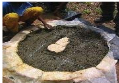
Figure E.4.2-3: The mould and slab casting for a circular slab
