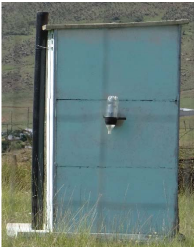
Figure E.4.4-2: Tippy Tap on a VIP Latrine, Bergville. (Source: S. Braid)
