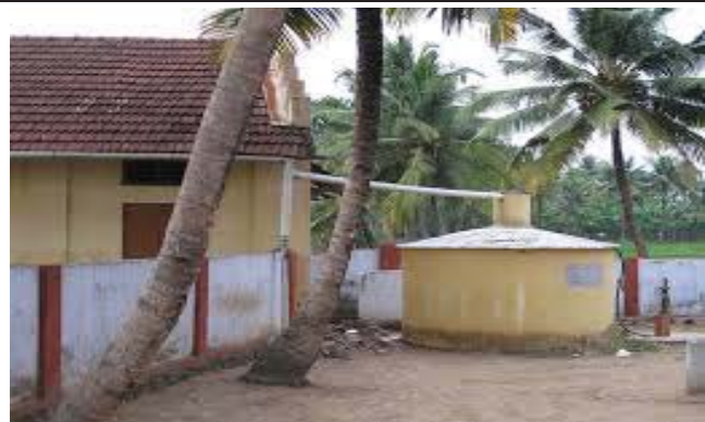
Figure C.2.1-3: Rooftop rainwater harvesting tank
