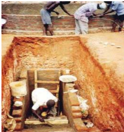
Figure C.2.2-4: Small wall and stairs into the base of the tank
