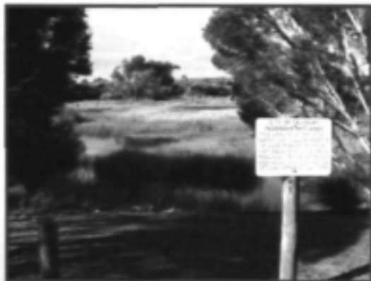
A wetland in Adelaide, Australia that was constructed to treat urban storm runoff prior to borehole injection
