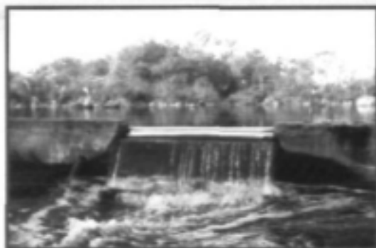
Treated wastewater discharging into the Sand River
