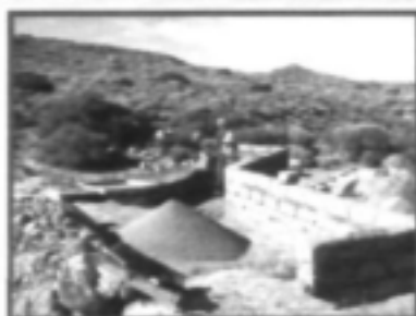
Sieving river sand for the sand filter
