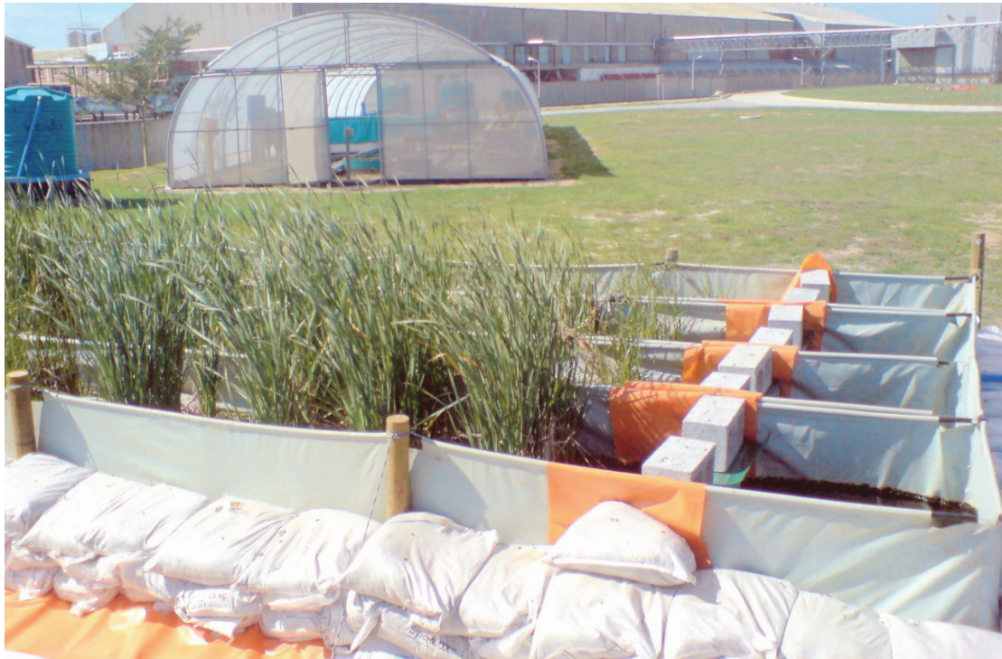
Figure 2.9 The constructed wetland is seen in the foreground with four parallel channels. The greenhouse tunnel that housed the algal ponding, hydroponics and aquaculture system is seen in the background (Photo: Rory Scheepers).
