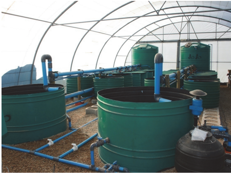
Figure 2.11 The aquaculture system with settling tanks in the foreground, the mechanical filter at the front right, the fish grow-out tanks in the middle and the biological filters at the back (Photo: Rory Scheepers).
