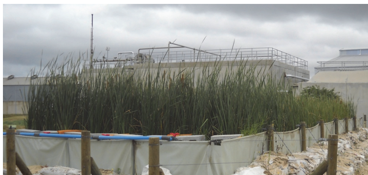
Figure 2.8 The constructed wetland (Photo: Rory Scheepers).
