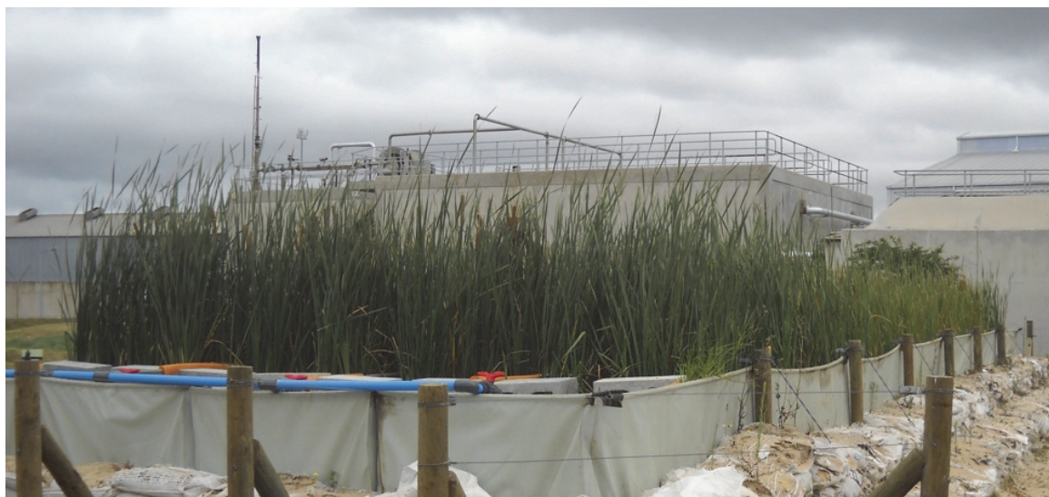
Figure 2 The constructed wetland used to treat brewery effluent subject to various pre-treatment processes (Photo: Rory Scheepers).
