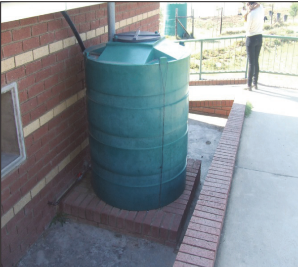
Rainwater Harvesting Tank
