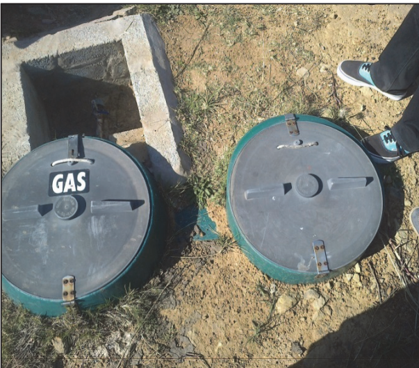
Biogas 'In' and 'Out' Tanks
