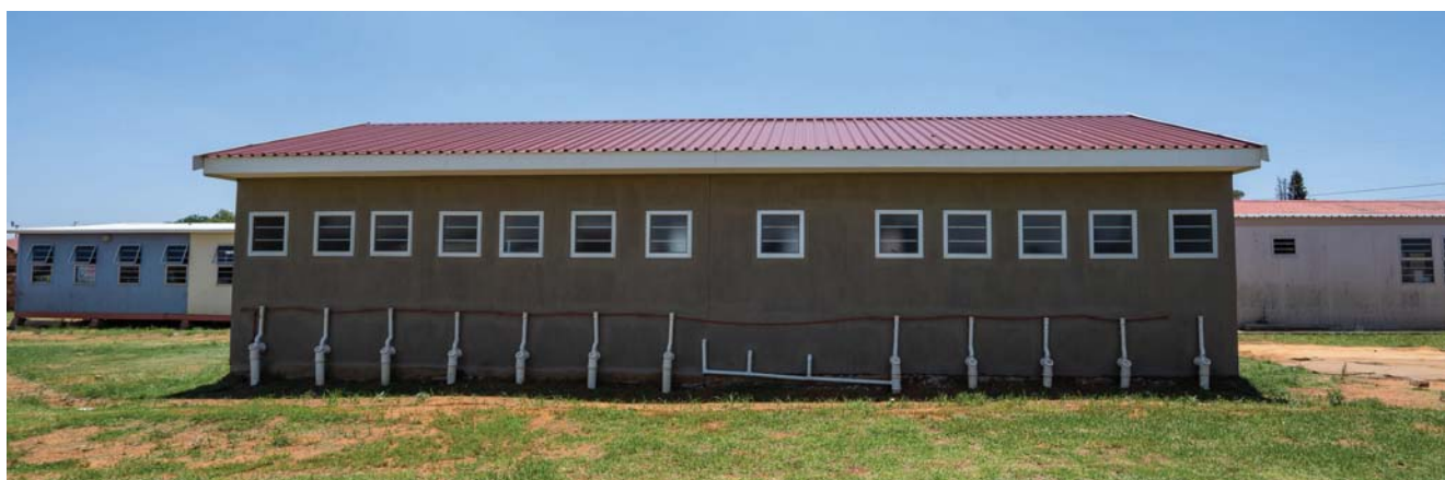
The outside of the new ablution block. Wastewater is gravity-fed to holding tanks before being treated in the on-site treatment system.
