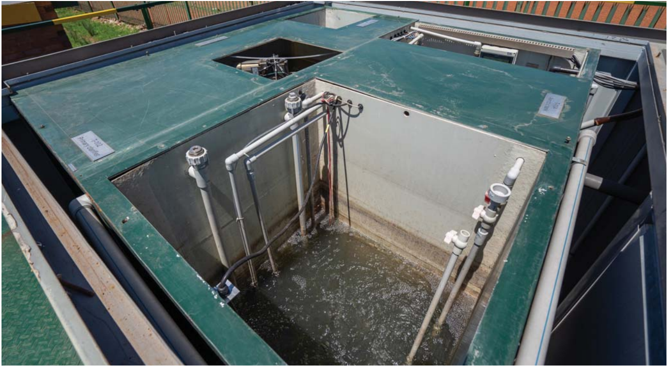
The Clear TT-5 containerised four toilet seat front and backend treatment plant abluion facility.
