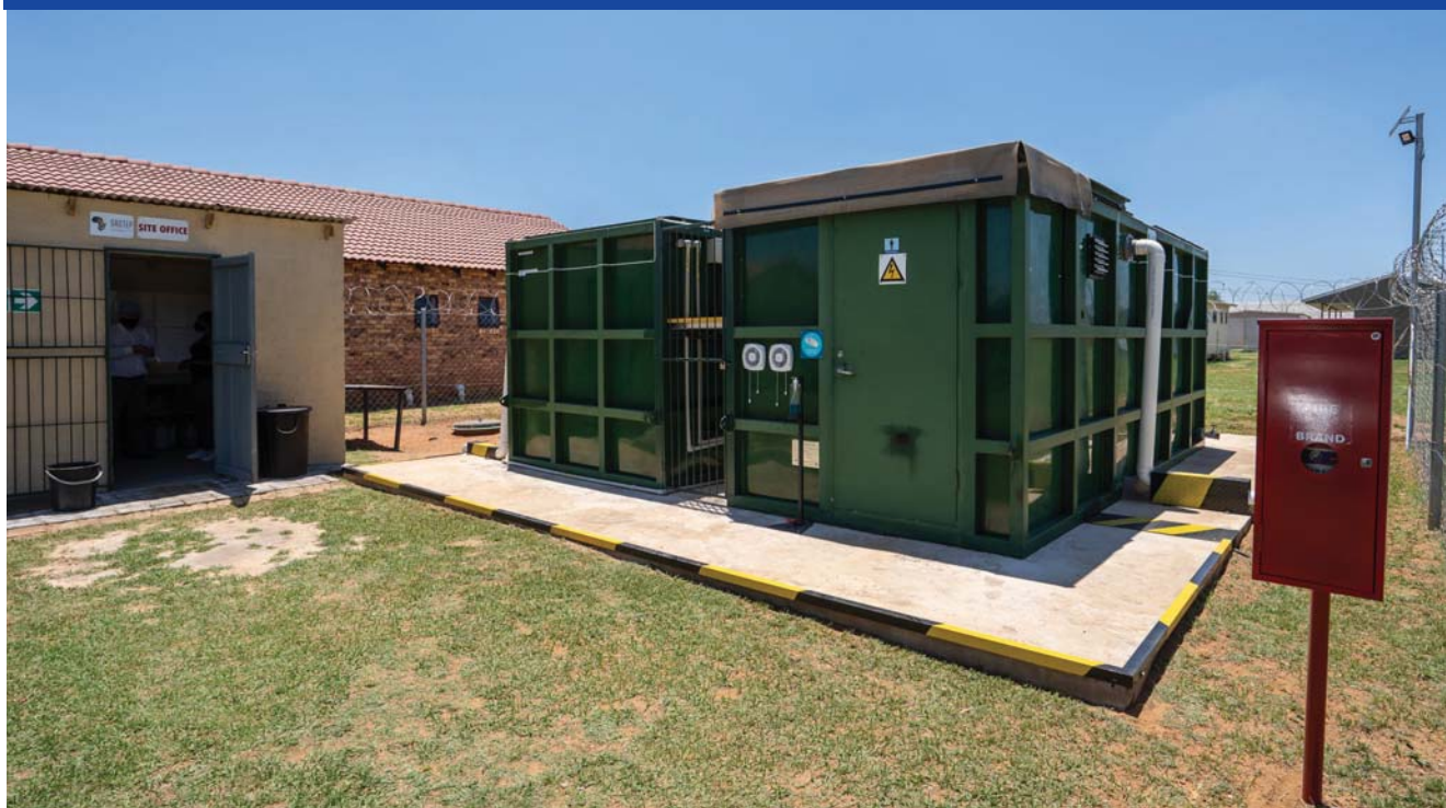
The containerised treatment unit treats wastewater on site for reuse. The treated water is recirculated for flushing.
