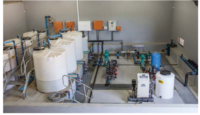
Part of the new system includes that all valves fertilizer is moved to a central pump house.
