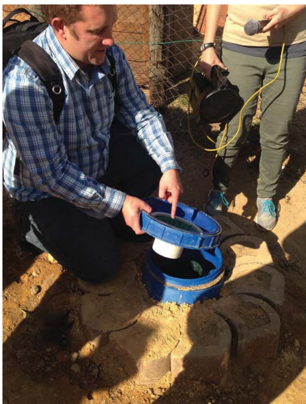
One of the greywater disposal points in Langrug settlement.
