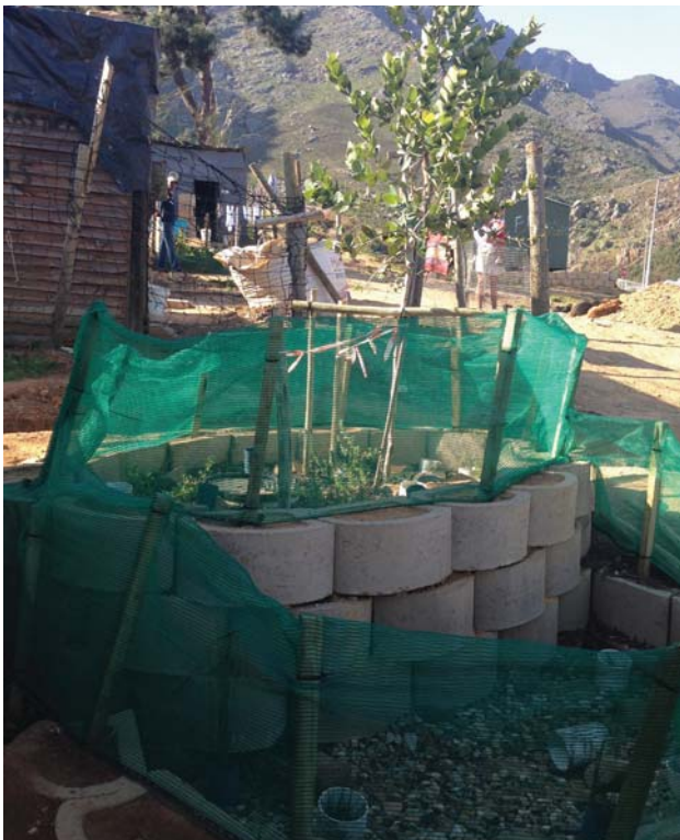
Tree pits just after installation at Langrug informal settlement. In a couple of decades these will be an outstanding feature of the settlement landscape, while still serving as a wastewater management system.
