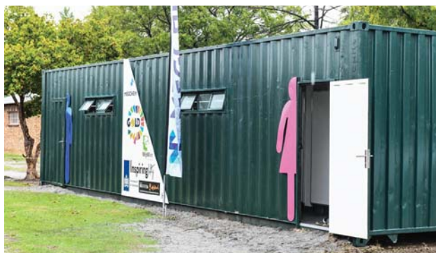
The containerised gender-neutral waterless urinal facility installed at the Osizweni Primary School in Embalehle, Mpumalanga.
