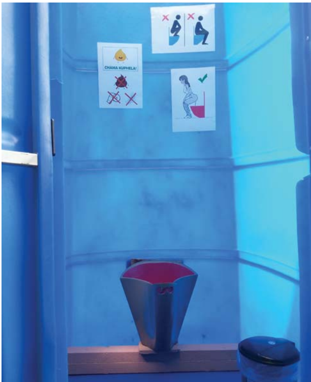
The toilet huts contained a Weestand urinal – a roll of toilet paper and a bin for disposal of used paper as well as signage to ensure learners used the urinals correctly.
