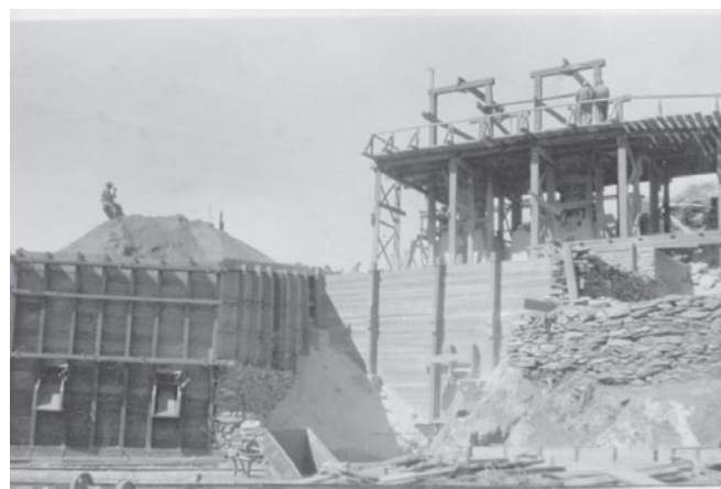
The sand and rock mixers on site in the early 1930s.
