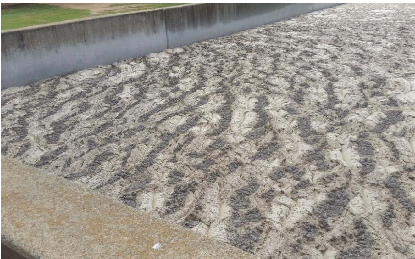
Sludge bulking in an activated sludge reactor
