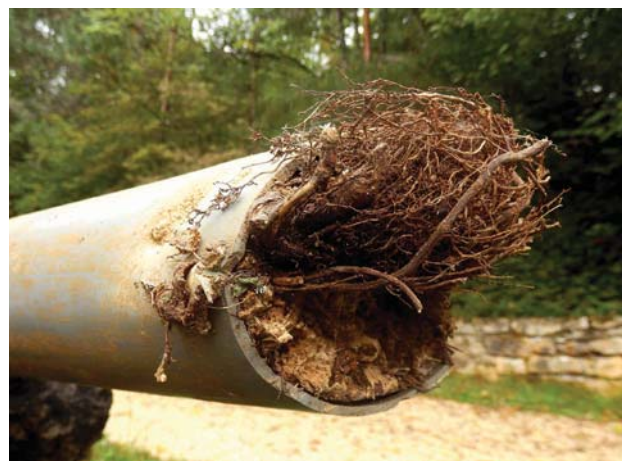
Tree roots blocking a sewer pipe.
