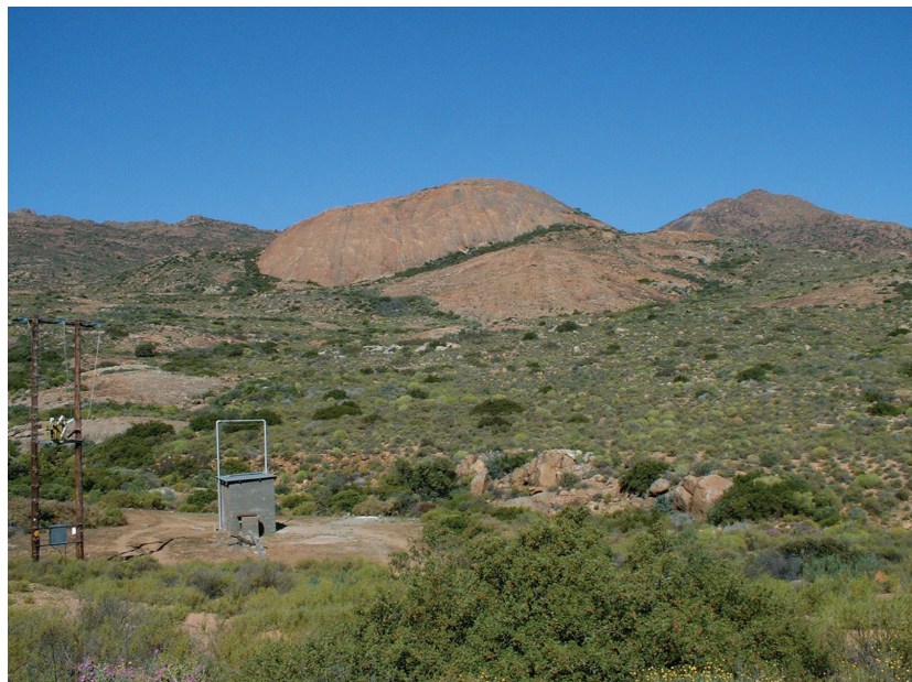
The pump house of the abstraction borehole is surrounded by granite outcrops.
