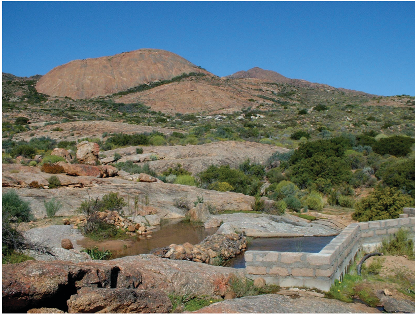
The simple sand filter in the bed of the river, which flows through a valley carved from granite.
