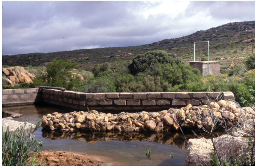
The sand filter where river water is filtered before it gravitates into the injection borehole. In the background is the pump house of the abstraction borehole.
