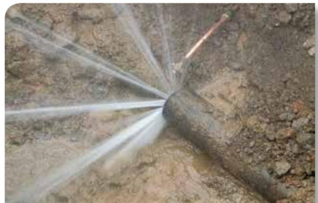
Figure 6: Underground leak running at high pressure (Ken Brothers)
