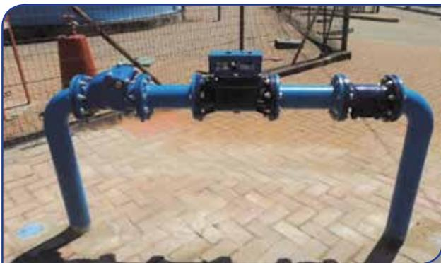
Figure 11: Typical bulk industrial consumer meter in Ekurhuleni
