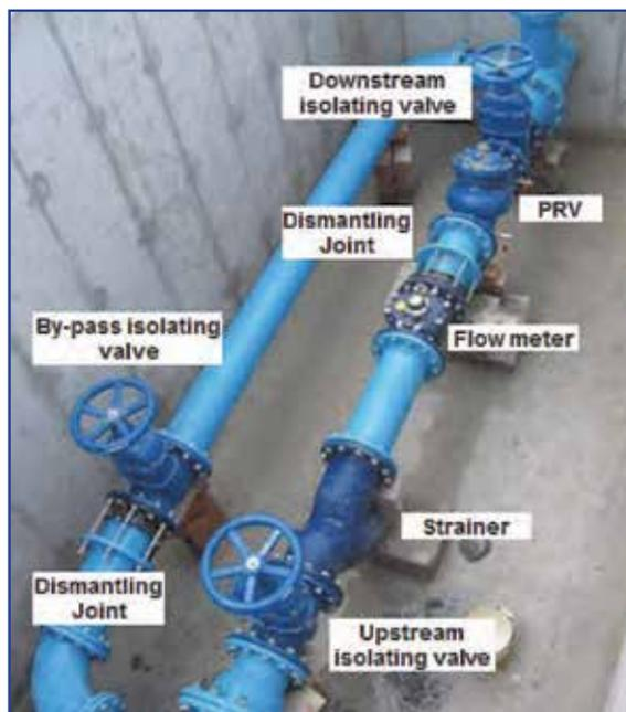
Figure 9: Typical bulk management meter in pressure reducing valve (PRV) chamber
