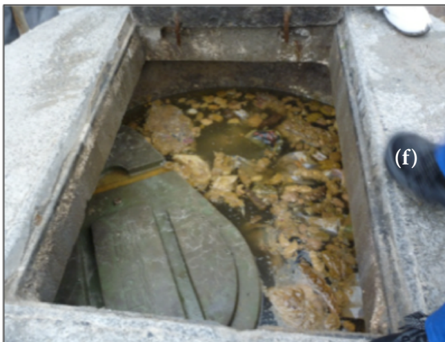
Photos of Kosovo's vacuum system and connected toilets. From the top: (a) raw sewage overflow from washbasin drain in June 2009, (b) attempts by residents to prevent spillage by covering drains with wooden boards in June 2009, (c) a used but disconnected toilet in November 2010, (d) a spoon piercing an interface valve diaphragm, (e) a brick in a sump, (f) a submerged collection chamber in a flooded concrete ring in June 2010 and (g) destroyed toilets in July 2010
