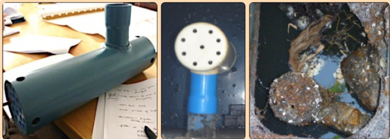
The 63 mm outlet filter (left) that is installed in Hermanus' properties. The middle photo is of a filter on a new tank that was just commissioned and the photo on the right is of a settled tank that has been in operation for several years (Photos by Ashipala (2010) and Taing (2012)).
