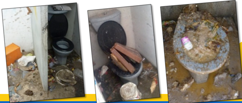
Evidence of greywater, food waste and solid waste disposal in Kosovo toilets connected to the vacuum sewer (Photos by Taing, 2010, 2011).
