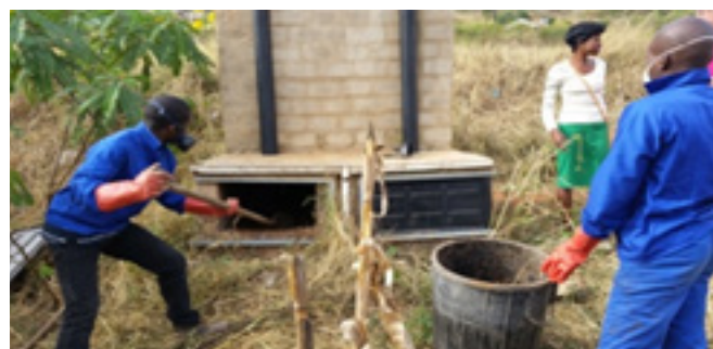
Emptying faecal sludge from a Urine Diversion Toilet
