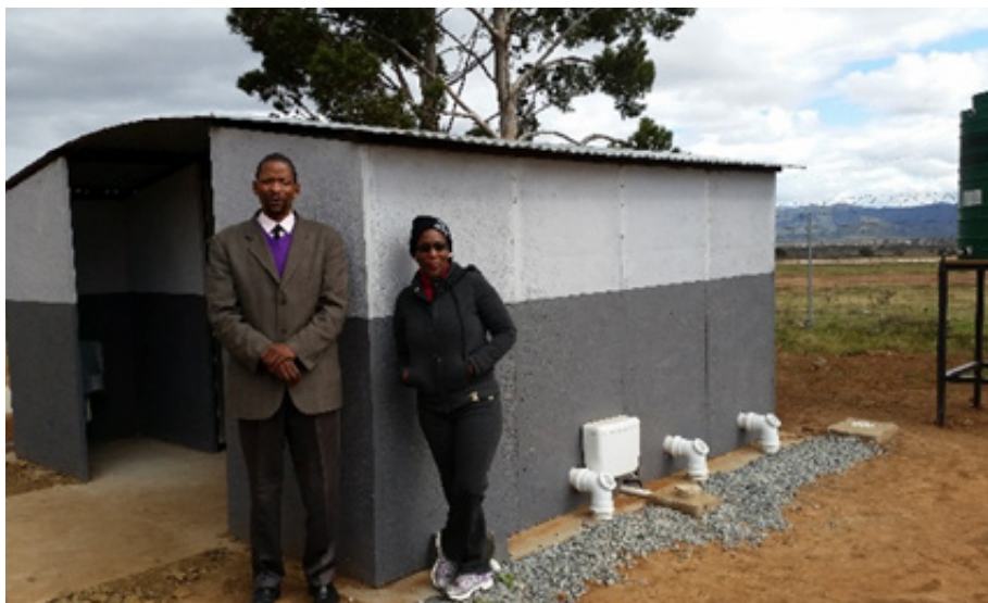
Facility built for schools housing the pour/low flush units.
