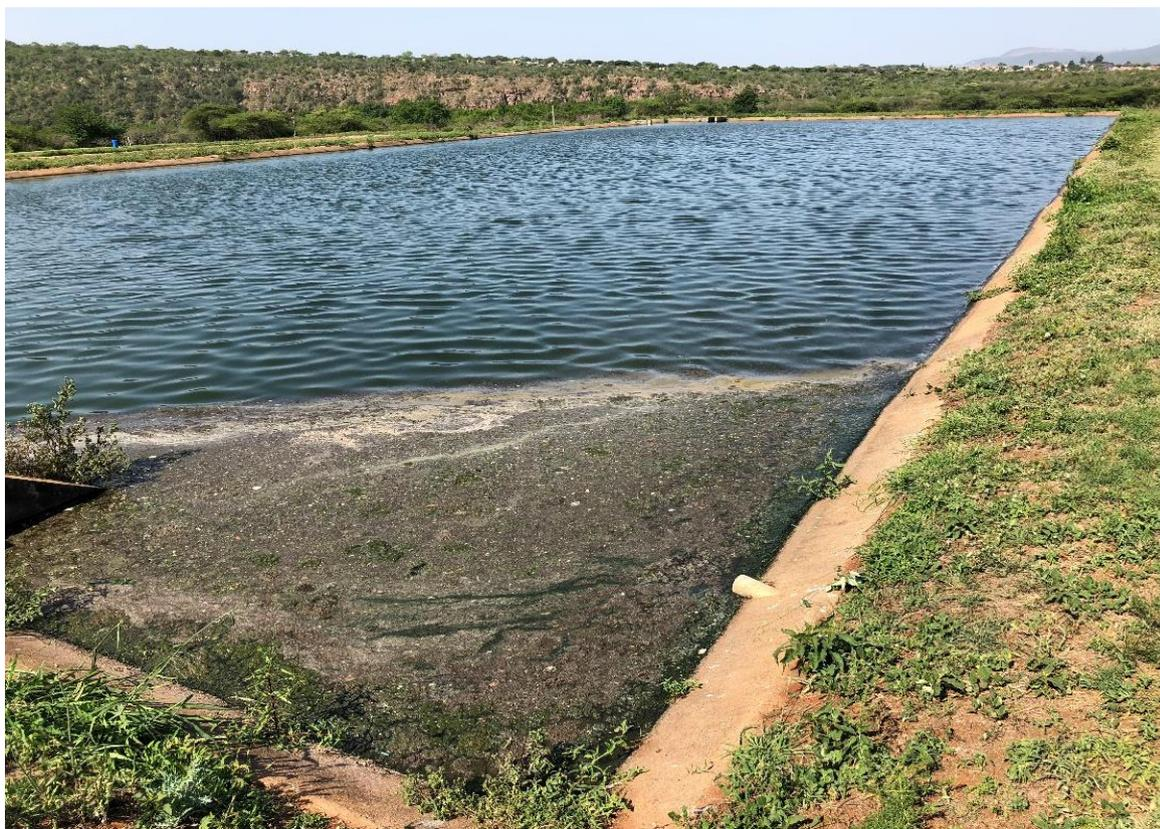
**Figure 6: Ulundi Ponds showing sludge**
