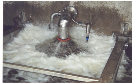
300 DIAM DV AS MANUAL VALVE FOR LARGE AUTOMATIC SCOUR GATE
