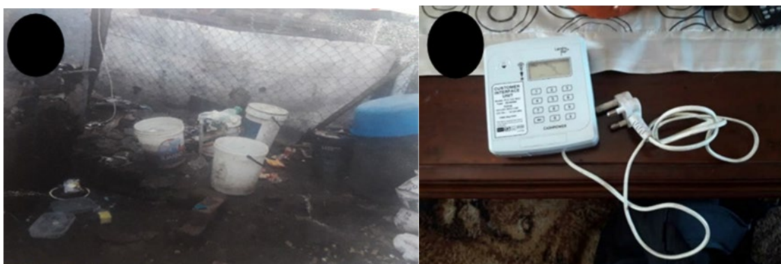
Figure 72 Left: electricity wire connected from outside the house. Right: external device used to recharge electricity pin on the meter box.
