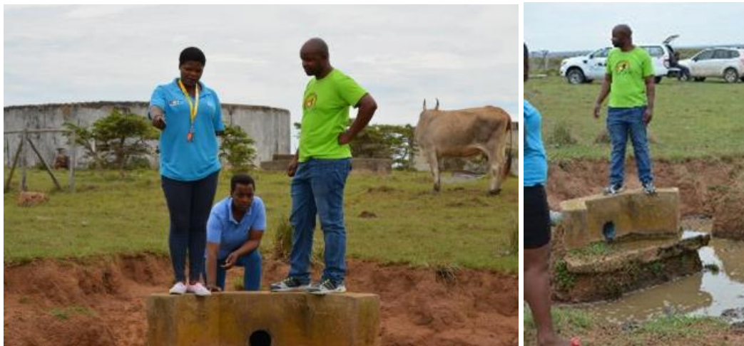
Figure 52 CRAs visit the Hamburg water reservoirs and inspect a cattle 'watering hole' created by a leak in the overflow pipe.
