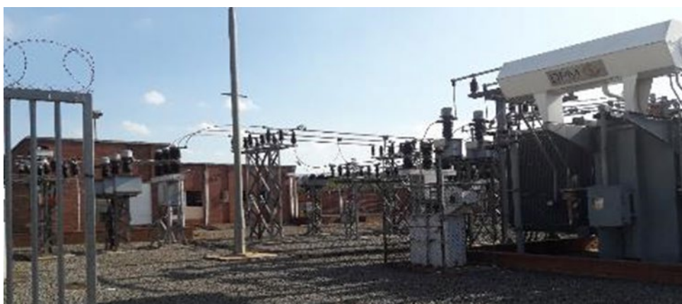
Figure 63 One of the electricity sub-stations visited in the uMngeni catchment. This is the point at which ESKOM supplies the municipality with electricity and the municipality then distributes it to consumers in the municipal area via its own distribution network.
