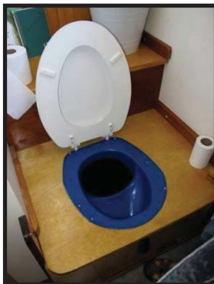
Figure 21. A typical urine separating toilet
