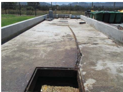
Figure 15: Septic tank
