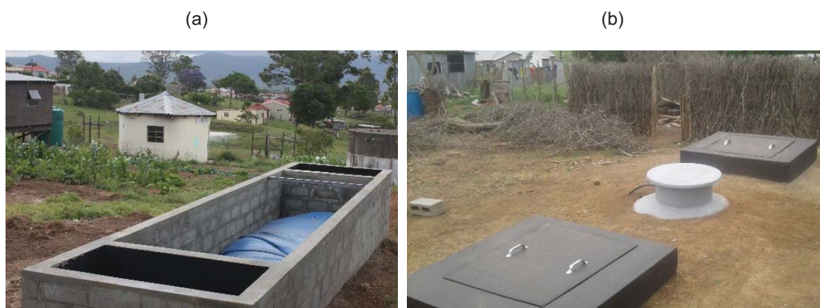
Figure 3.11: Two types of digesters installed in the two villages: (a) balloon; and (b) fixed-dome digesters
