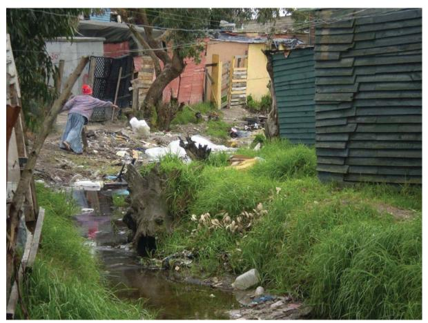
Figure 3.2 An example of a drainage channel being used as a conduit for solid waste in Masiphumelele settlement, Cape Town (photo: N. Armitage)
