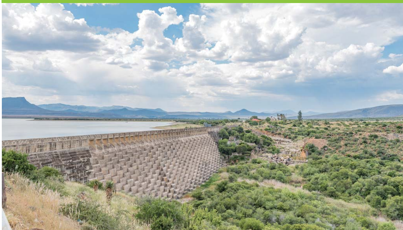
The fine material that fills Nqweba Dam has a high silt (40%) and clay (55%) content making it tricky to work with.
