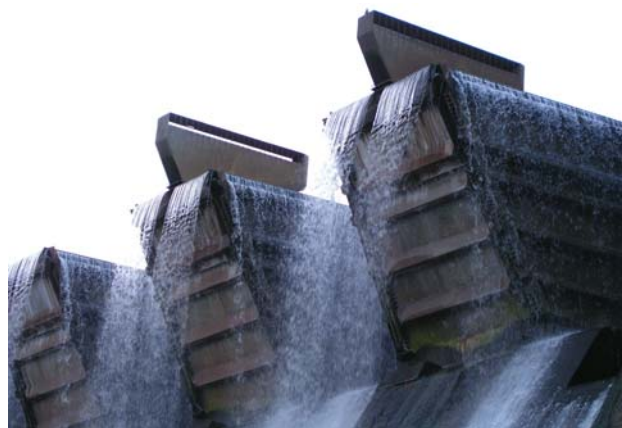
A close up of the fuse gates, which were added to the wall in 1994.
