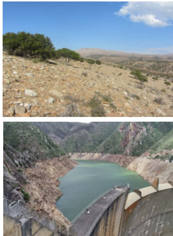
Figure 2: (top) Dry slopes with little to no plant cover in the Baviaanskloof (Source: Luyanda Luthuli) and (bottom) the Kouga dam at 14% full on 26 November 2021 (source: https://www.facebook.com/gamtoosirrigationboard )
