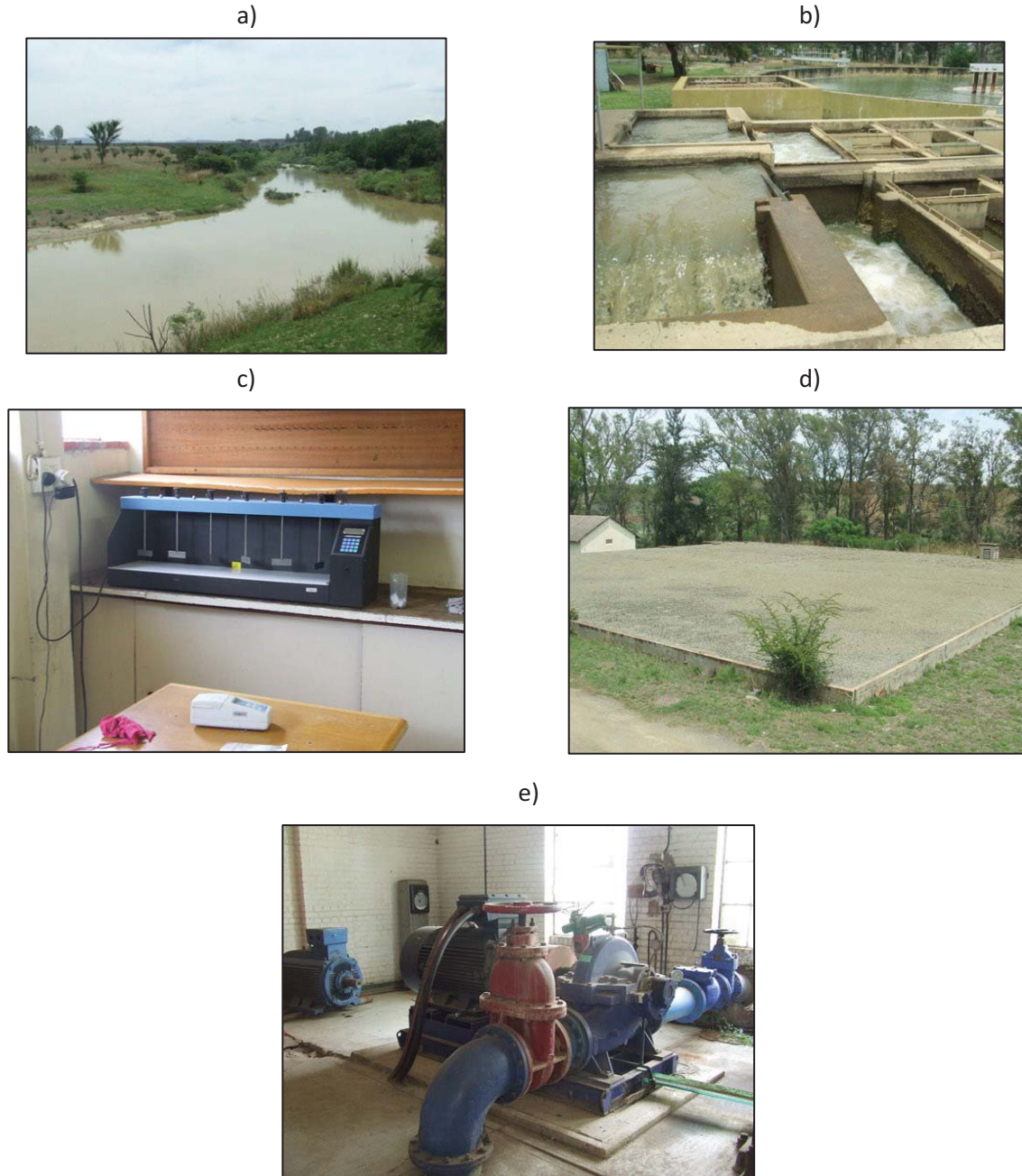
Figure 47: Components of the Ladysmith water supply inspected during the site visit. The components include a) the source water, b) the water treatment works, c) the onsite laboratory d) the reservoir and e) pump stations
