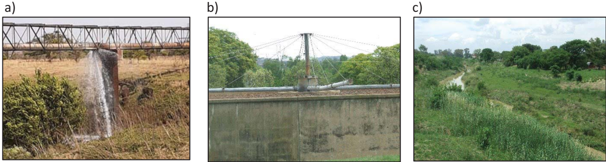
Figure 49: Examples of components within Uthukela that are likely to be impacted by climate threats. In the above figure a) indicates a pipe burst due to poor infrastructure condition, this is likely to worsen during periods of high flows; b) indicates that flows into works negatively impacting on microbiological treatment efficiency of biofilters; c) flows into the works based on drought and impacts need to be managed
