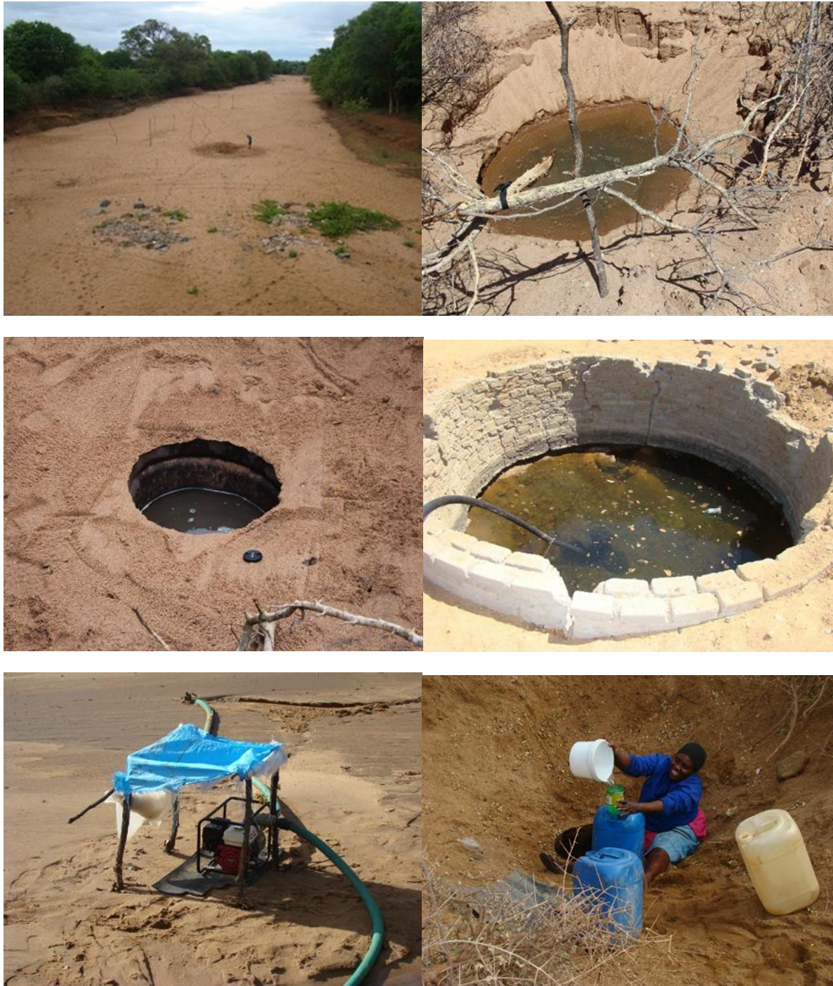
Figure 2.1 Examples of installations for shallow groundwater abstraction from sand river aquifers in the Limpopo Province, South Africa.
