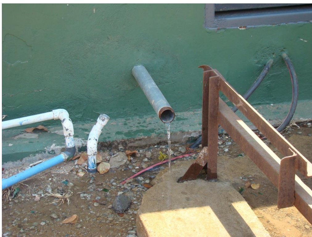
Figure 5.4 Top: Borehole H14-0025 in Matsotso. Bottom: The borehole is operating at low pressure; the pump pressure head needs to be increased.
