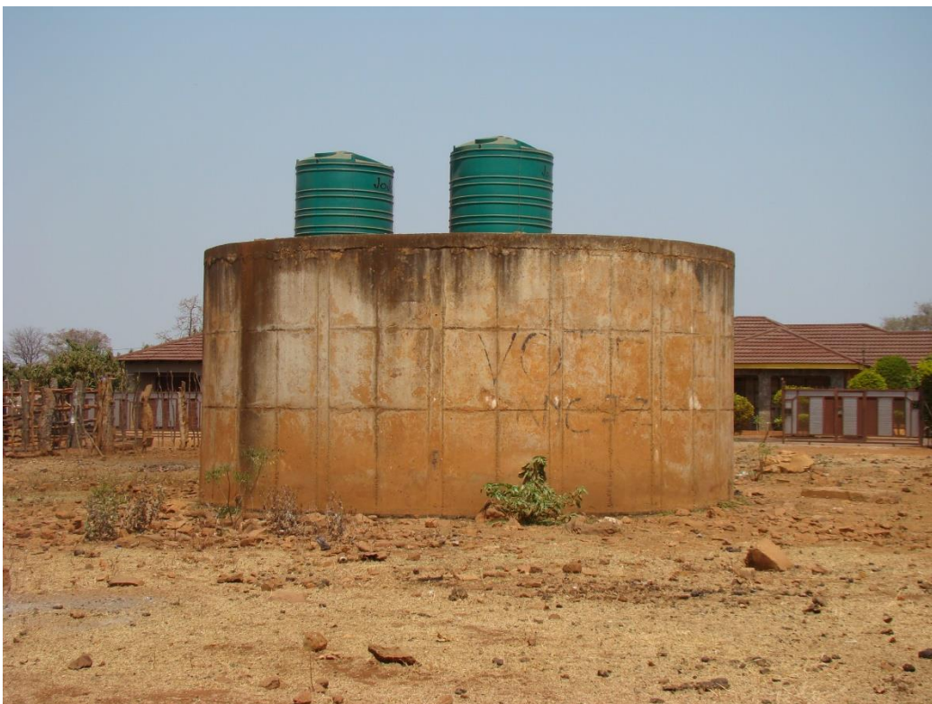
Figure 5.3 Top: Borehole at Mzilela. Bottom: Village reservoir; a booster pump is sufficient to fill tanks; however no diesel is supplied by Municipality to operate it.
