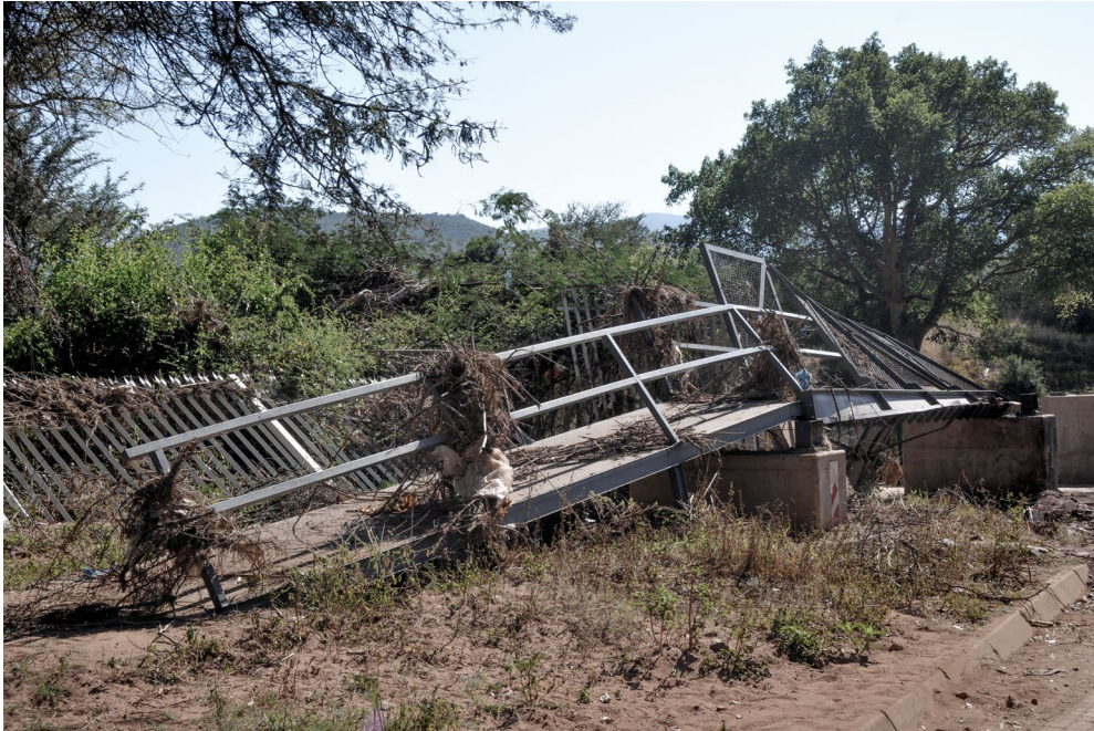
Figure 74. Bridge destroyed during cyclone Eloise in Limpopo
