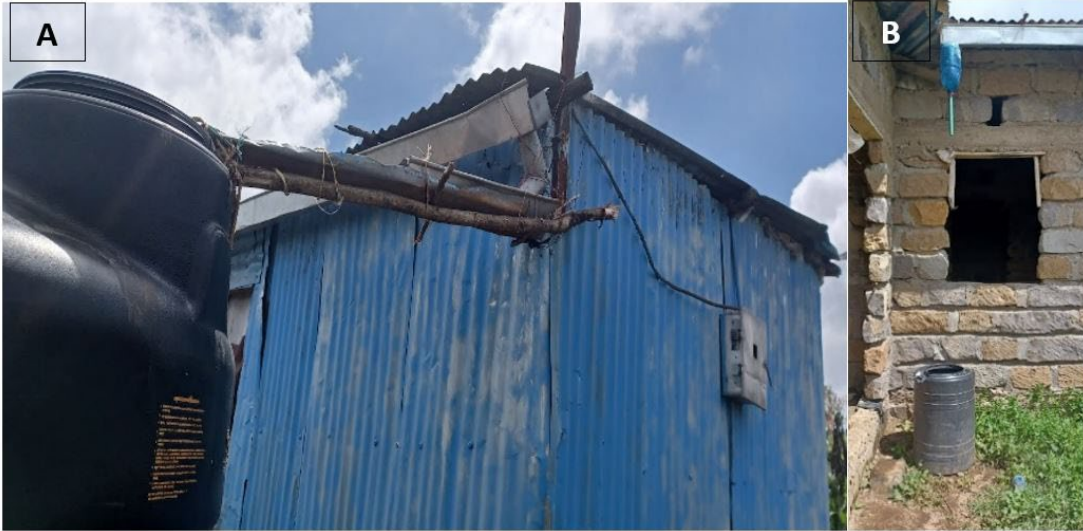
Figure 76. Two examples of water harvesting systems adopted by some households in Narok, Kenya
