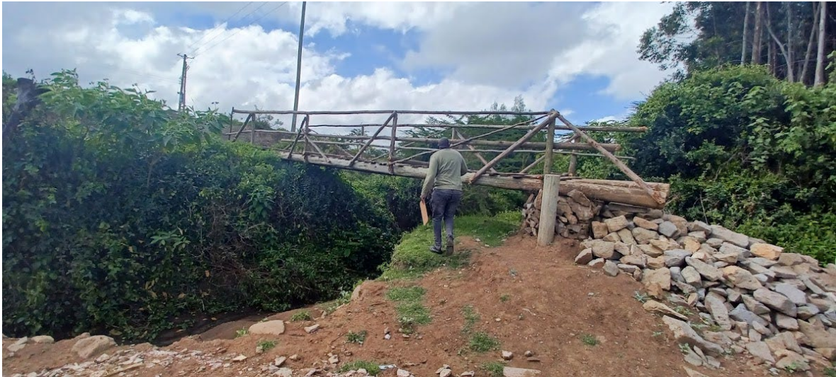
Figure 79. A makeshift bridge constructed by community members when the road was washed of during the floods. The bridge allows communities to cross the river during the rainy season and access homes and grazing lands in the reserve
