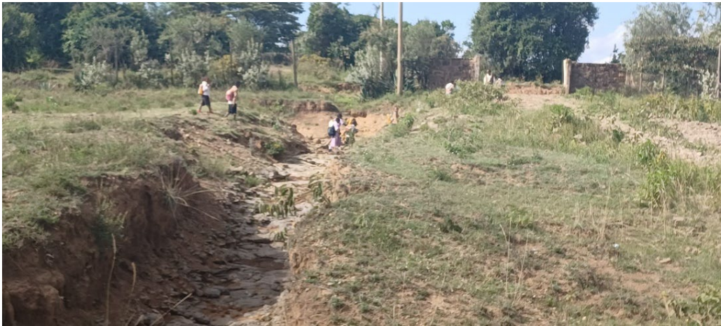
Figure 78. A gully formed during the floods that learners now have to cross to access their school in Narok
