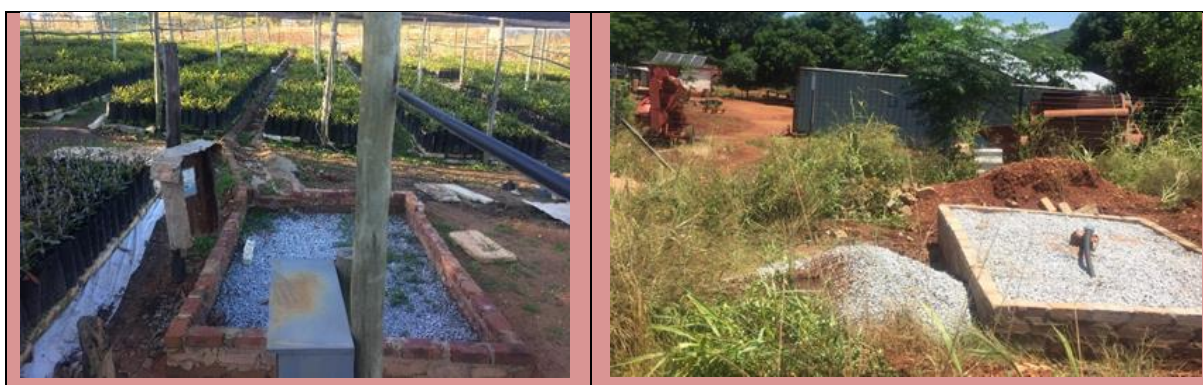
Figure 4.18. Completed filter box or tank and borehole known as Bhungroo
