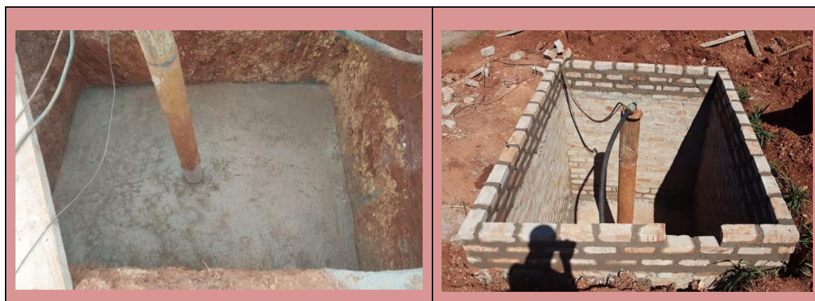
Figure 4.16. Constructed bottom slab and brick walls for the filter box
