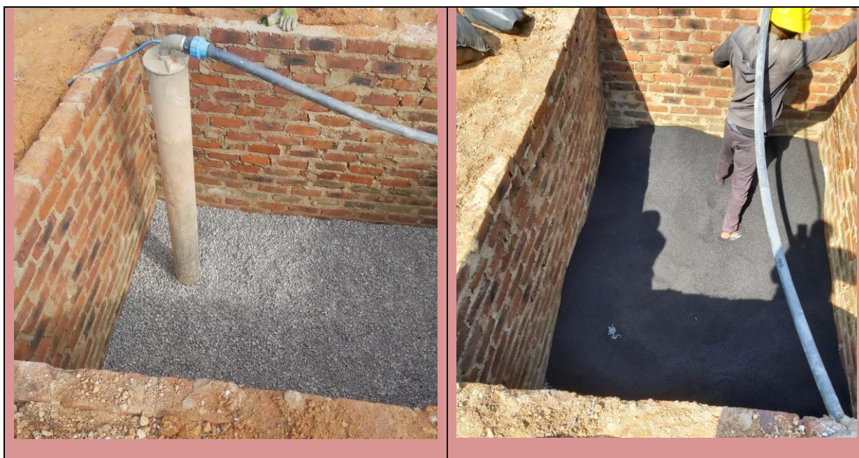
Figure 4.17. Laying of filter material, small stones and activated carbon in the filter box
