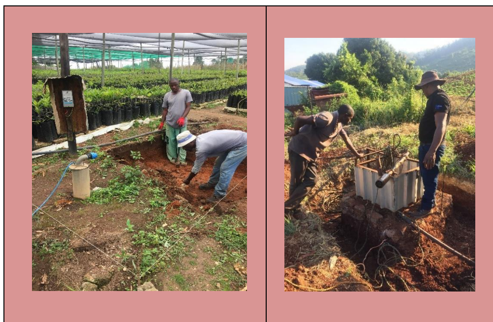
Figure 4.15. Marking the dimensions and manual excavation of the filter box
