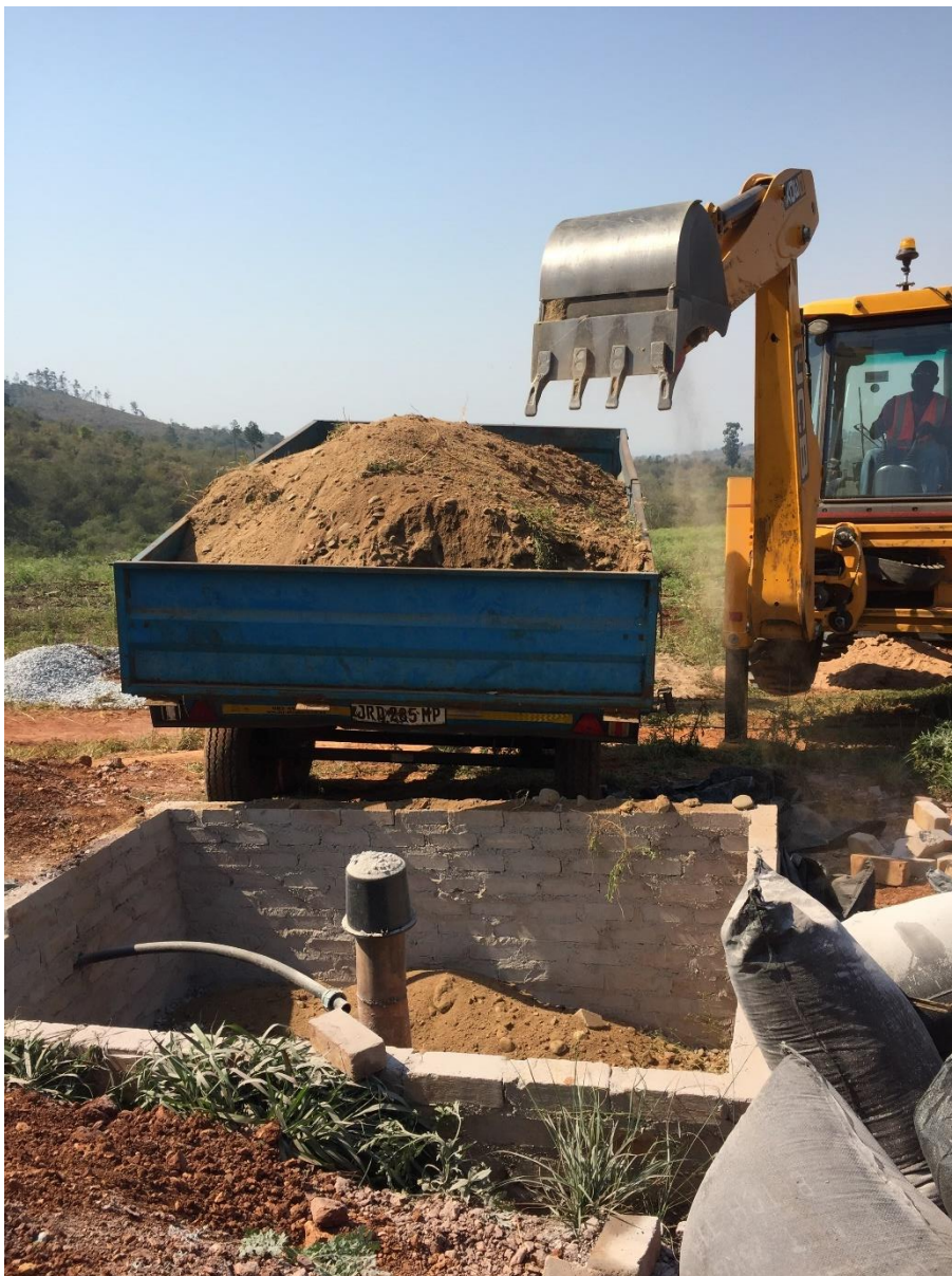
Figure A3: Placing of river sand in the filter box with extended borehole casing at Schoemansdal site
