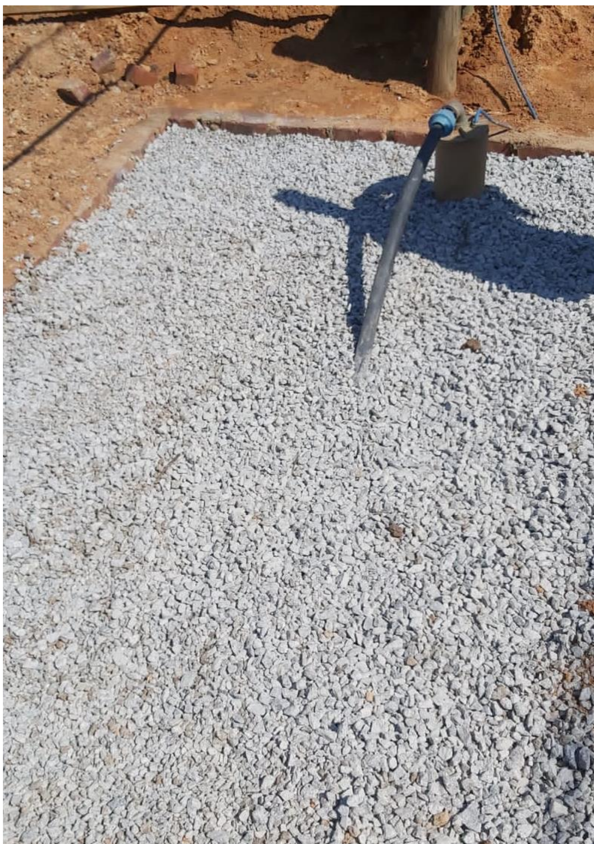
Figure A4: Completed filter box for the Bhungroo borehole at White River site
