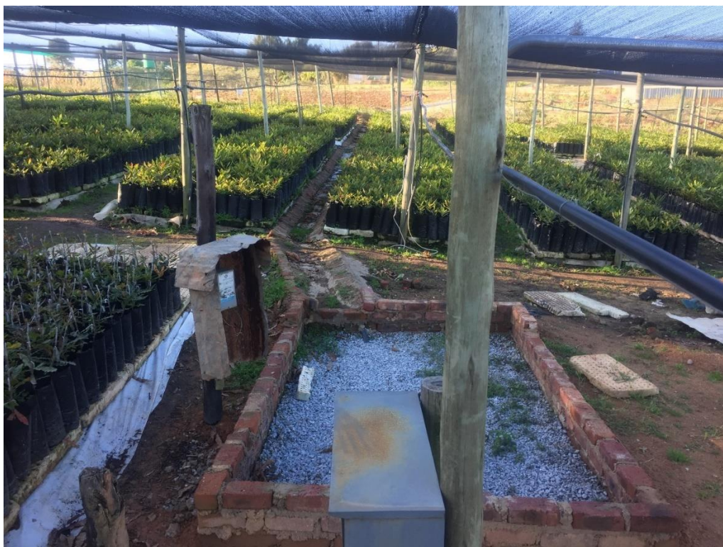
Figure 3.4. Channel harvesting runoff to the Bhungroo filter box at White River site
