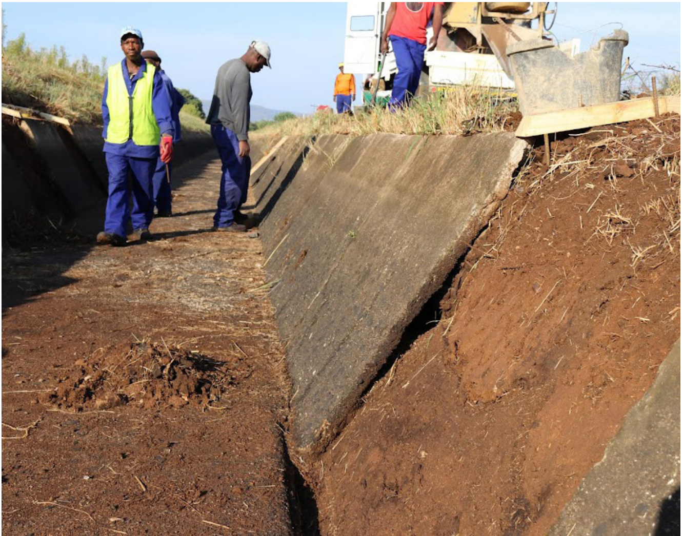
Maintenance workers repair a damaged section of canal at the Loskop irrigation scheme.
