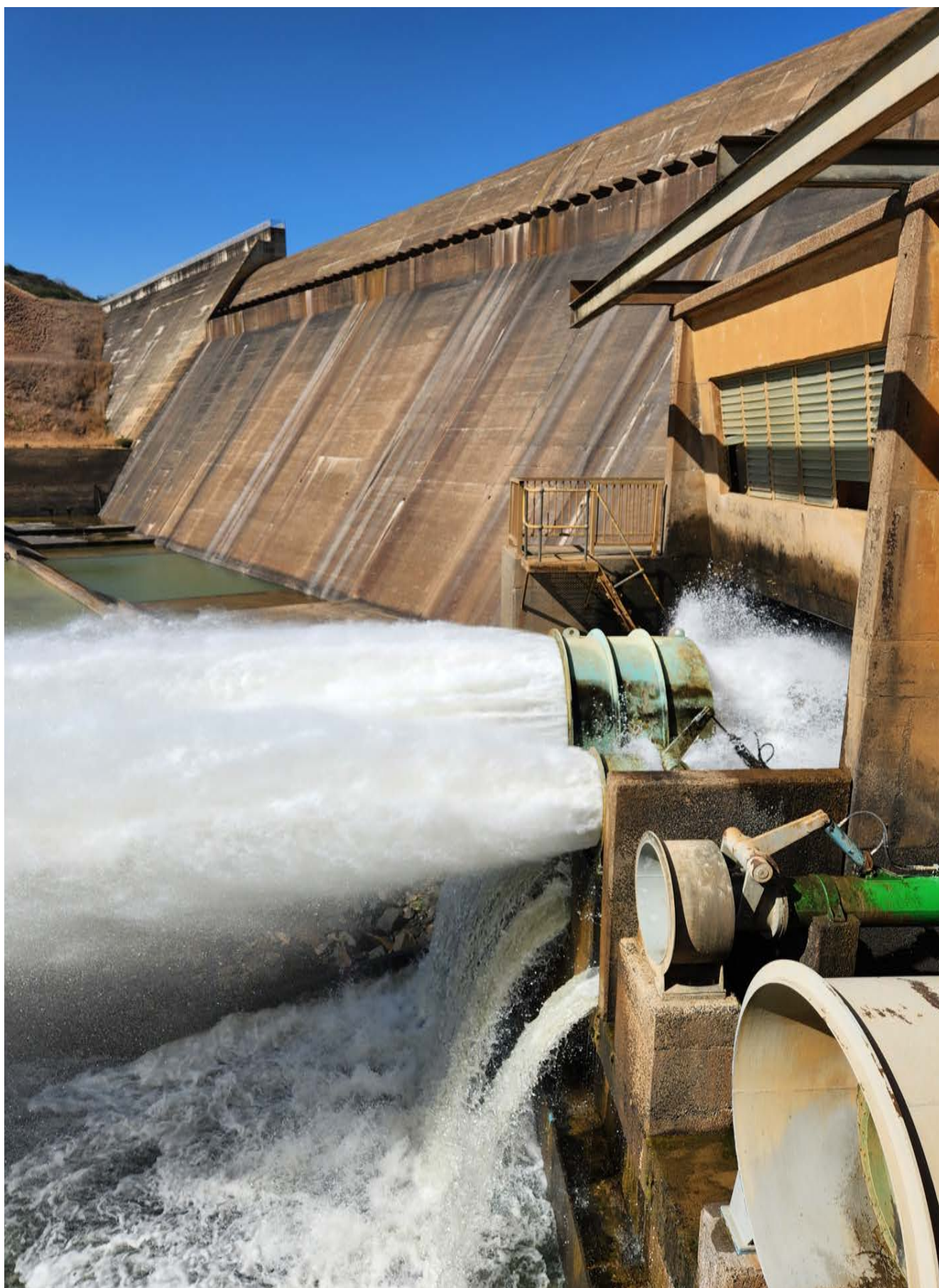
Water exiting the sleeve valve at the Spioenkop Dam outlet, near Winterton in KwaZulu-Natal. There is an opportunity to install a hydropower plant at the dam – and at many other such sites across the country.
