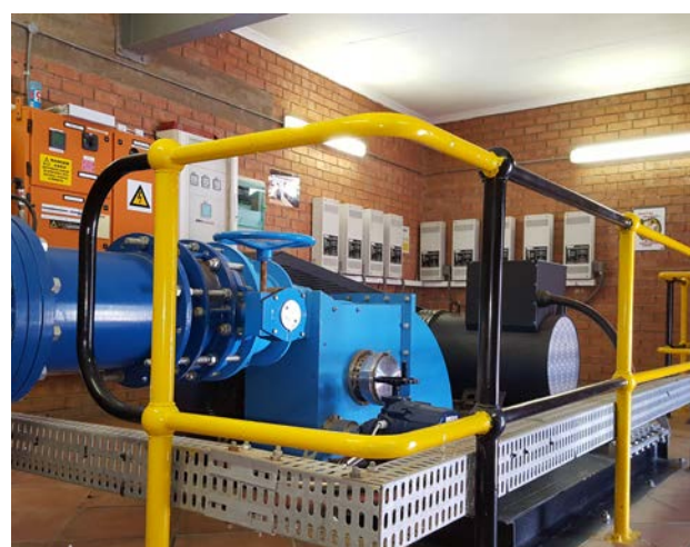
The 96 kW hydropower plant at the Vaal Central Water Board’s (formerly Bloem Water) Brandkop reservoir in Bloemfontein. The plant was installed in 2015 and powers the utilities’ head office.
