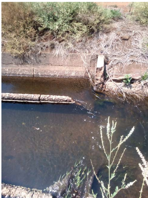
A section of broken wall on one of the canals at the Loskop irrigation scheme. Enormous volumes of water can go to waste if irrigation canals are not maintained properly.
