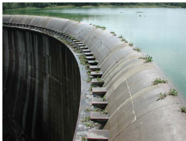
A close up of the Roberts' splitters on the dam wall.
