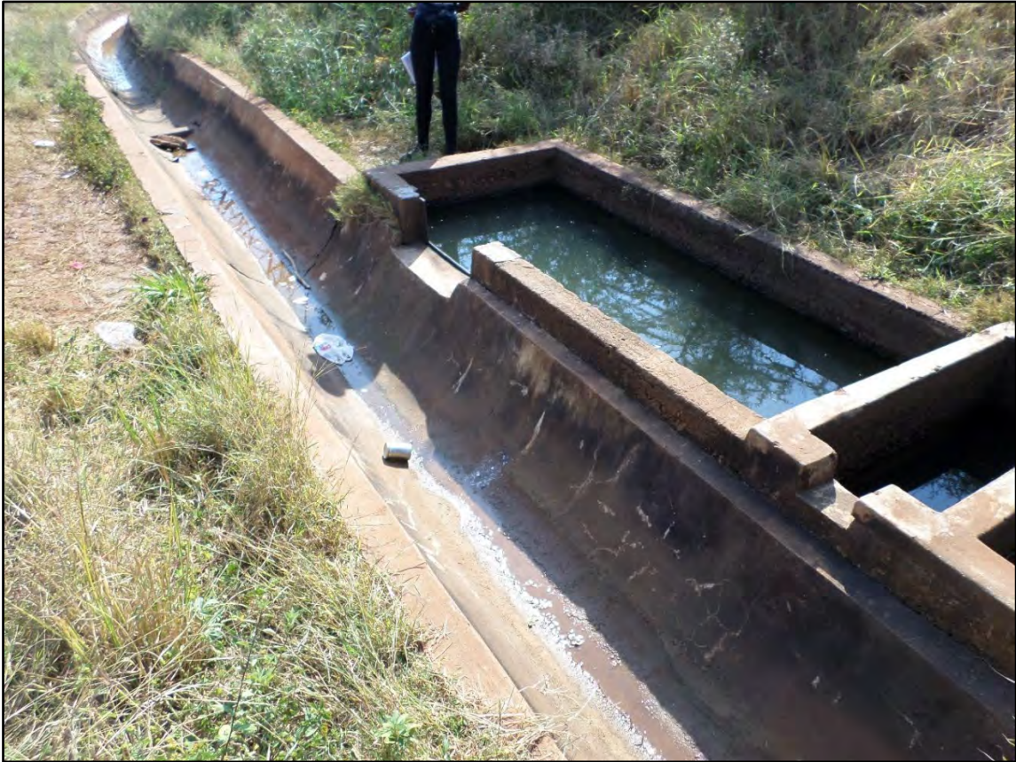
Figure 3.44: Mamuhohi outlet valve stilling basin and overflow
