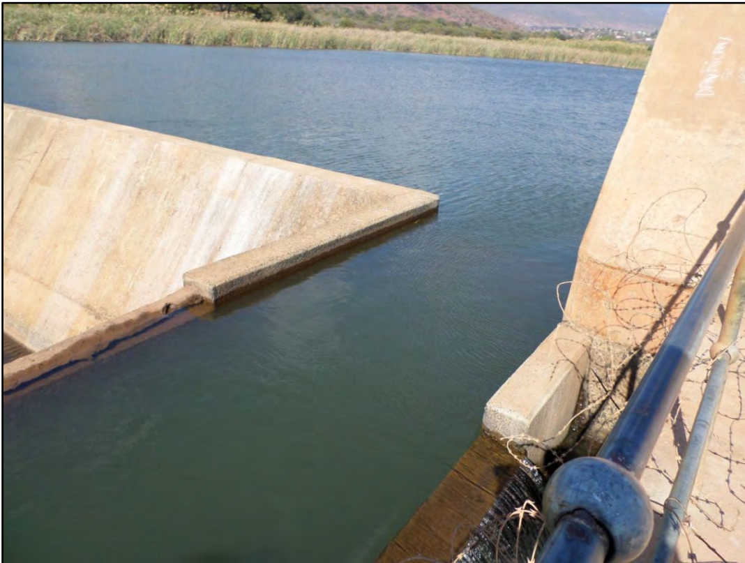
Figure 3.12: Scour channel and overflow into intake chamber at Raliphaswa
