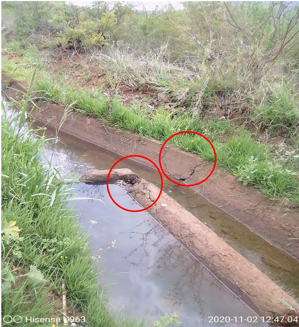
Figure 5.19: Structural damage to main canal at Mandiwana
