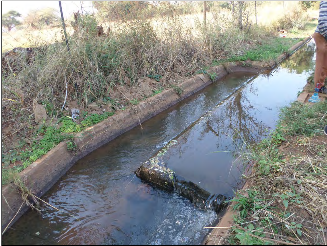
Figure 4.16 Typical L- shaped long weir at the study scheme
