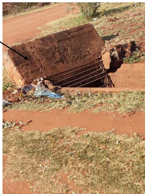
Figure 5.23: Deposition in canal at entrance of Mamuhohi irrigation scheme and collapsed structural member of crossover bridge to night storage dam
