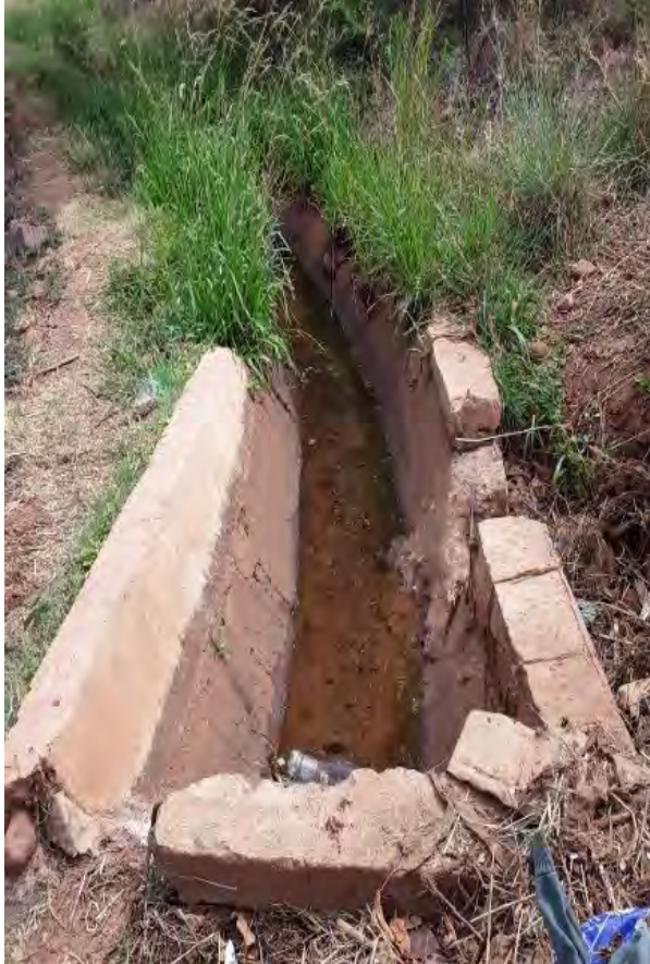
Figure 5.15: Main canal at inlet to underground pipe
