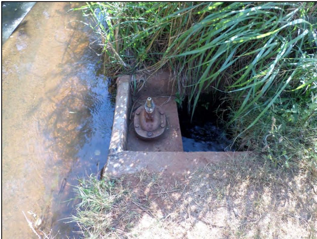
Figure 3.20: Silted long weir and typical offtake at Raliphaswa
