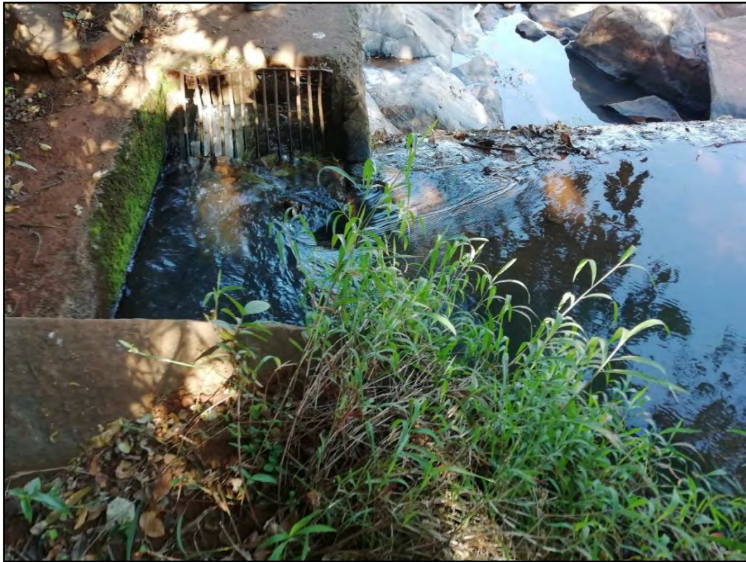
Figure 3.3: Upstream view of Dzindi river intake with trash screen
