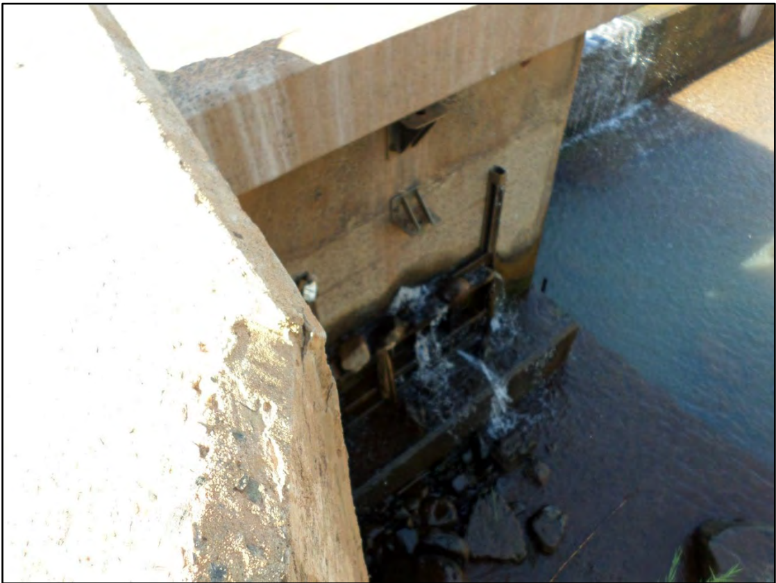
Figure 3.61: Leaking sluice gate from scour channel at Mphephu
