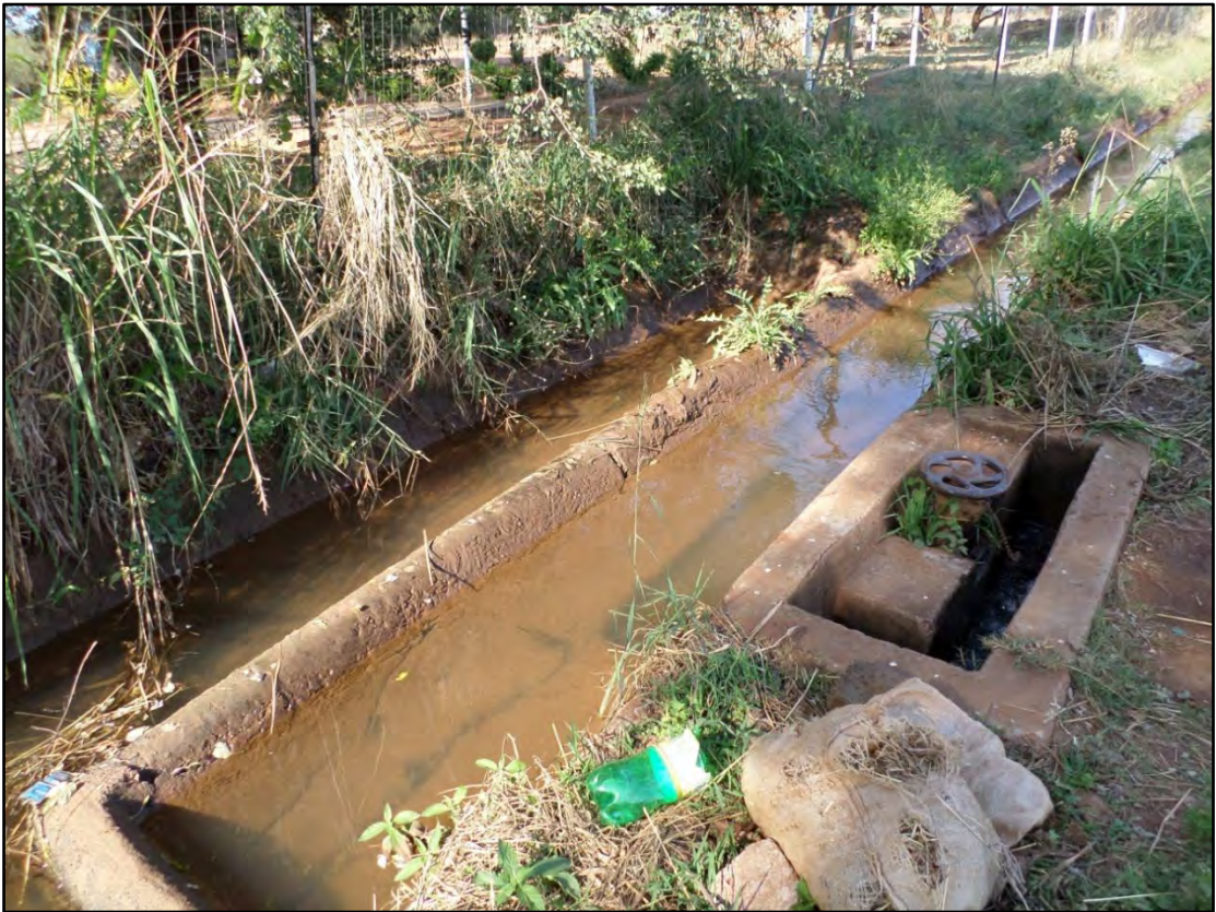
Figure 3.35: Last long weir structure and offtake at Mandiwana
