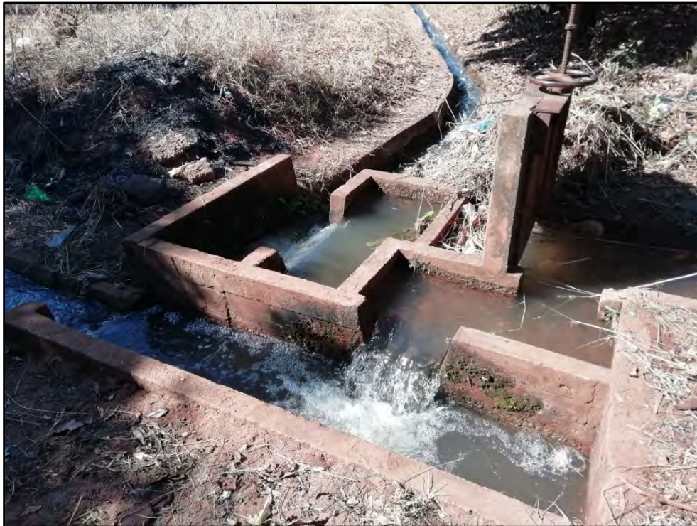
Figure 3.9: Typical bifurcation structure at Dzindi
