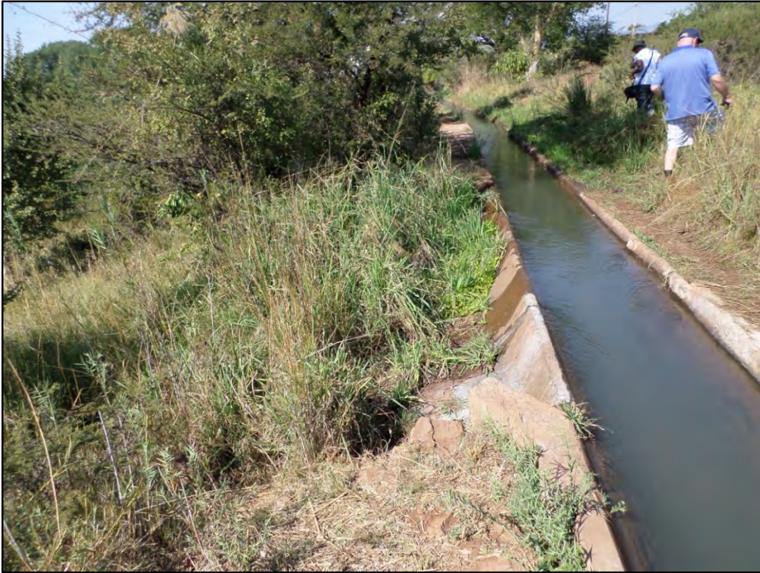
Figure 3.52: Rabali canal reject (overflow structure).
