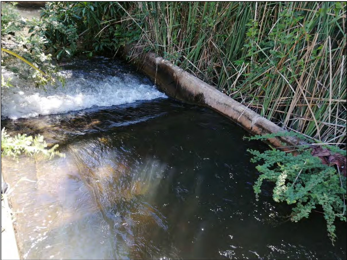
Figure 6.5: Hydraulic jump downstream of crump weir at Raliphaswa SIS
