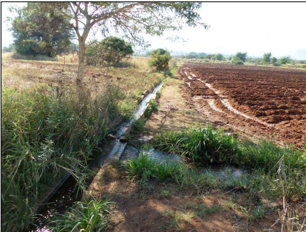
Figure 3.22: Typical concrete main furrow at Raliphaswa
