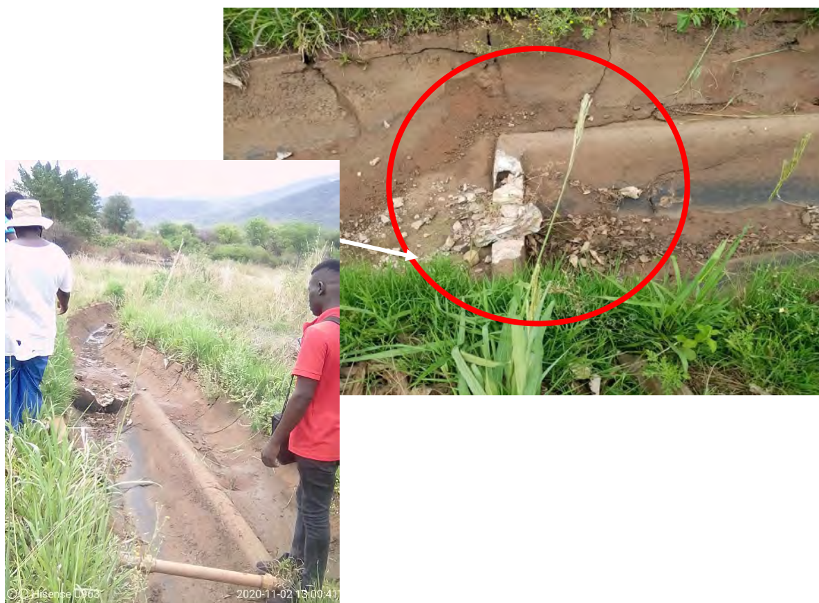
Figure 5.35 Example of vandalised dry main canal at Mandiwana irrigation scheme
