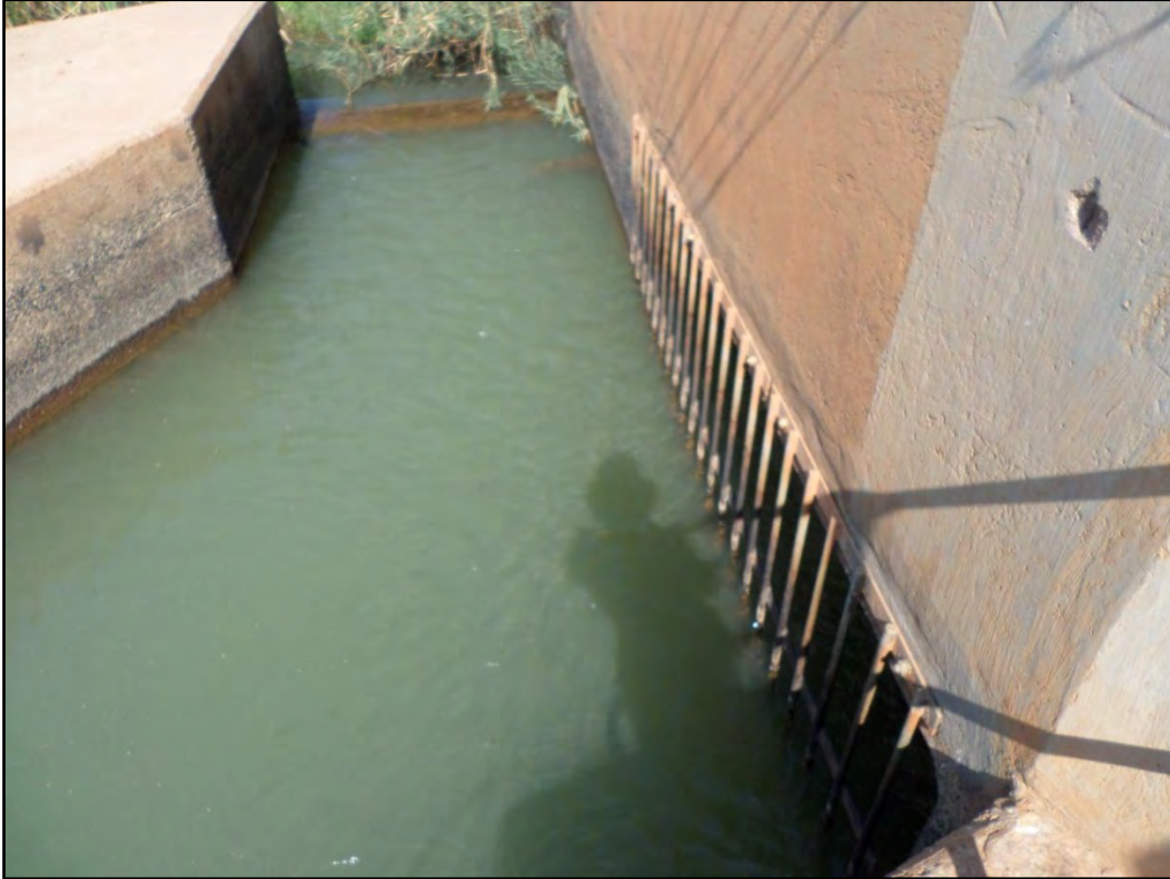
Figure 3.49: Intake into scour channel and trash screens at Rabali
