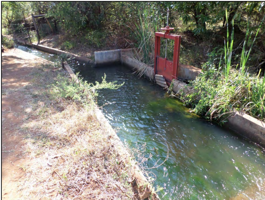
Figure 3.17: Sluice gate reject and reduction to scheme main channel at Raliphaswa
