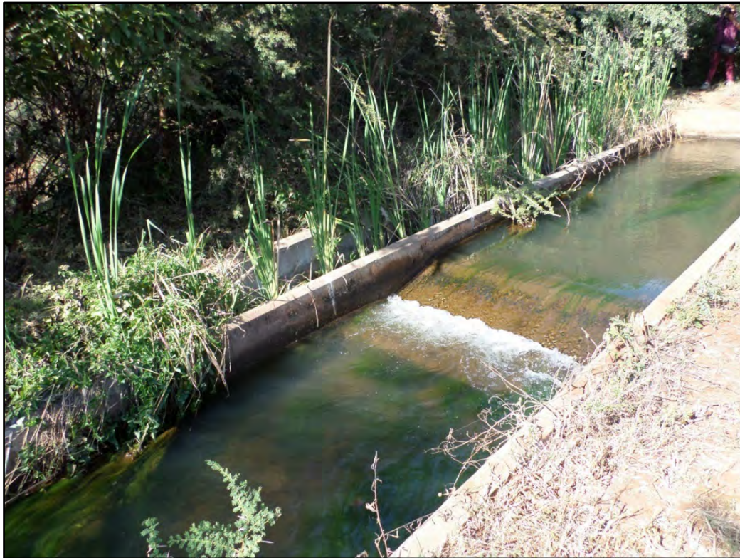
Figure 3.16: Intake pipe outlet and crump weir gauging structure at Raliphaswa
