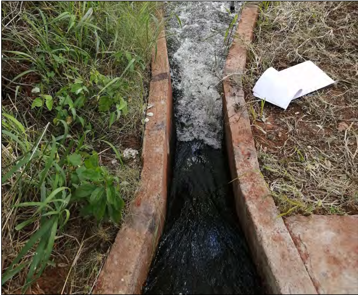
Figure 6.6: Hydraulic jump downstream of Parshall flume.
