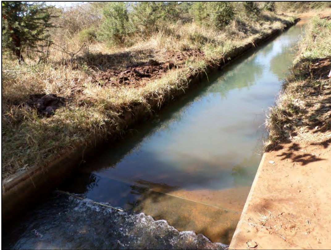
Figure 3.64: Crump weir flow gauging structure at Mphephu
