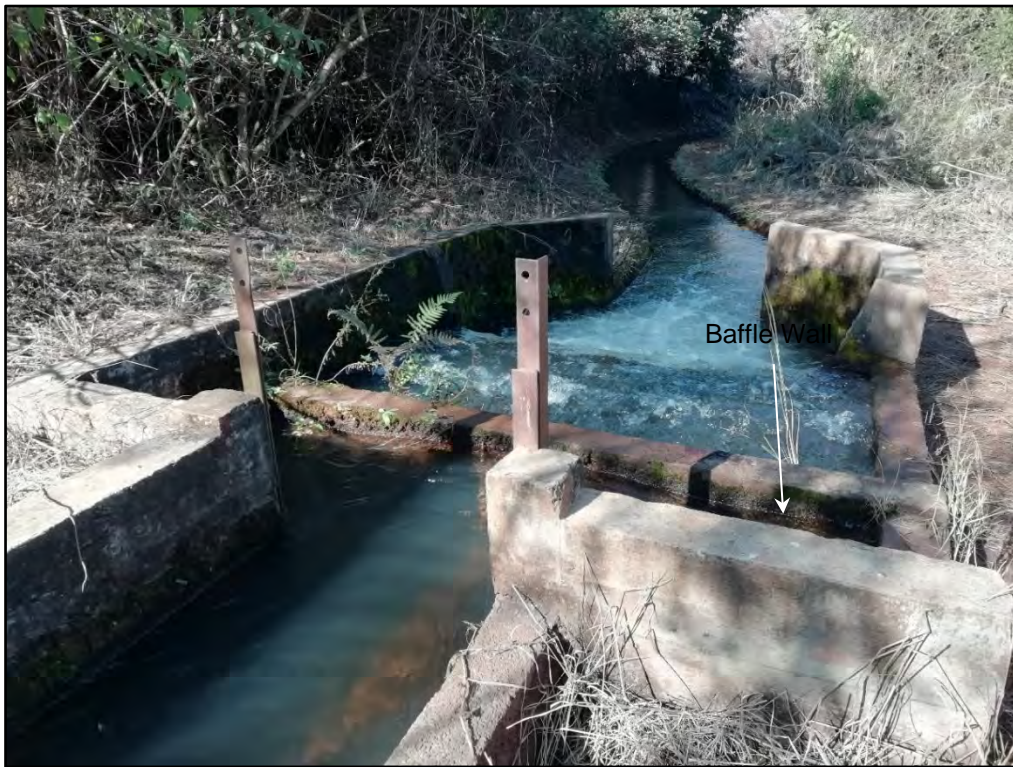
Figure 3.5: Downstream view of Dzindi intake channel exit, impact stilling basin and (Cipolletti) sharp crested weir
