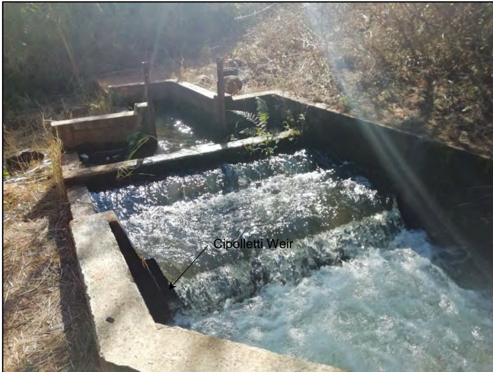
Figure 3.6: Upstream view of Dzindi intake channel exit, impact stilling basin and trapezoidal (Cipolletti) sharp crested weir
