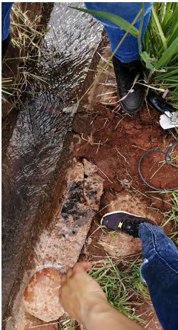
Figure 5.33 Broken canal to divert water to field (plot)
