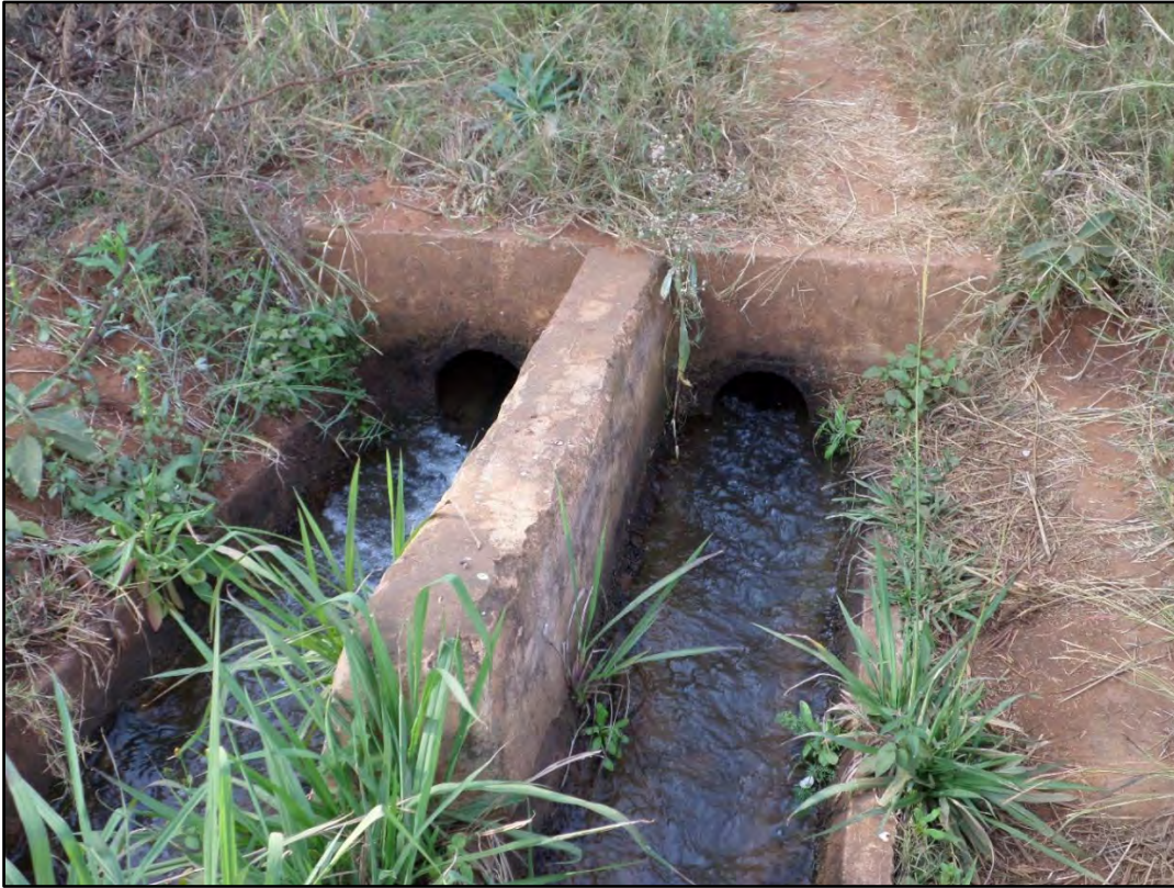
Figure 3.38: Main concrete furrow split after the offtake structure at Mandiwana
