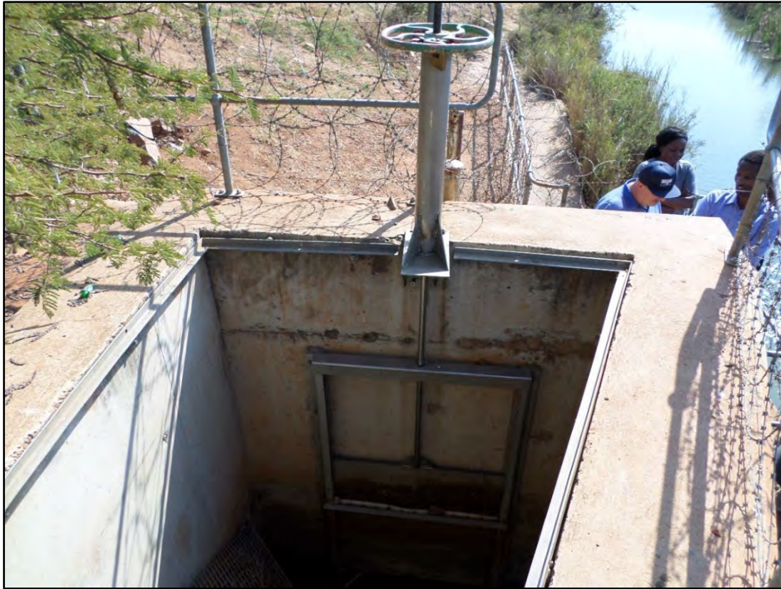
Figure 3.51: Intake chamber and sluice gate at Rabali
