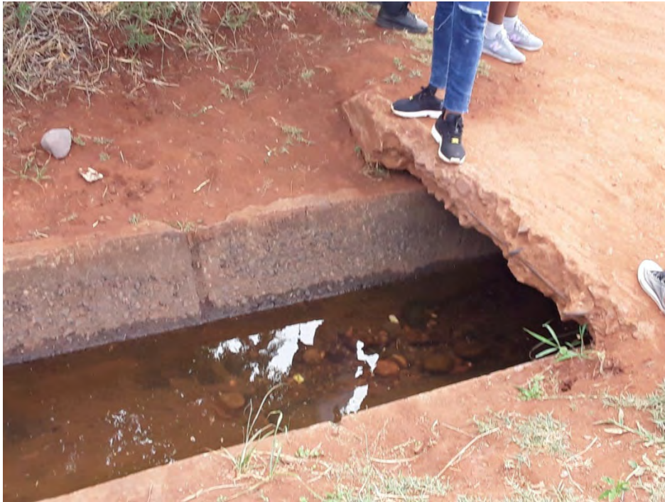
Figure 5.12: Small rocks at bottom of main canal at crossover bridge closer to entrance of Raliphaswa irrigation scheme
