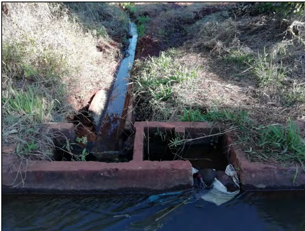
Figure 3.8: Typical offtake at Dzindi and main concrete furrow
