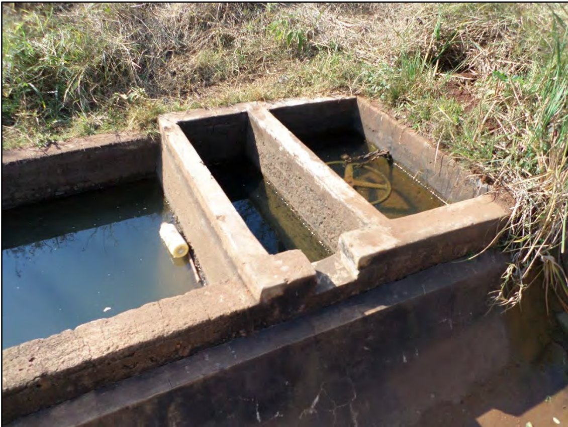
Figure 3.43: Mamuhohi night storage dam outlet valve
