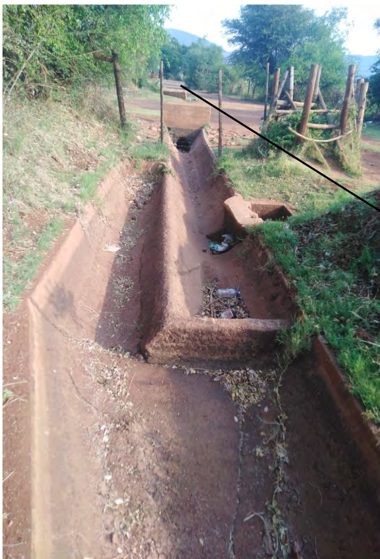
Figure 5.23: Deposition in canal at entrance of Mamuhohi irrigation scheme and collapsed structural member of crossover bridge to night storage dam
