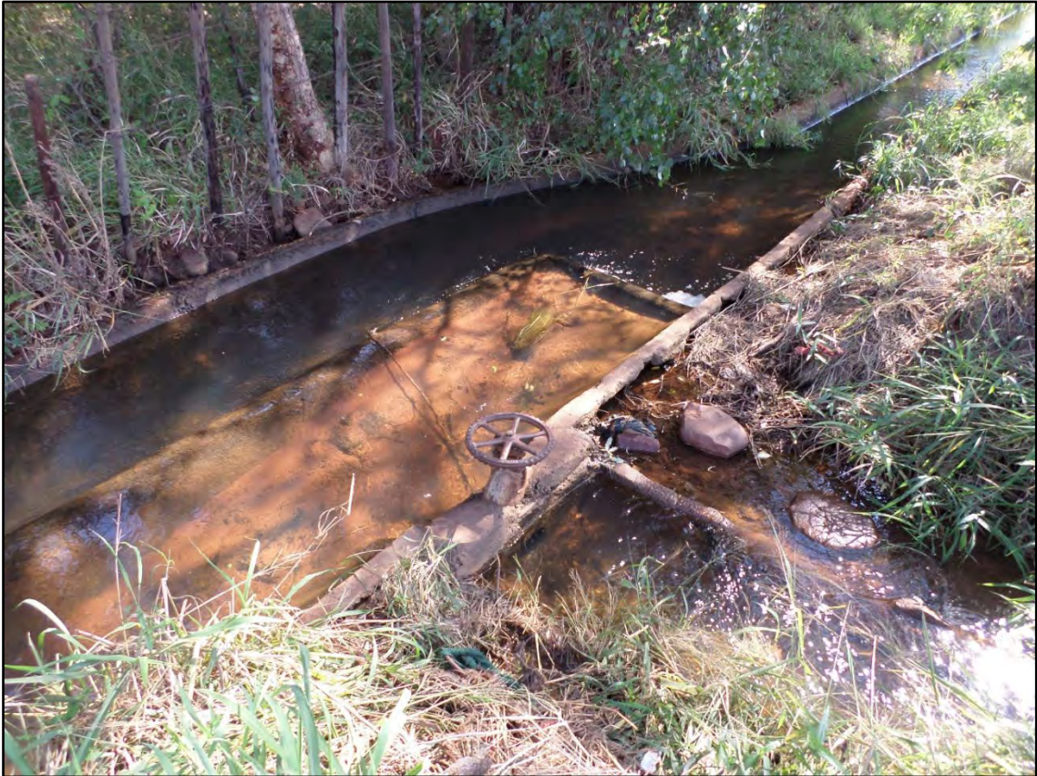
Figure 3.23: Silted long weir and offtake structure at Raliphaswa
