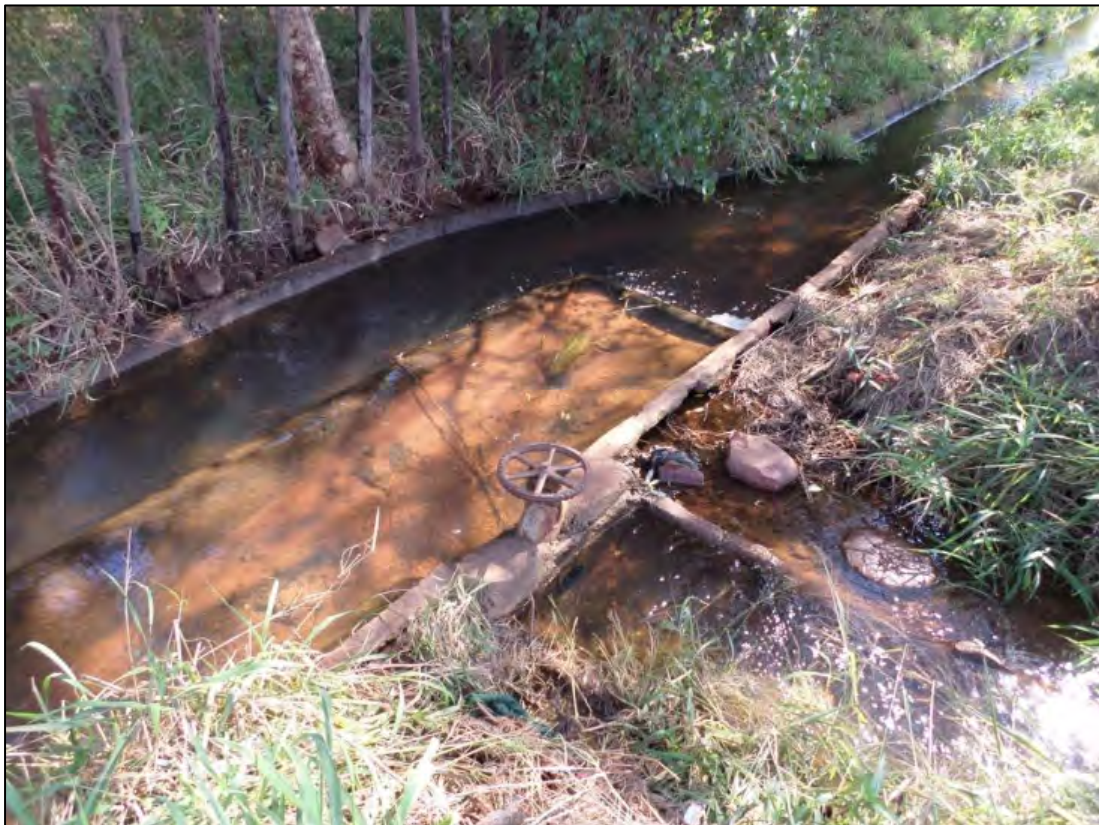
Figure 4.19 Typical long weir at Raliphaswa scheme with sediment accumulated at weir and erosion patterns around infrastructure
