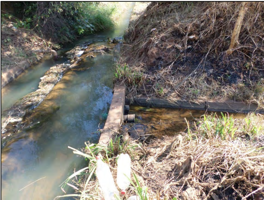
Figure 3.57: Typical orifice offtake at Rabali
