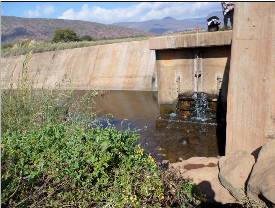
Figure 3.14: Leaking scour sluice gate at Raliphaswa
