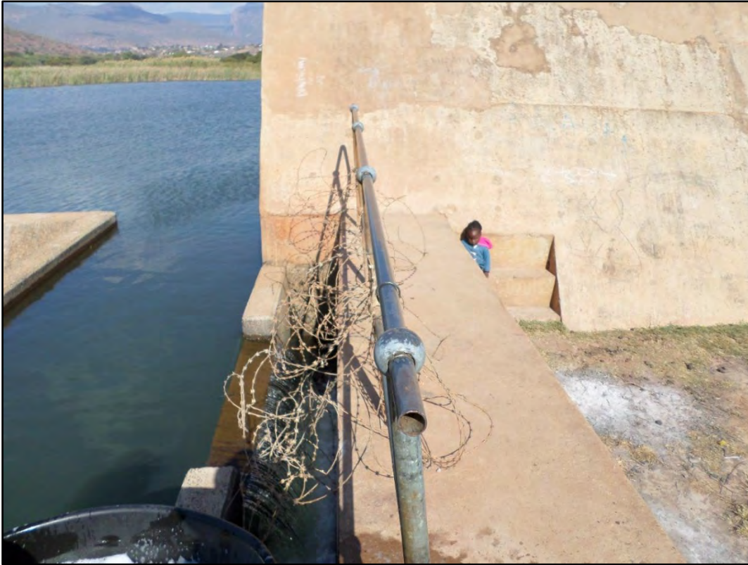
Figure 3.13: Intake into scour channel and overflow into intake chamber at Raliphaswa
