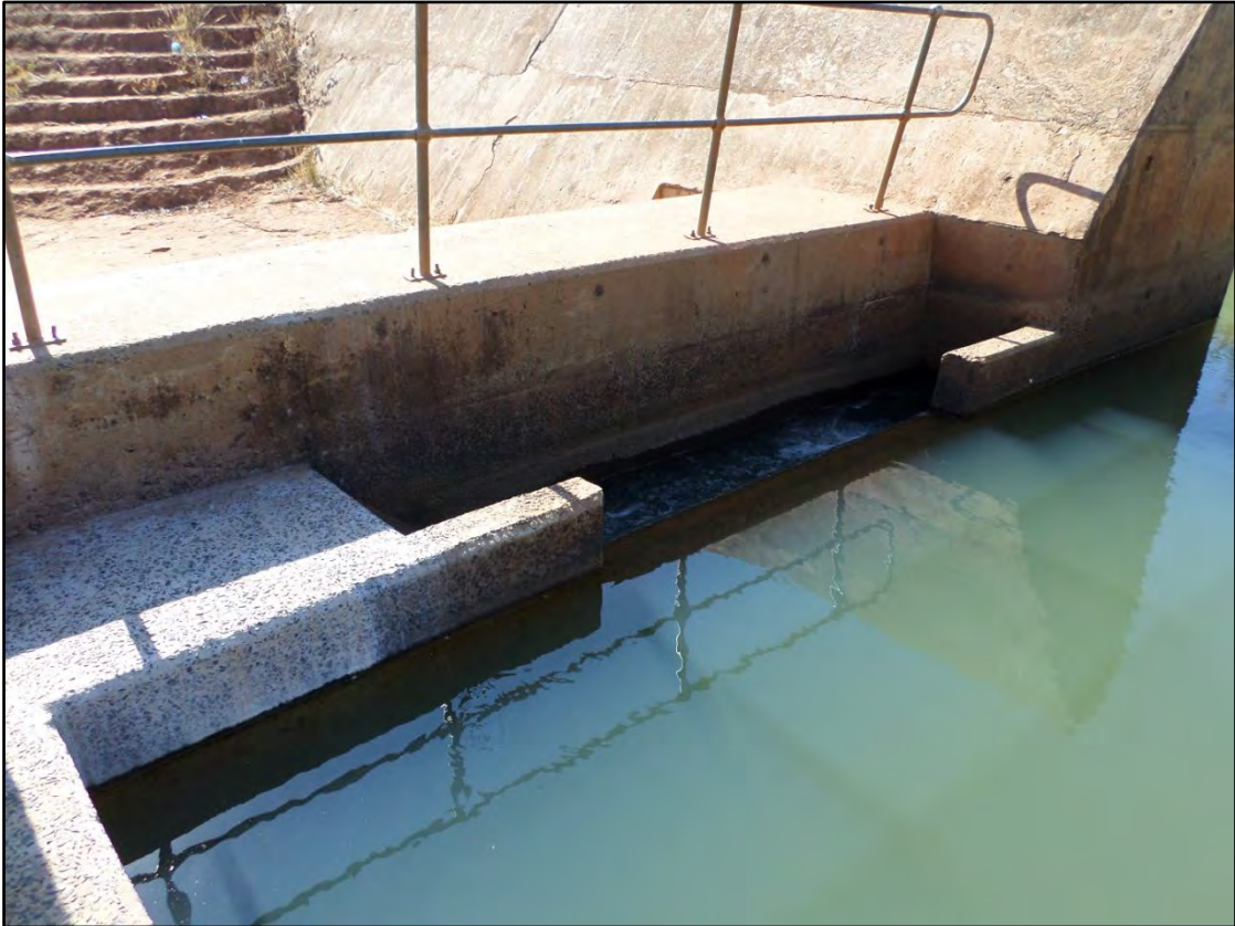
Figure 3.60: Overflow into intake chamber from scour channel at Mphephu
