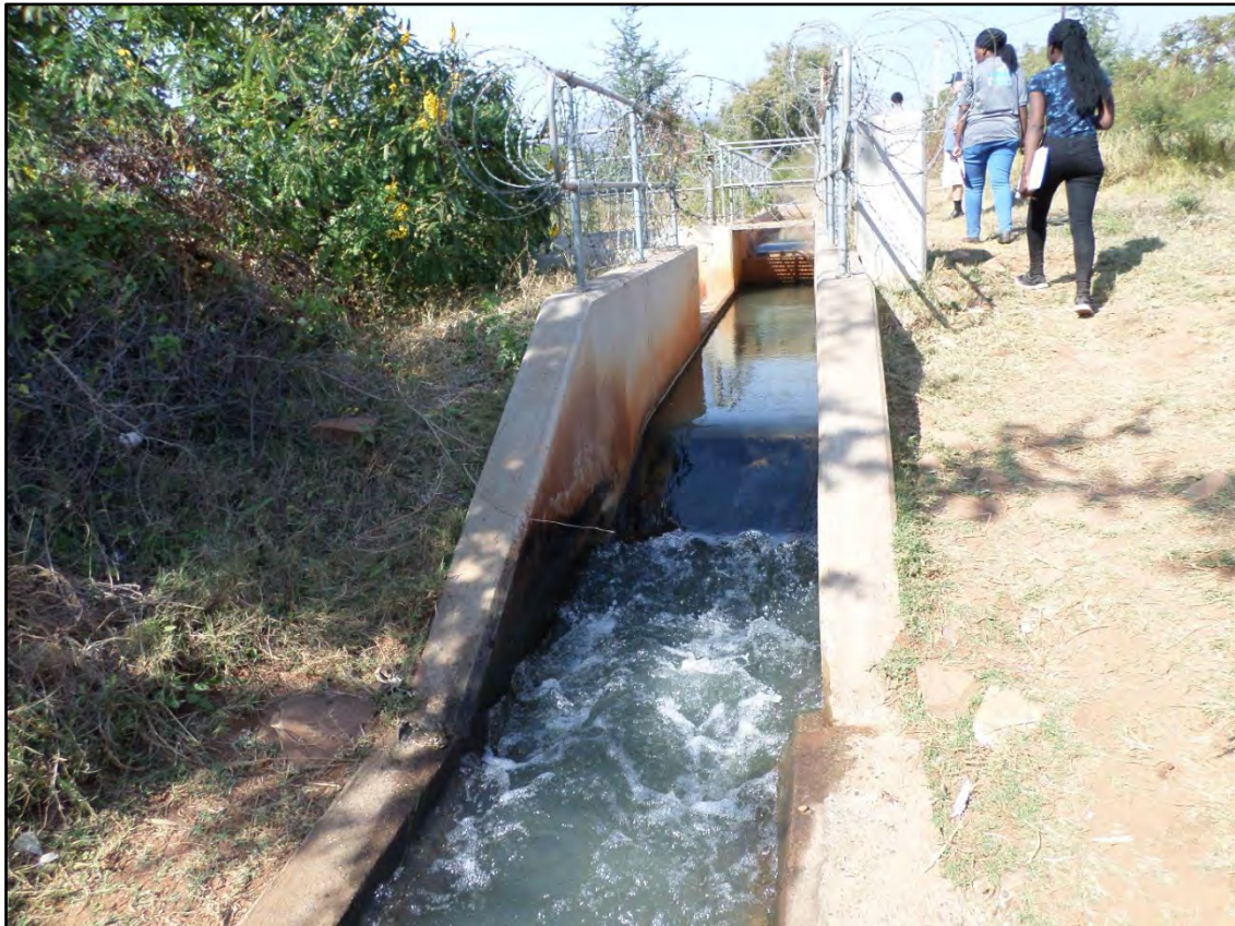
Figure 3.54: Reject and flow gauging structure at Rabali
