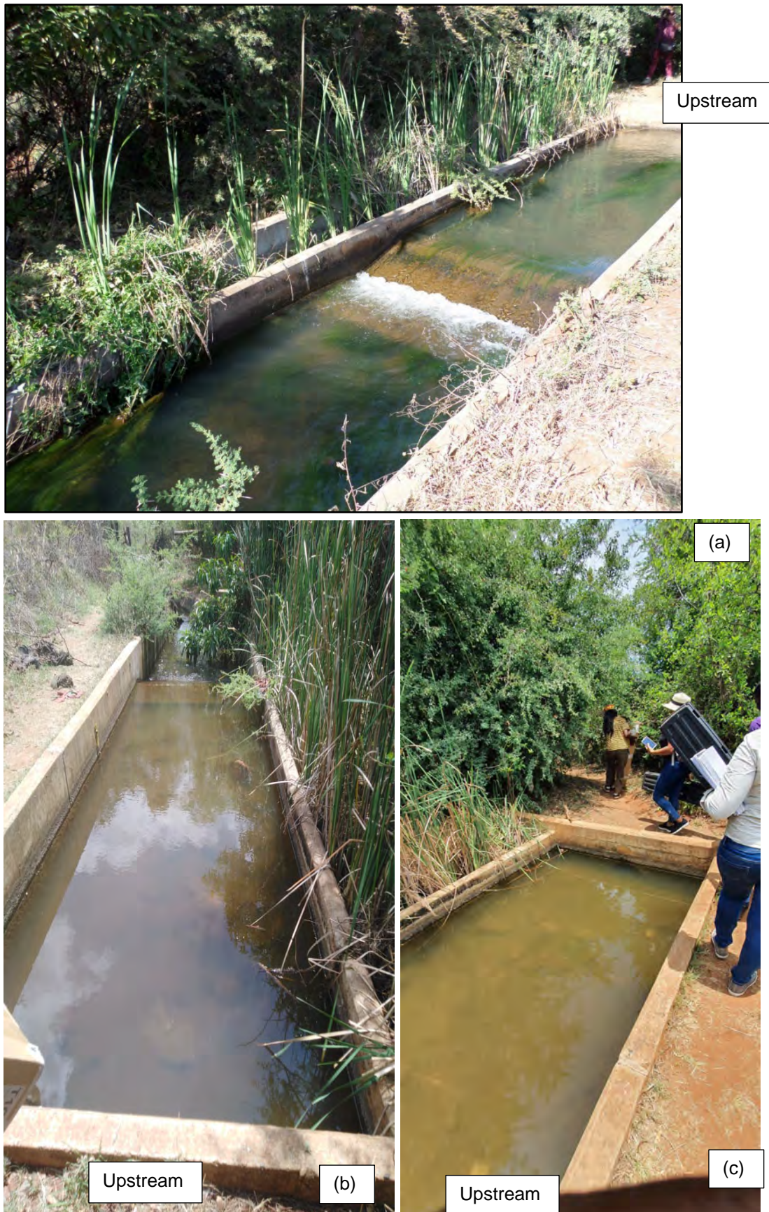
Figure 5.4: Intake pipe outlet and crump weir gauging structure on (a) 18 June 2019, (b) 02 November 2020 and (c) 19 November 2020
