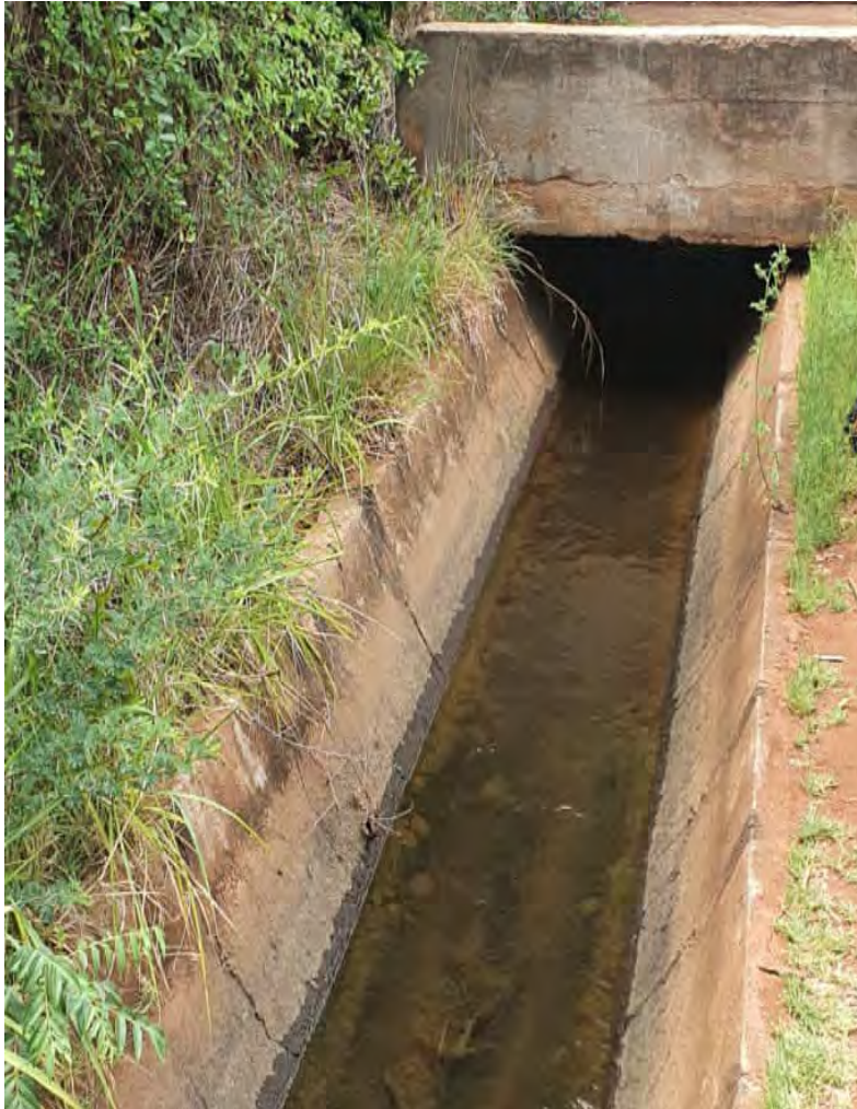
Figure 5.11: Main canal just after sluice gate with sediment deposits
