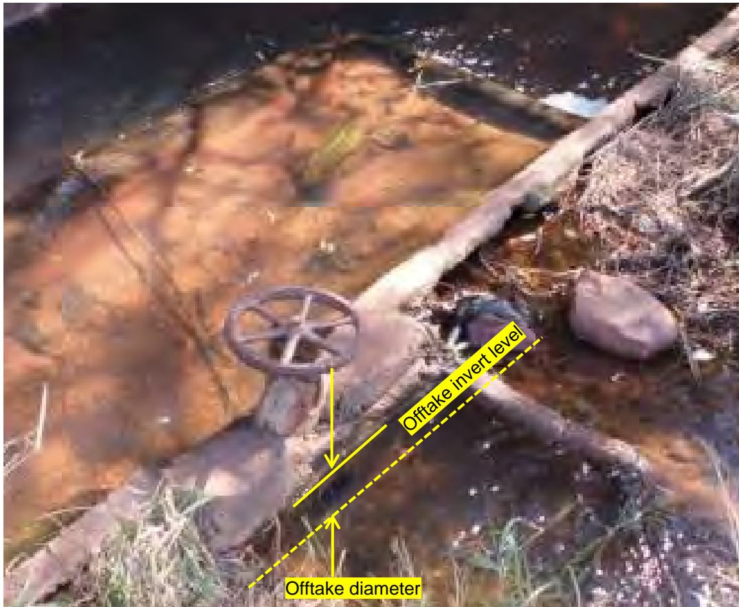
Figure 8.18 Hydraulic features of long weir and offtake structures
