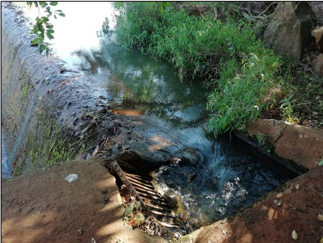
Figure 3.2: Downstream view of Dzindi river intake with trash screen
