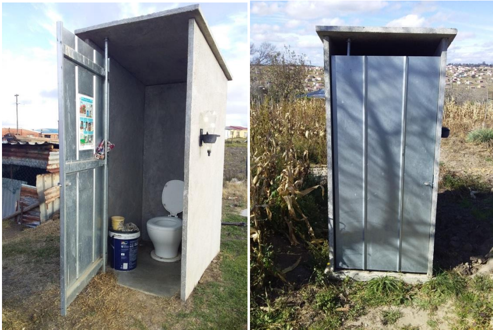
Figure 22: Typical pour flush construction in Jerseyvale
