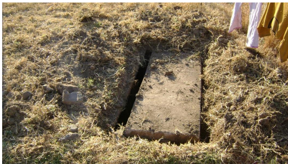
Figure E78: Excess soil and grass removed from pit cover slab for opening
