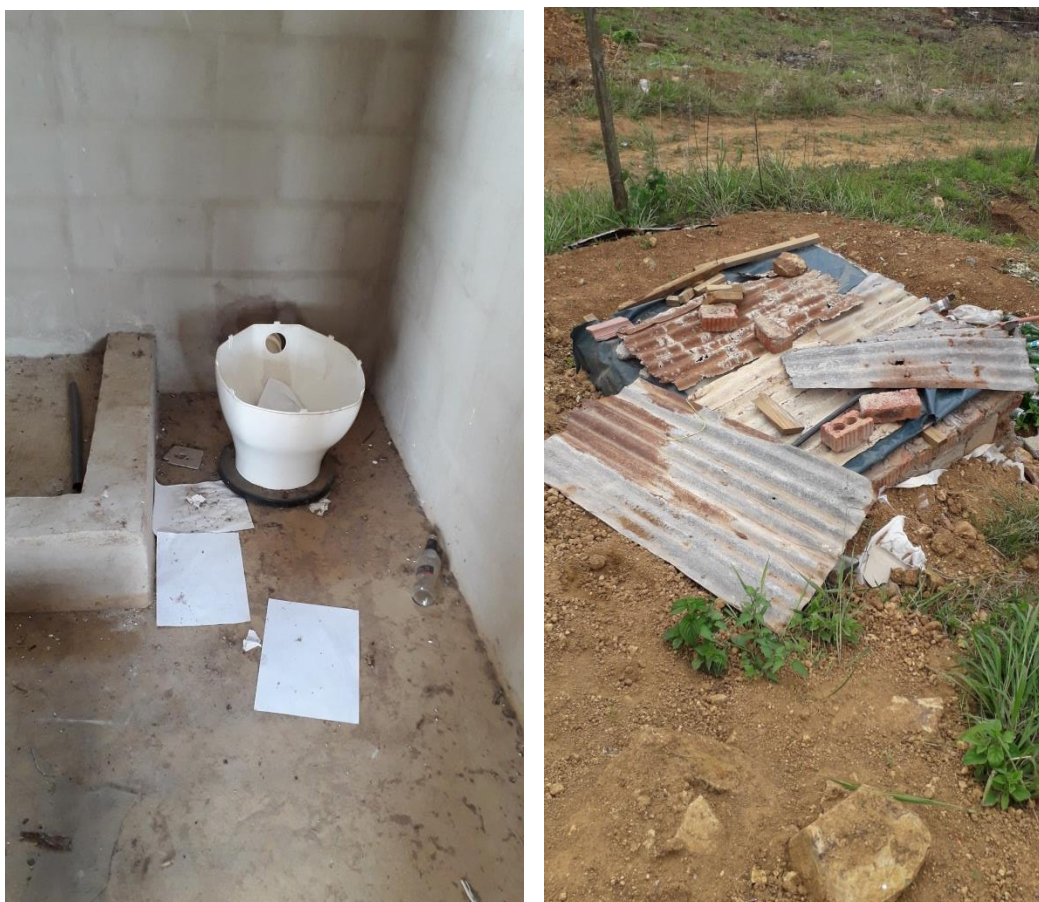
Figure K150: Unfinished construction as evidenced by improper pedestal (left) and home-built septic tank (right)
