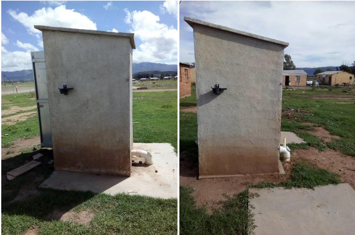
Figure 25: Single pit (left) and twin pit (right) pour flush units with pit cover slabs
