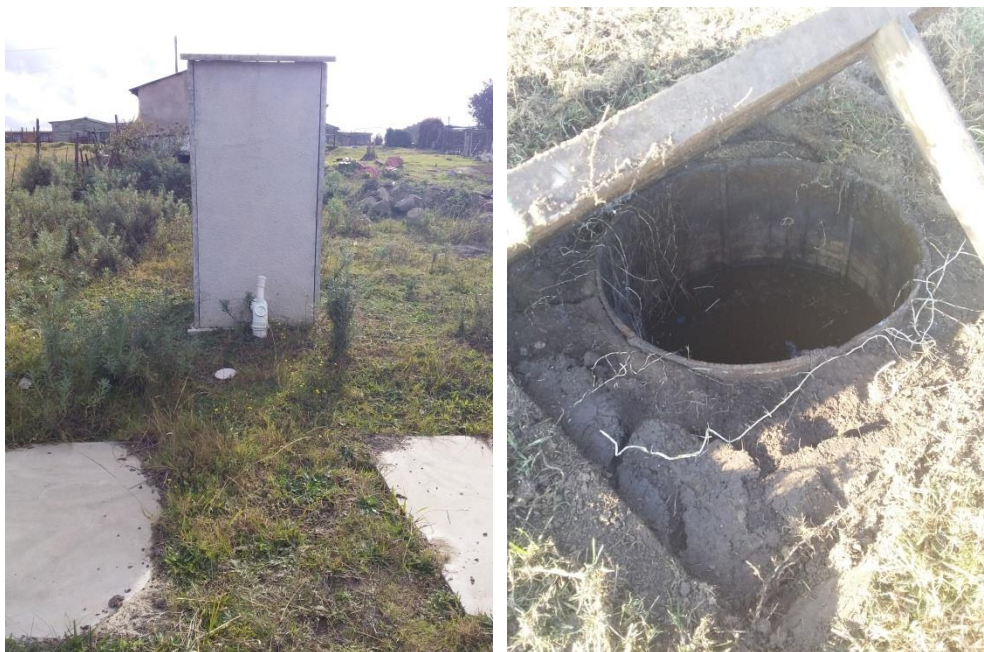
Figure F87: Typical leach pit design in Jerseyvale
