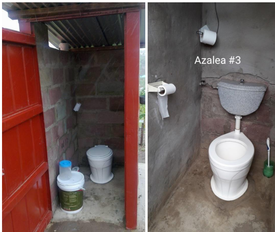
Figure 17: Unit in Azalea before (left) and after (right) upgrade to low flush unit
