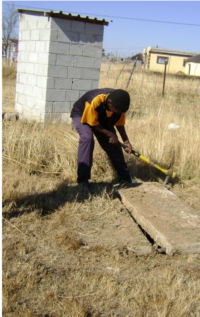
Figure E79: Worker removing pit cover slab for measurements
