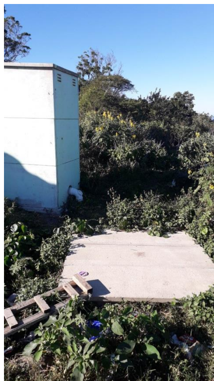
Figure N168: Single leach pit in Port St John's
