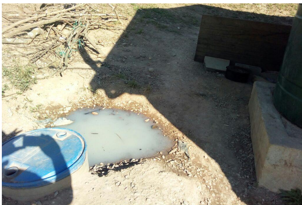
Figure K149: Example of greywater not properly draining and rather pooling on the surface
