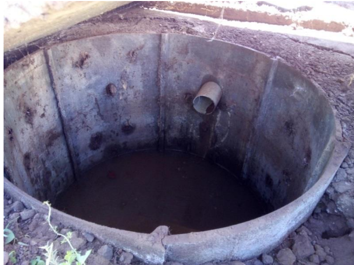
Figure G94: Typical leach pit design in Bongoletu
