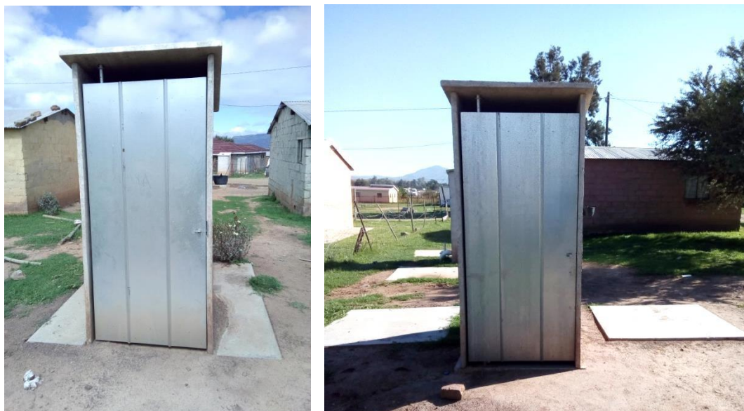
Figure G93: Single pit (left) and double pit (right) pour flush toilets in Bongolethu
