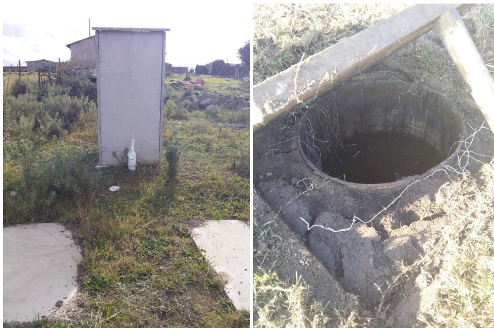
Figure 23: Typical leach pit design in Jerseyvale
