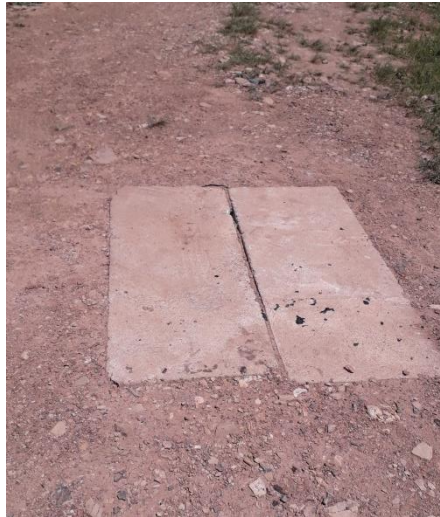
Figure K142: Offset pits and concrete covers
