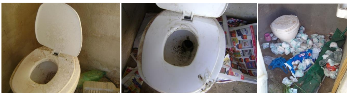
Figure H116: Pour flush toilets that are either no longer used or used but not properly maintained
