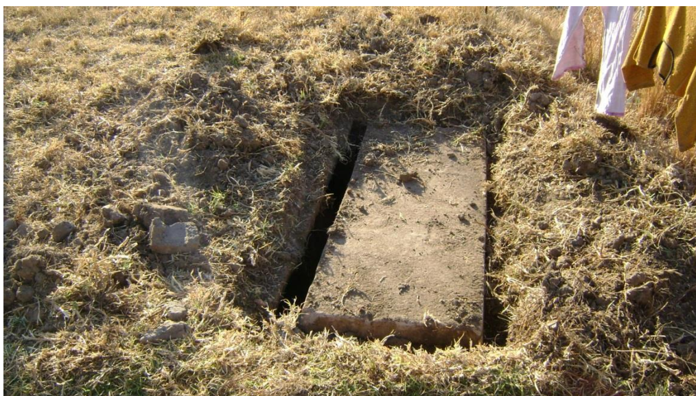
Figure 20: Excess soil and grass removed from pit cover slab for opening
