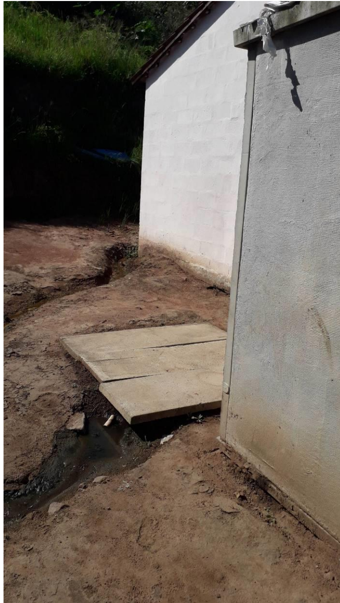
Figure 35: Pit cover slabs and a leak from the pit
