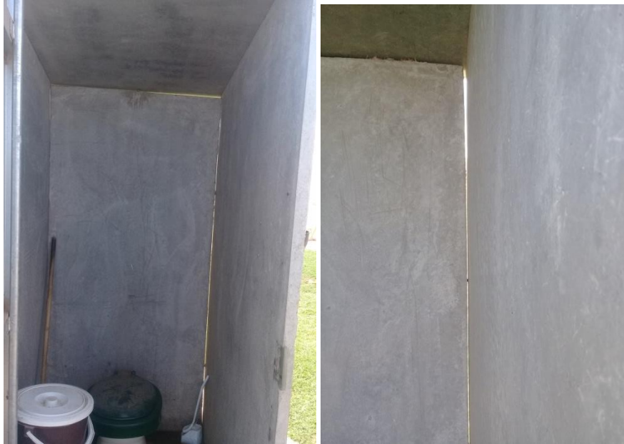
Figure G99: Pour flush toilet structures with joints that were not sealed
