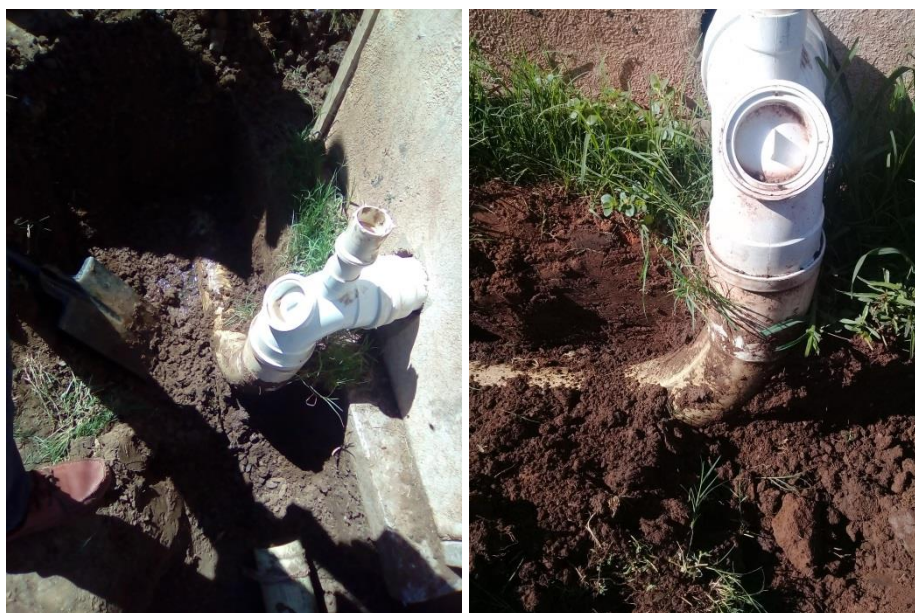
Figure 67: Pipework switching option using an elbow
