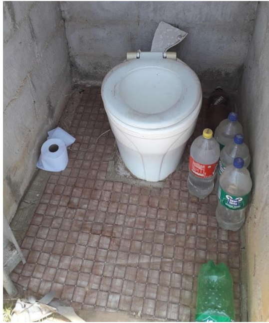
Figure D68: Pour flush unit in Msunduzi with water stored in 2-litre bottles
