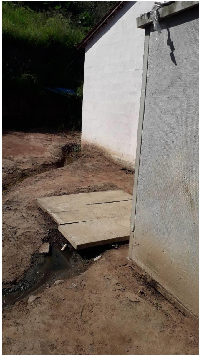
Figure J133: Pit cover slabs and a leak from the pit
