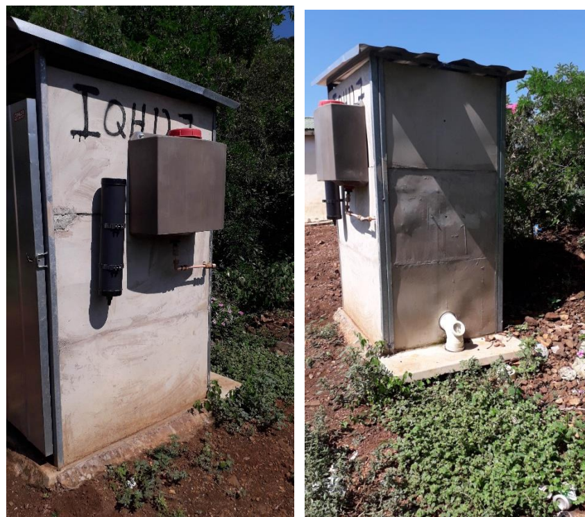
Figure 66: Pour flush toilet with 50 litre tank installed on the outside and connected to a cistern inside the toilet, located in Maphumulo, Ilembe DM
