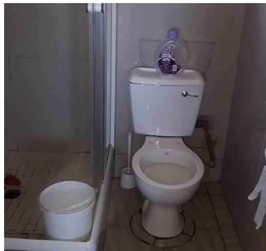
Figure K141: New pedestal and cistern installed at Oakford (full flush)
