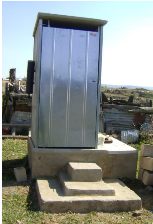
Figure H115: Newly constructed VIP toilet (note elevated structure due to high groundwater table)
