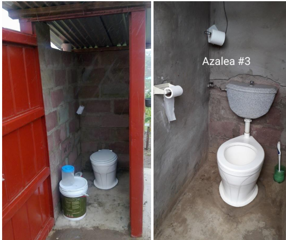
Figure D70: Unit in Azalea before (left) and after (right) upgrade to low flush unit
