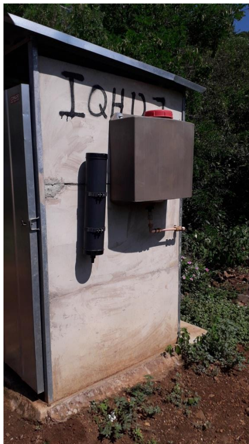
Figure L155: Pour flush toilet with large water storage tank installed outside toilet structure, connected to the cistern
