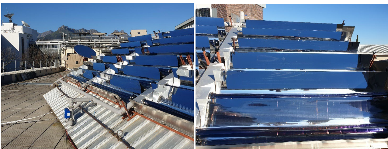
Figure 3.10. Photographs of the low-cost solar concentration parabolic through system developed by the Solar Thermal Energy Research Group, at the University of Stellenbosch
